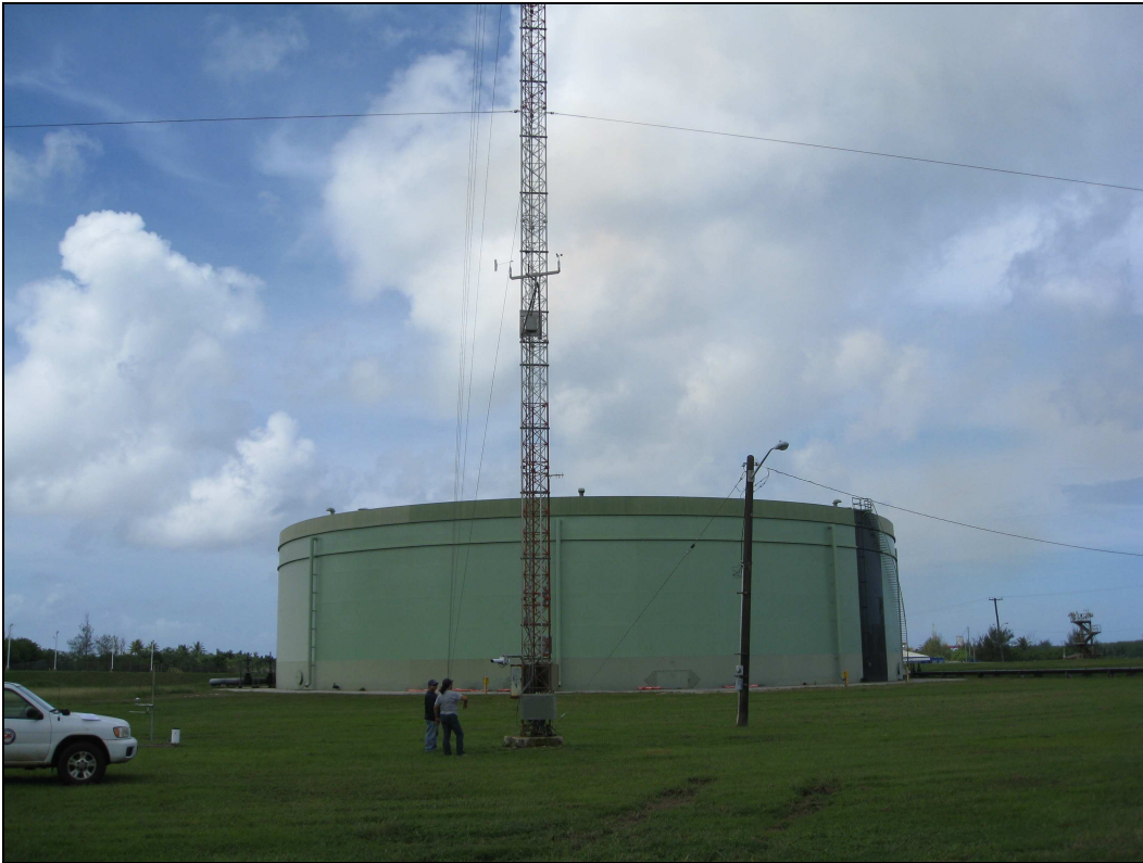
Figure 8. GPA 60-m met tower at Cabras-Piti Power Plant
