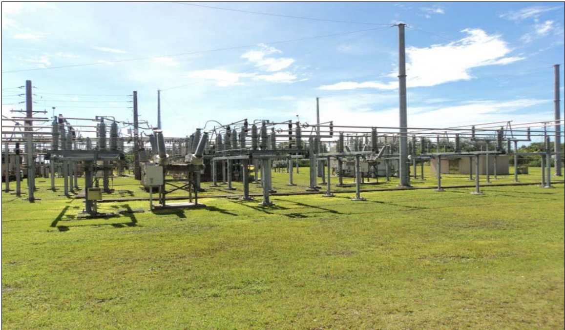
Eastern End Looking West - Existing Substation
