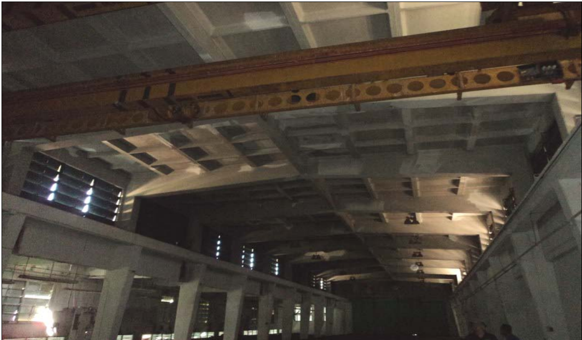
Agana Power Plant - Western End Looking East
