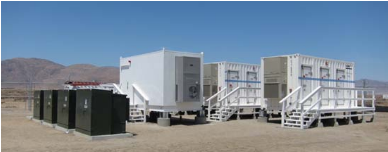
Figure 5-8 Small Scale Container Installation (Lithium-Ion)
