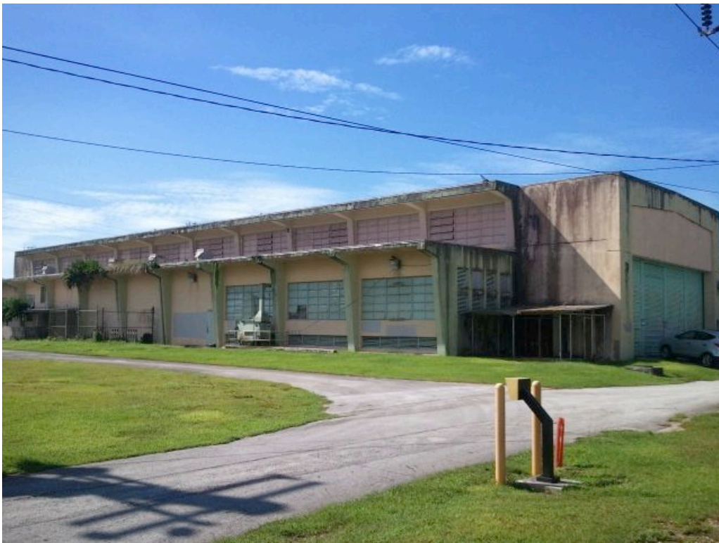
Photo B Exterior view of Agana Power Plant facing north/northwest
