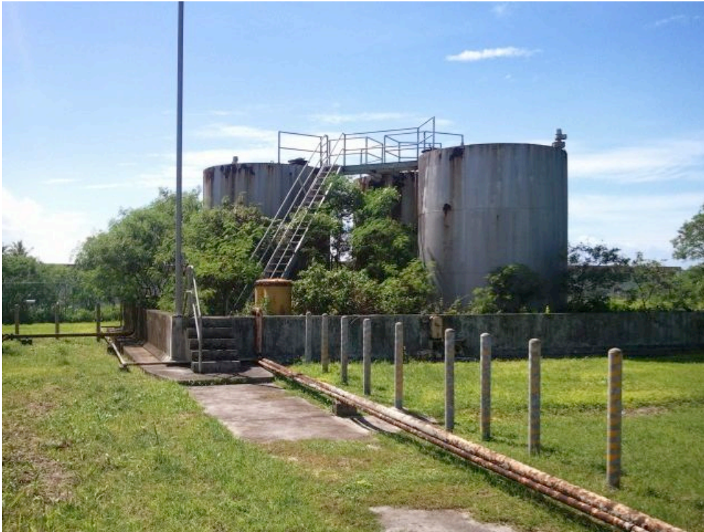
Photo I View of ASTs present at Agana Power Plant
