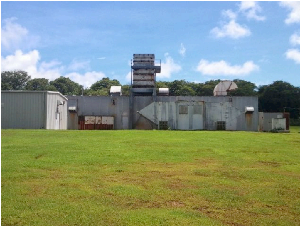
Photo N View of MARBO Power Plant facing south
