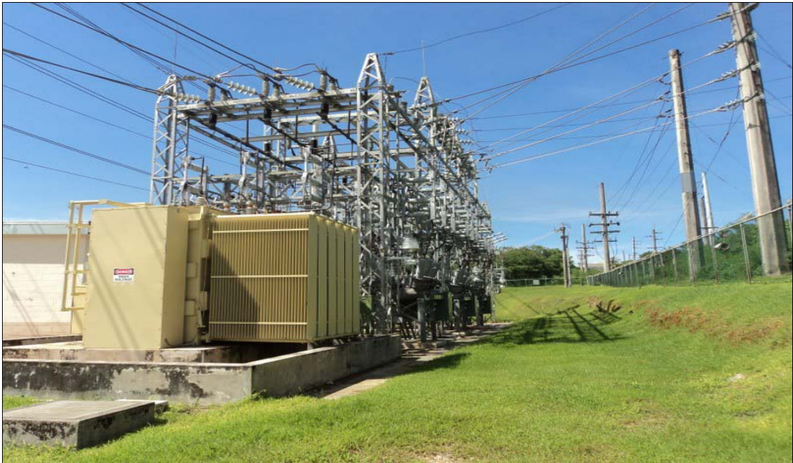
34-5 kV Substation East of Building
