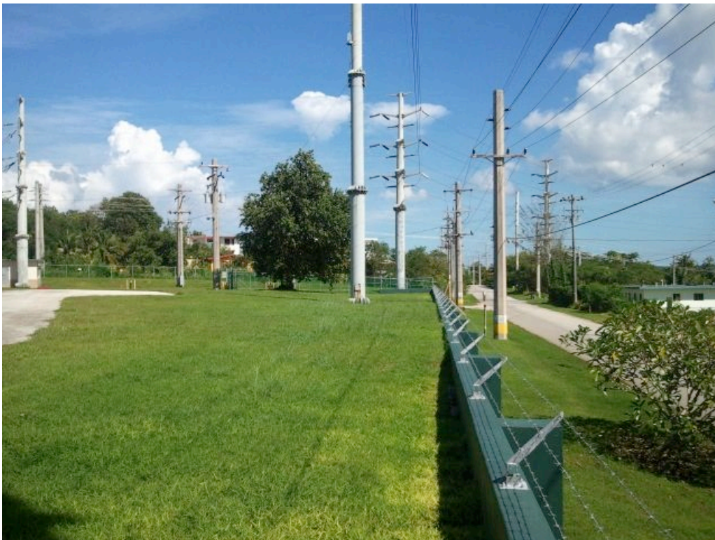
Photo L View of fence line running north at Agana Power Plant
