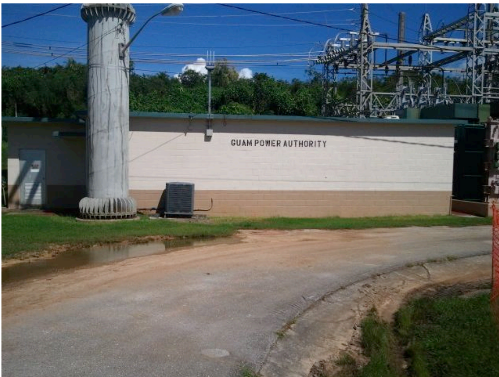
Photo D View of first substation building at Agana Power Plant
