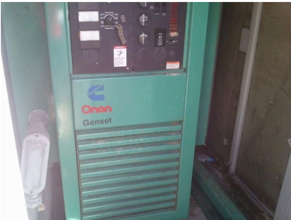
Photo V View of small generator at MARBO Power Plant
