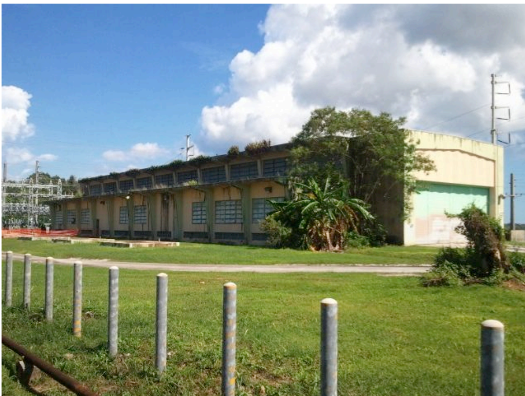
Photo J View of AST Agana Power Plant looking southeast
