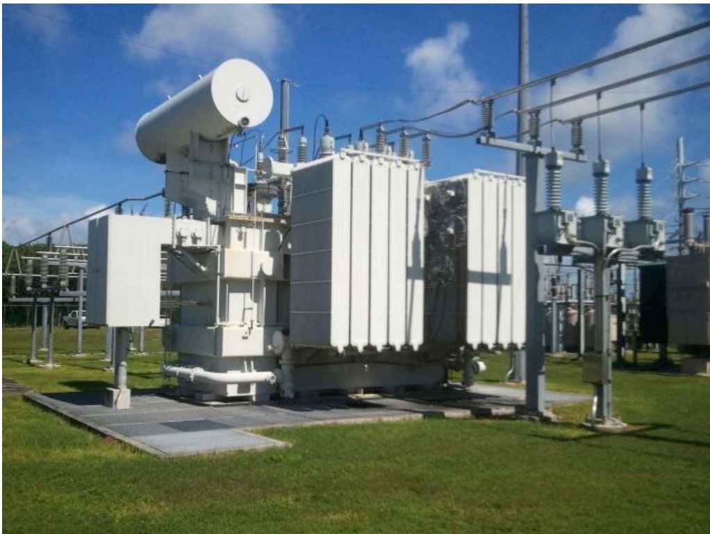
Photo BB View of transformer at Harmon Substation
