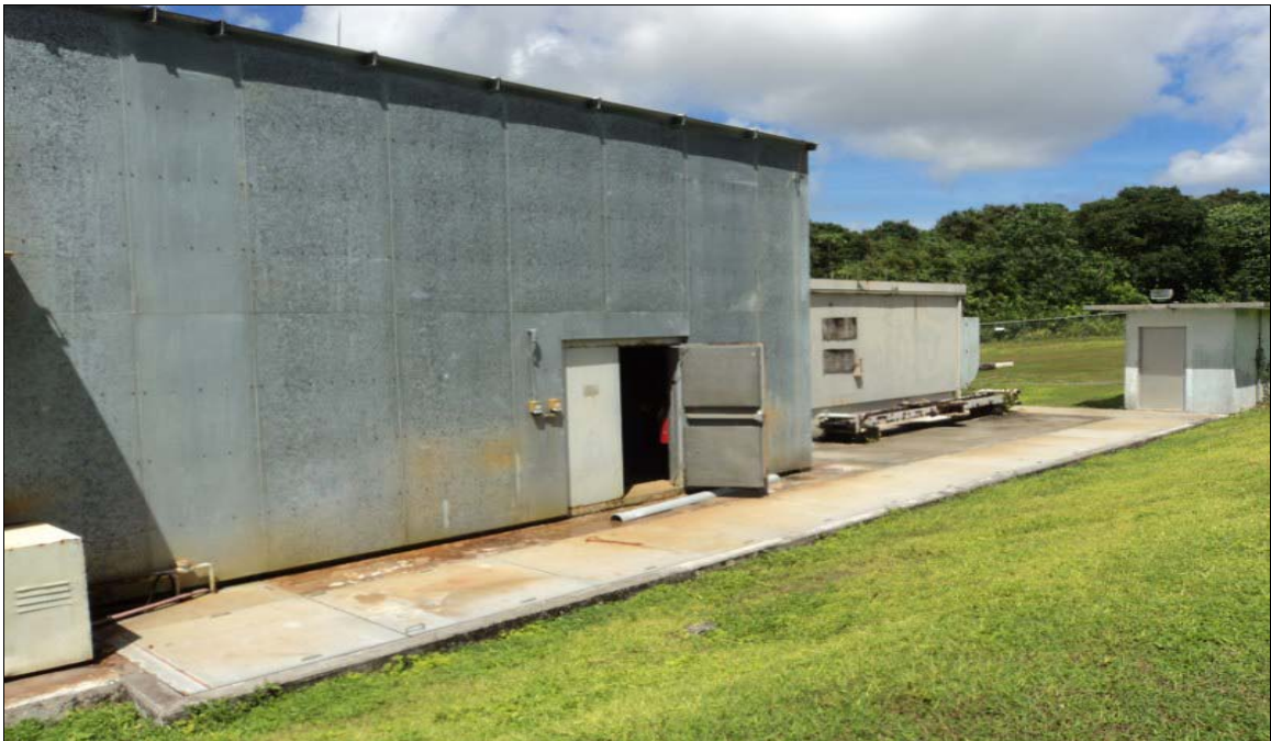
Southern End of Structure
