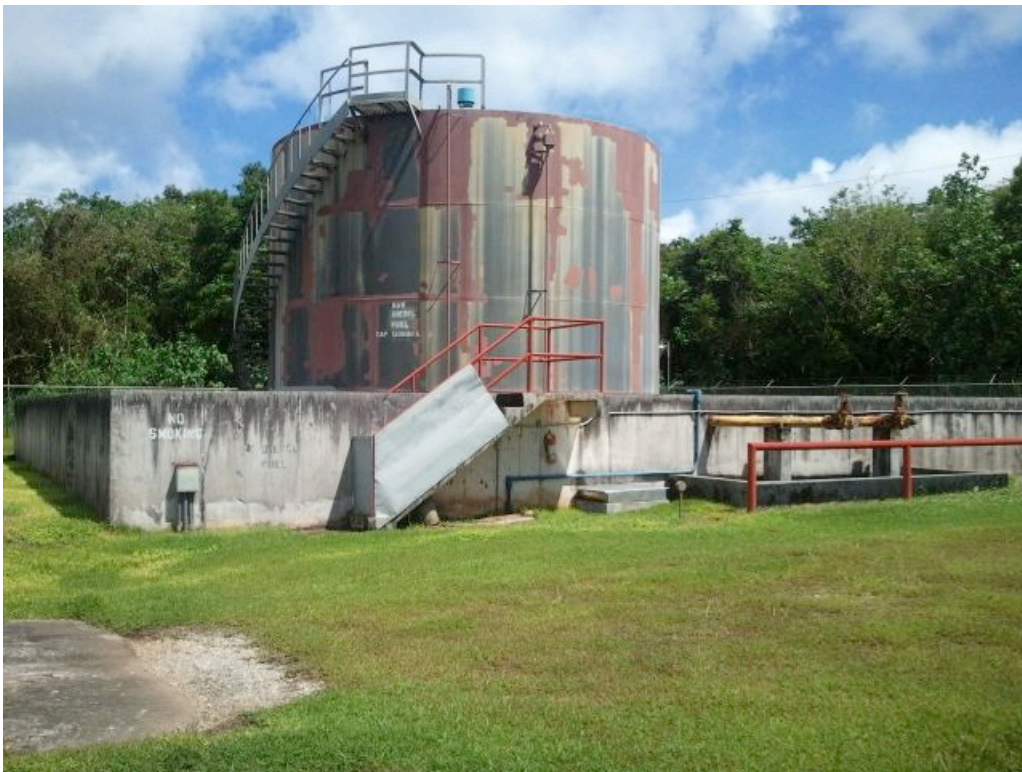
Photo T View of AST at MARBO Power Plant
