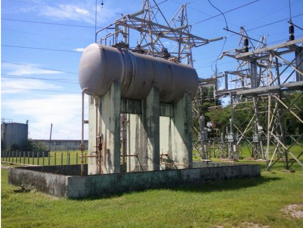
Photo G View of AST present at Agana Power Plant
