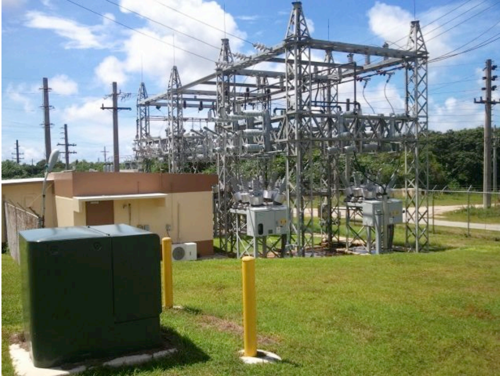
Photo O View of substation at MARBO Power Plant
