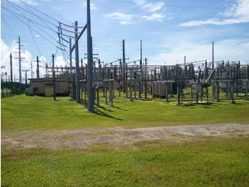
Photo Y View of Harmon Substation facing west
