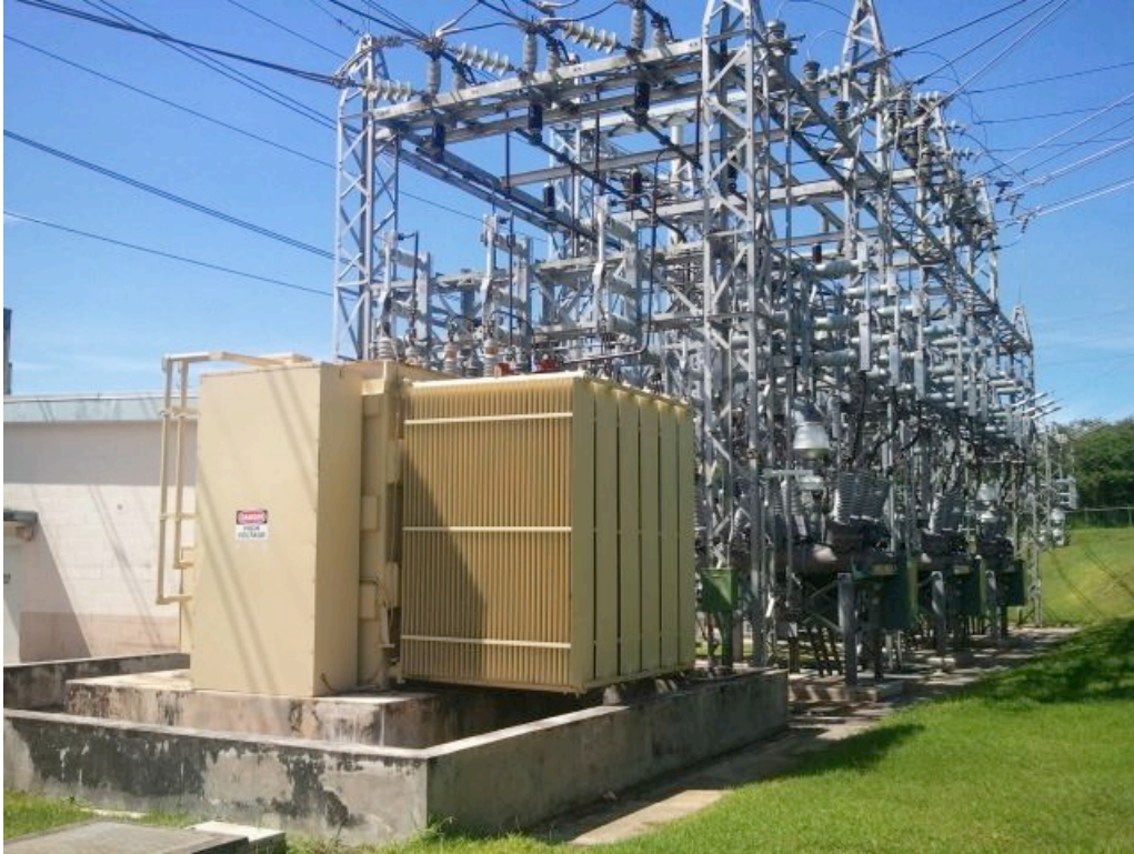
Photo C View of electrical equipment present at Agana Power Plant
