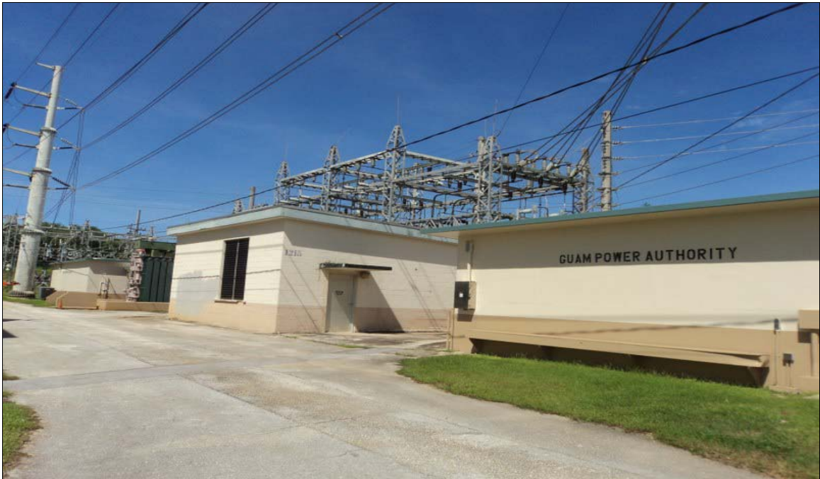
Existing Substation East of Building
