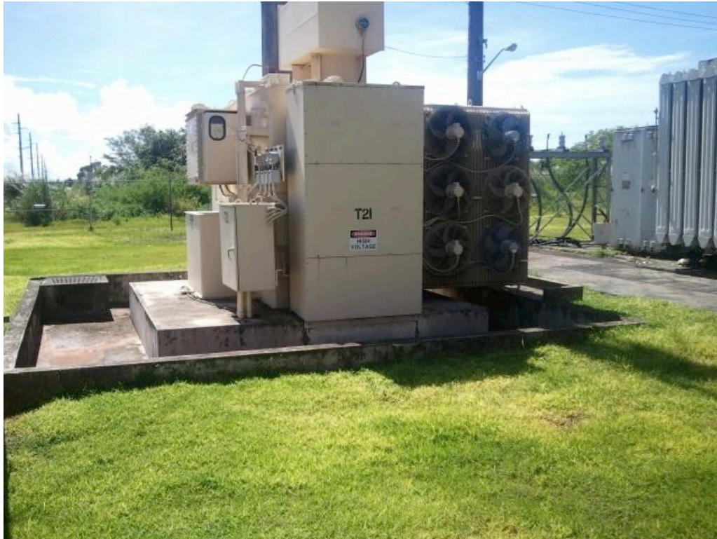
Photo EE View of transformer at Harmon Substation
