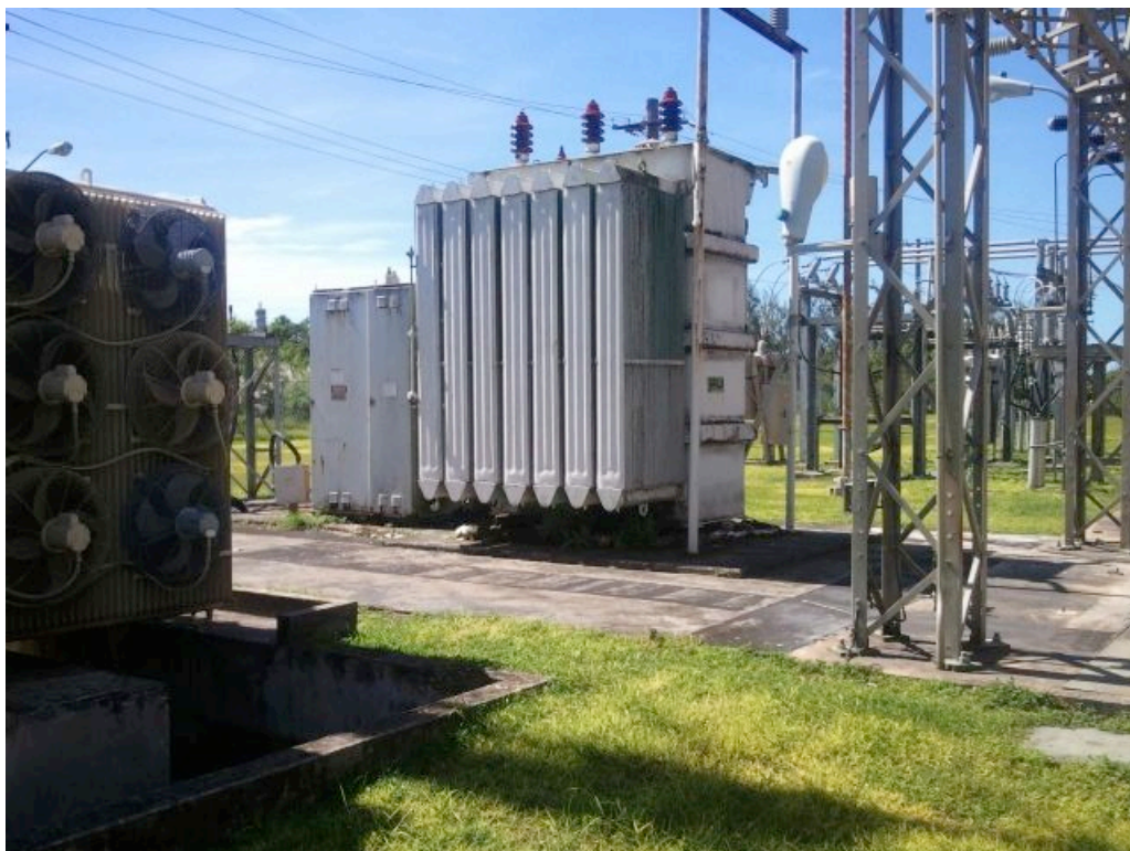
Photo FF View of transformer at Harmon Substation
