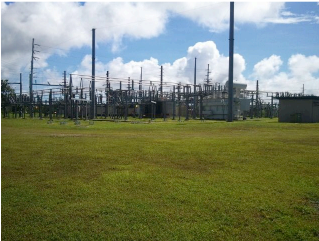
Photo Z View of Harmon Substation facing south
