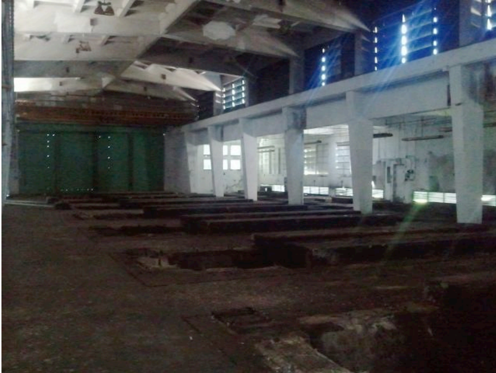
Photo A Interior view of Agana Power Plant
