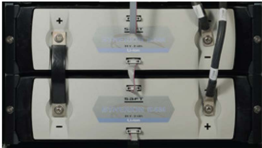
Figure 5-2 Example Lithium-Ion Battery (Saft)
