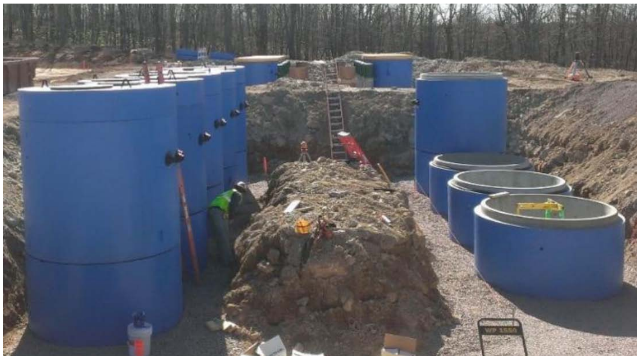
Figure 5-9 Below Ground Flywheel Installation
