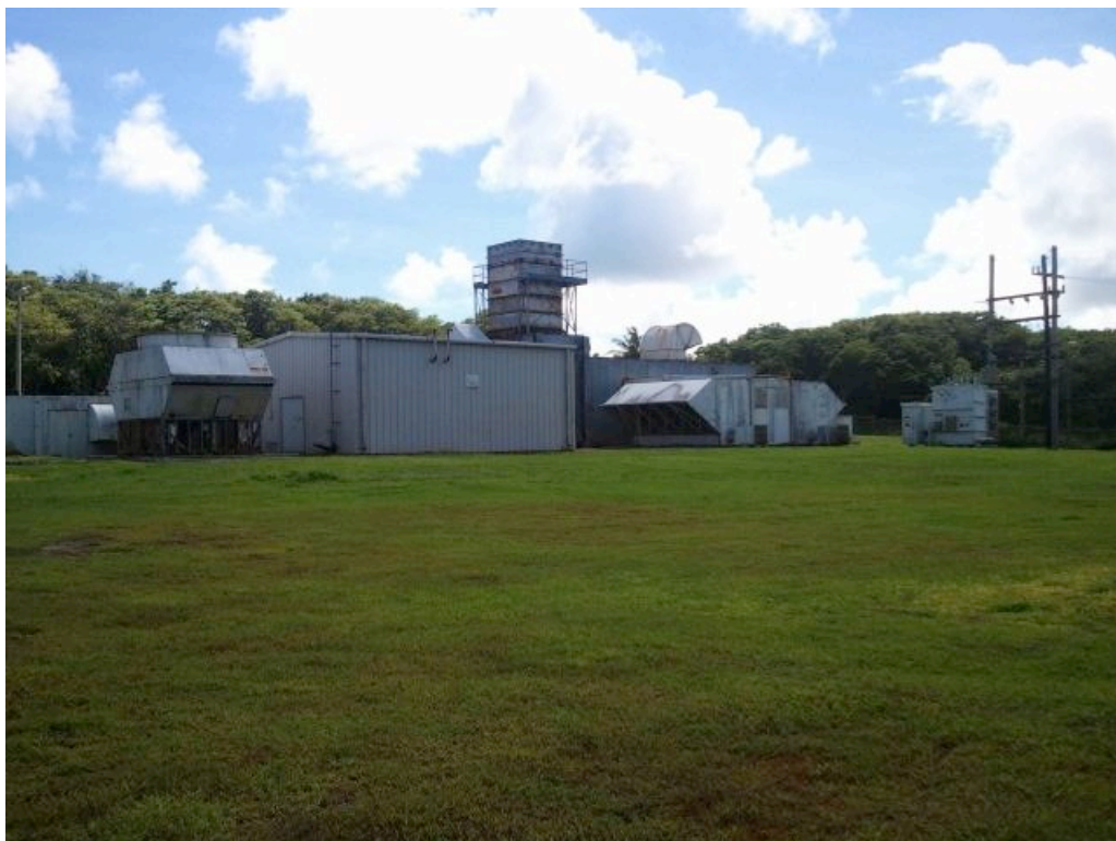
Photo X View of MARBO Power Plant facing southwest
