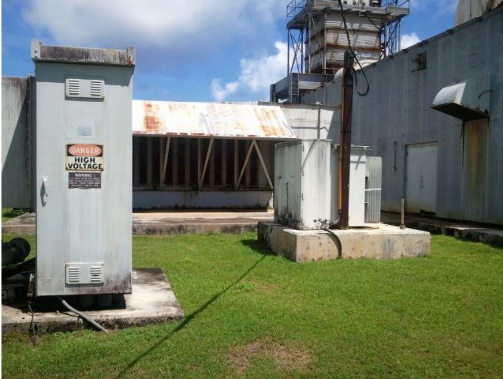
Photo Q View of second transformer at MARBO Power Plant
