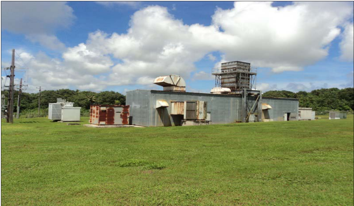
Southern End Looking North
