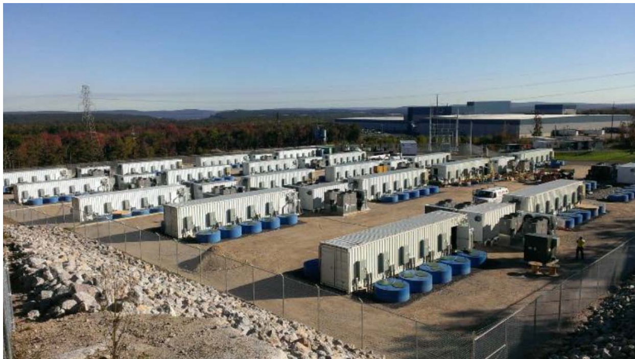
Figure 5-10 Example Final Site Installation
