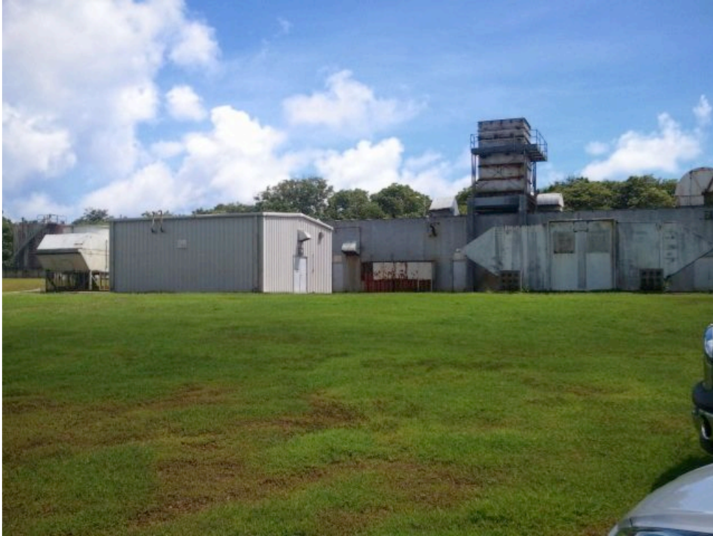
Photo M View of MARBO Power Plant facing south
