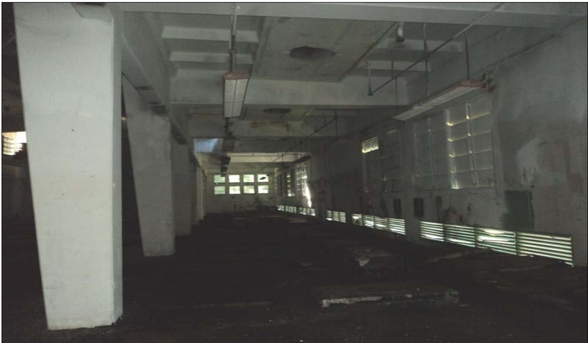
Agana Power Plant - Northern Portion Looking West
