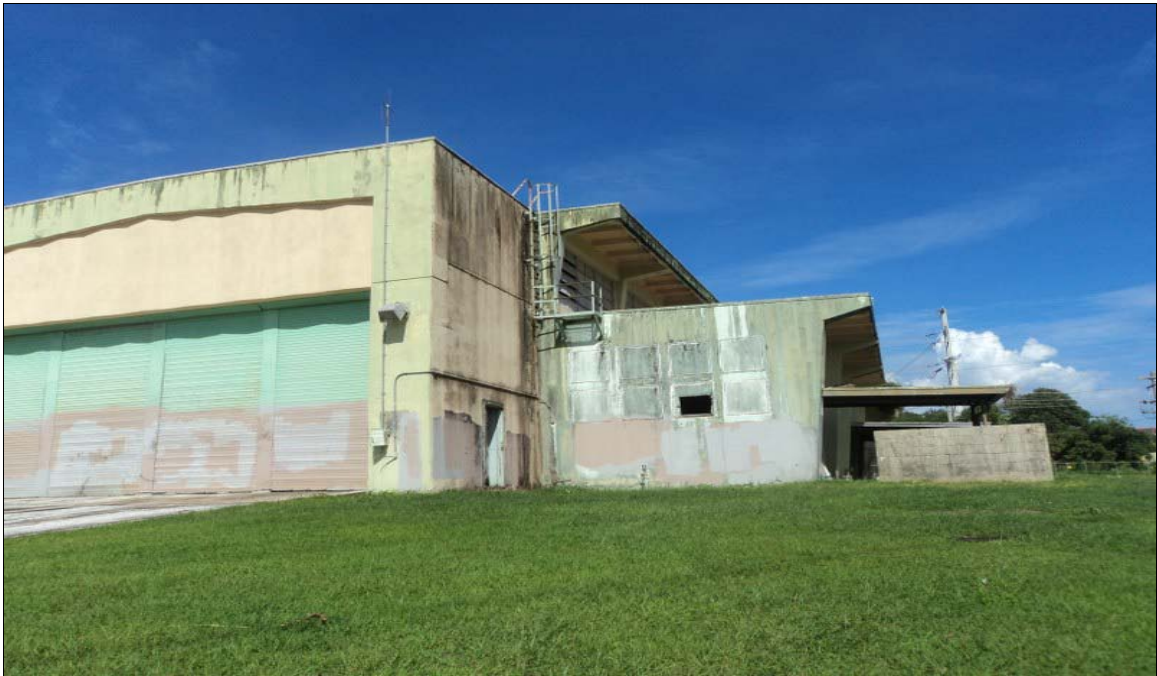
Western End of Building - Outside
