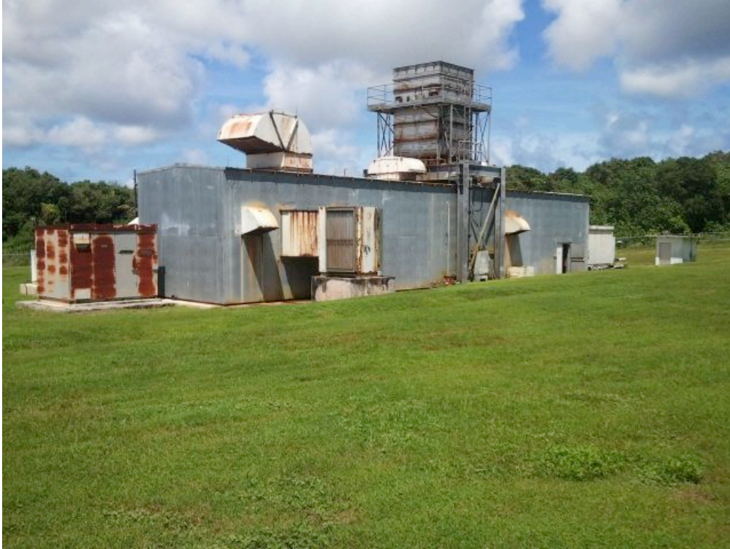
Photo S View of MARBO Power Plant facing north/northeast
