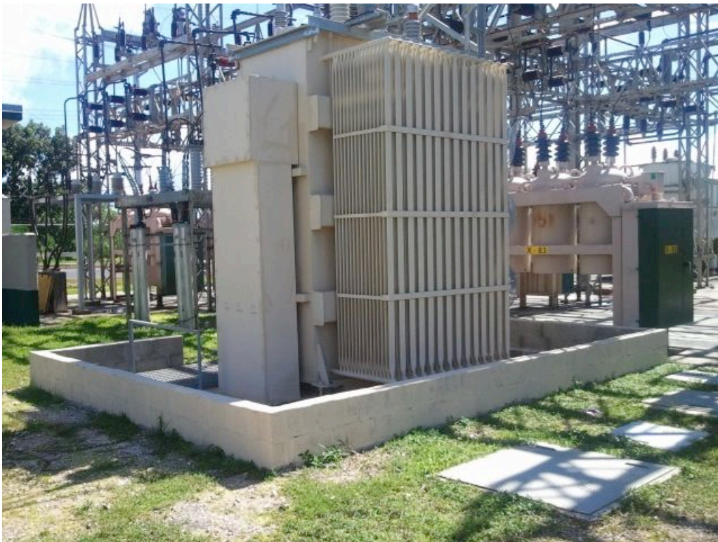
Photo DD View of transformer at Harmon Substation
