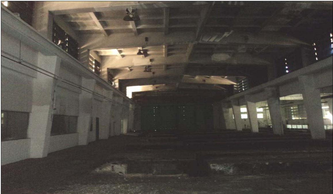
Agana Power Plant - Eastern End Looking West
