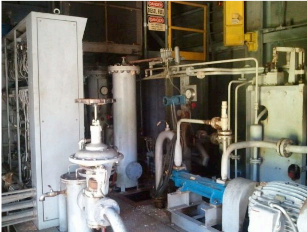
Photo W View of interior of MARBO Power Plant
