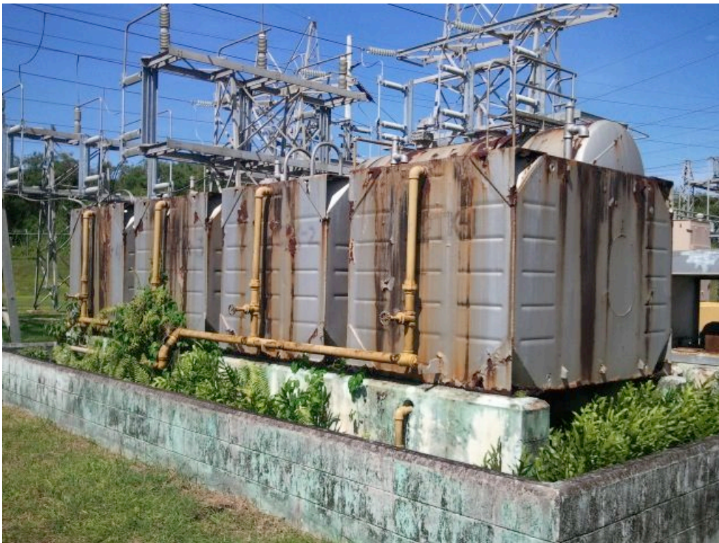
Photo H View of AST present at Agana Power Plant
