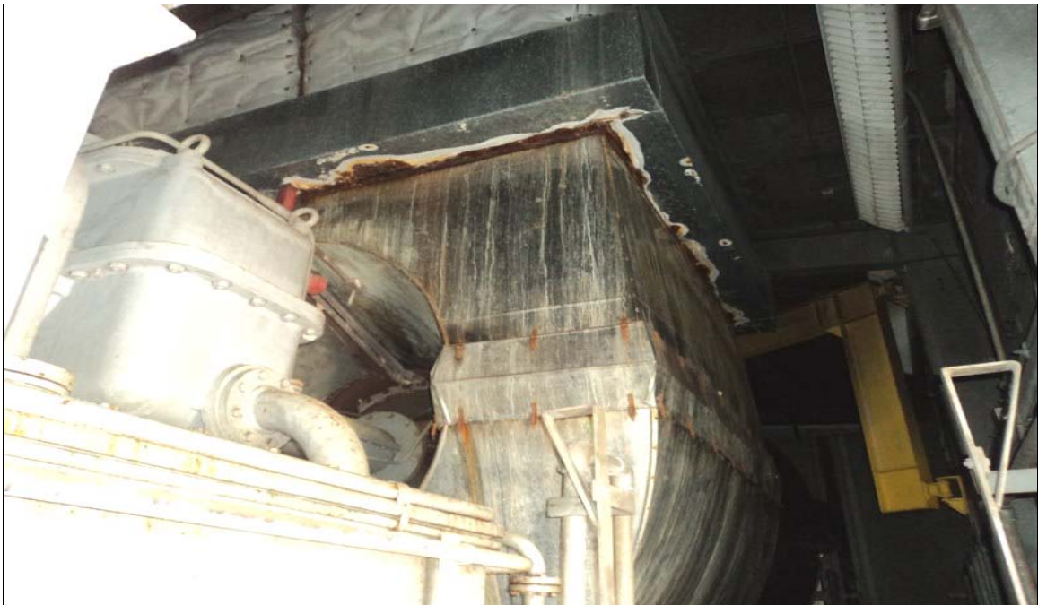
Interior Southern Building
