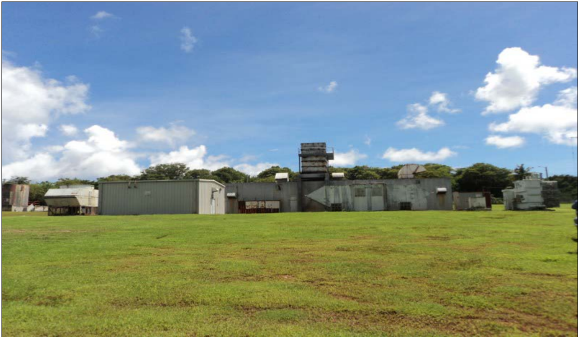
Northern End Looking South
