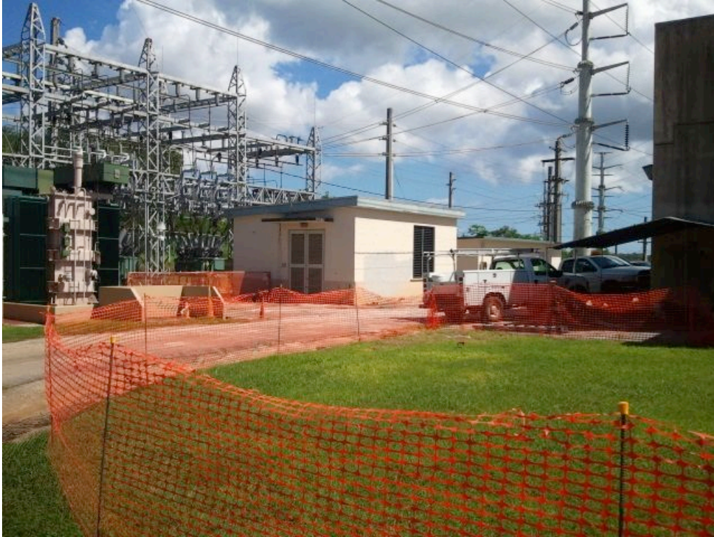
Photo E View of second substation building at Agana Power Plant
