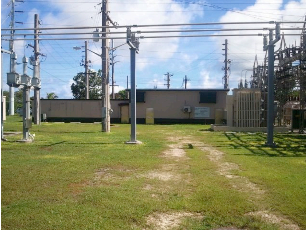
Photo CC View of Harmon Substation control building facing southeast
