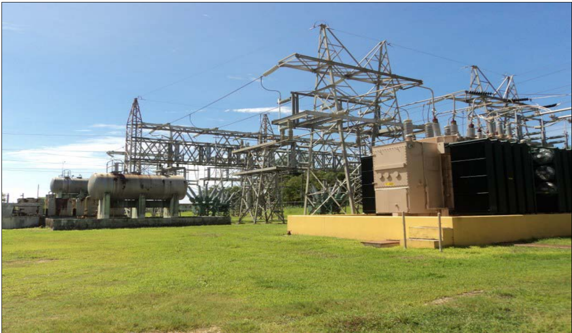
115kV Substation and Existing Fuel Tanks
