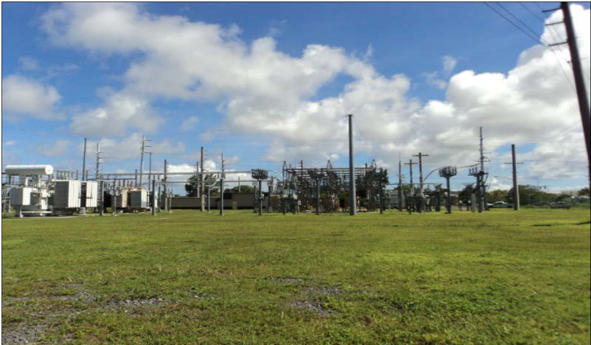
Northern End Looking South - Existing Substation
