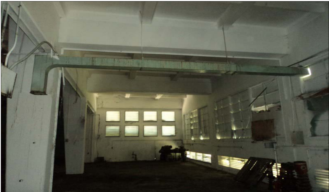
Agana Power Plant - Southern Portion Looking East
