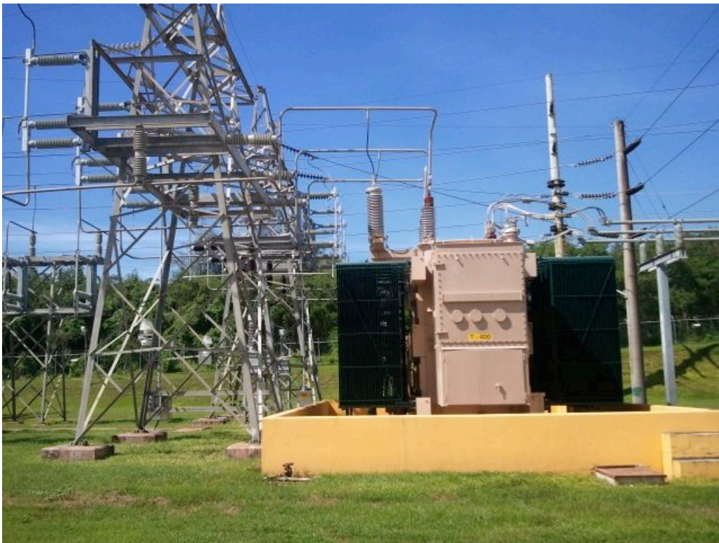
Photo F View of electrical equipment present at Agana Power Plant
