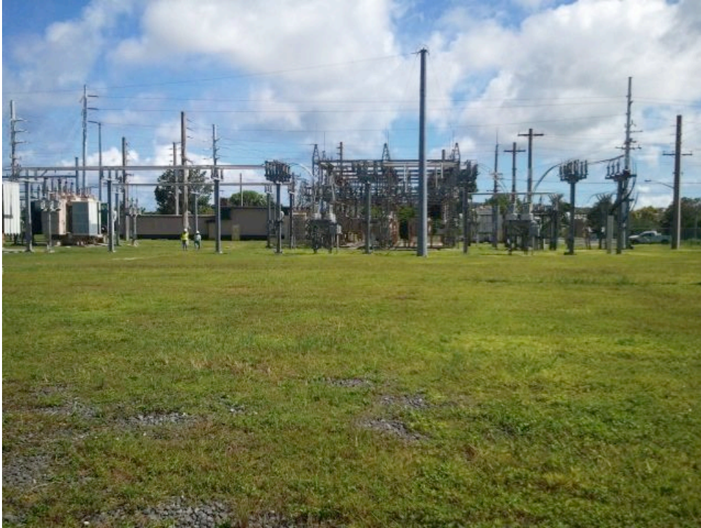
Photo AA View of Harmon Substation facing southeast
