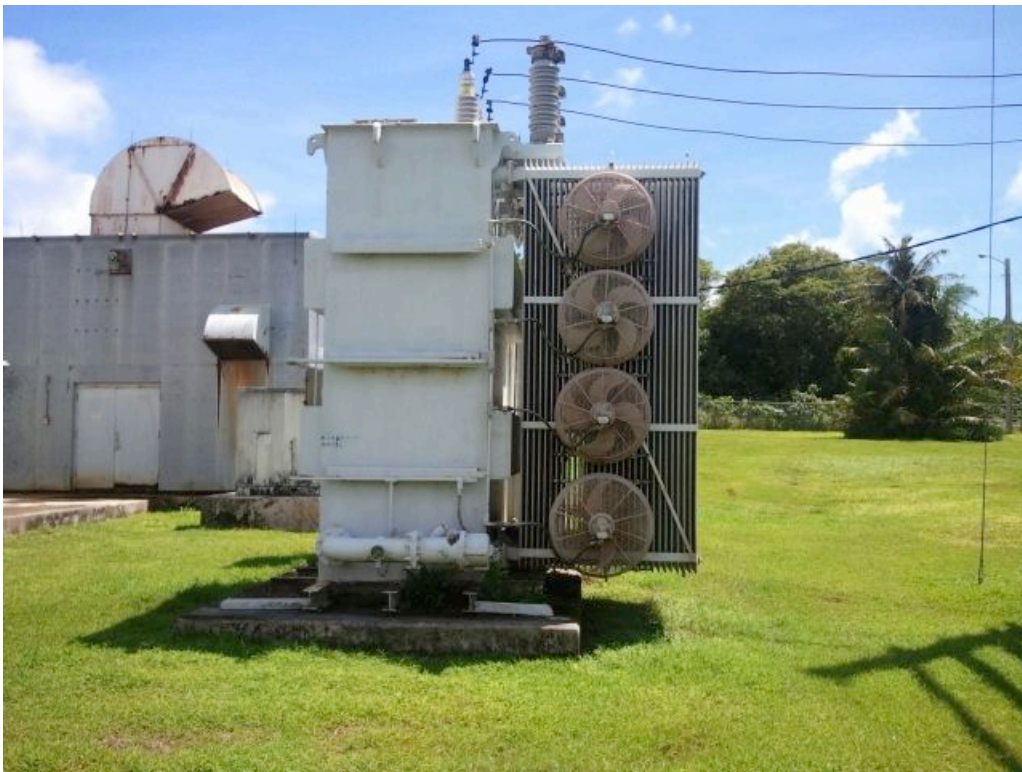
Photo P View of first transformer at MARBO Power Plant
