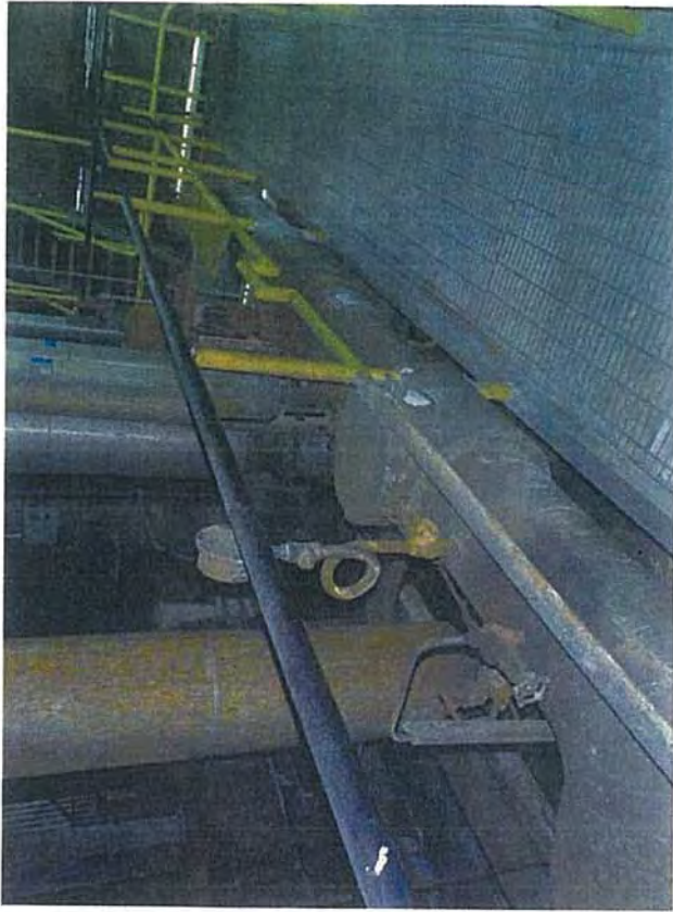
Mezzanine—C1—View of Pipes above Evaporator
