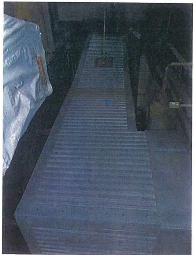
Ground Floor—E1—View of Boiler, APH Duct, and Tank Vent (left)
