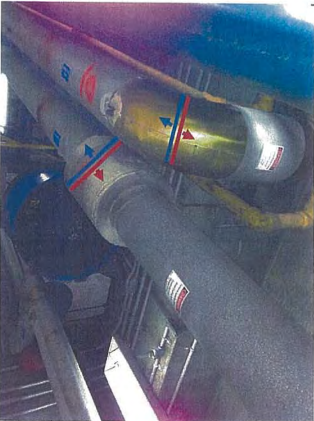
Basement—C2—View of Overhead Pipes; Asbestos (red)/Non-asbestos (blue) Junction
