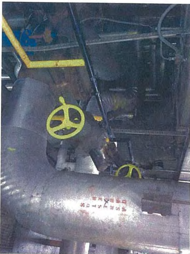
Ground Floor—B3—View of Condenser/HP Heater Pipes
