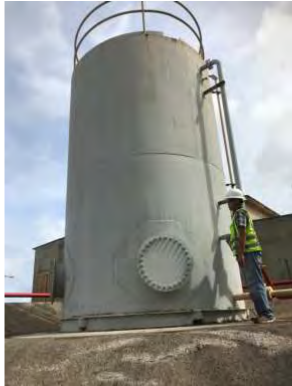
No. 2 light oil storage tank
