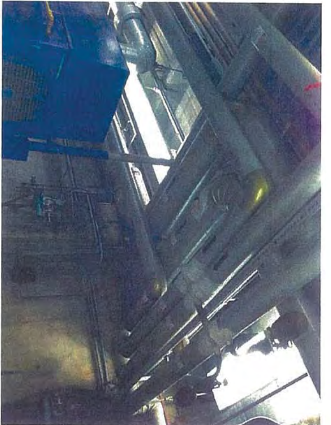
Basement—F2—View of Pipes along Staircase Leading to Upper Levels
