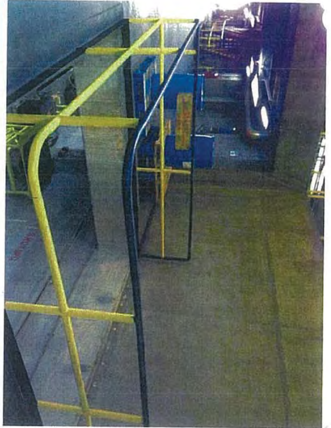
Ground Floor—C3—View of Crane Access
