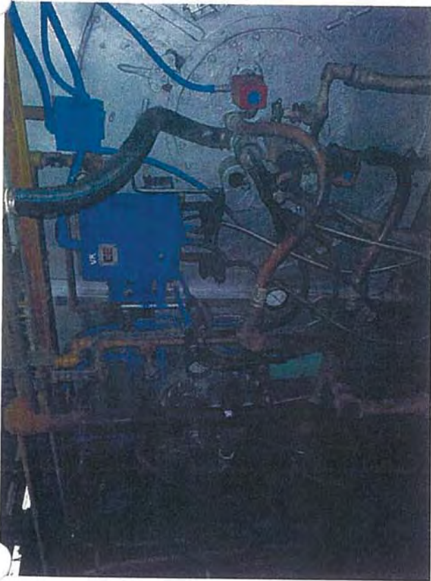
Mezzanine—B2—View of Boiler
