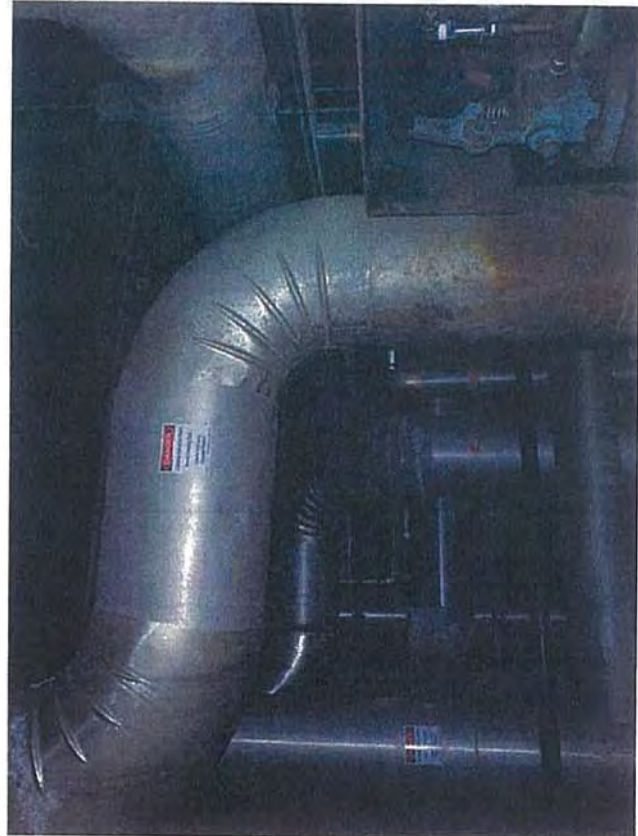
Mezzanine—E1—View of Pipes of Upper Mezzanine Deck
