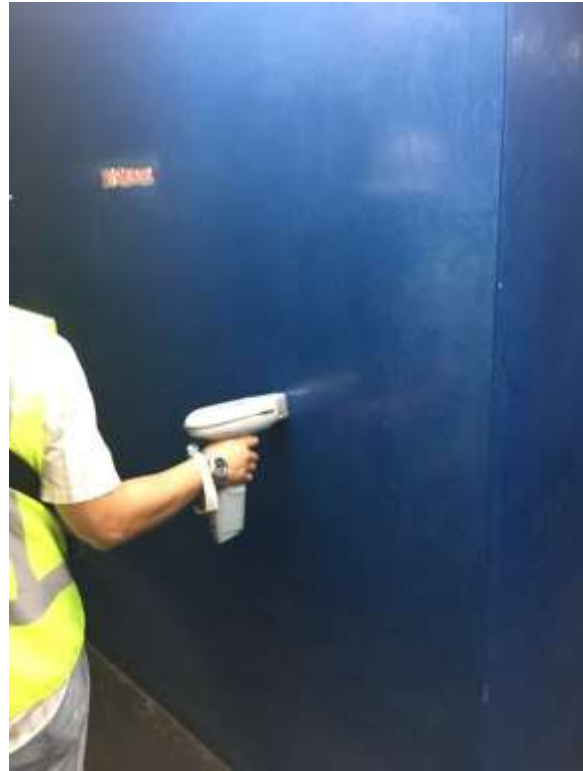
Blue switch panel
