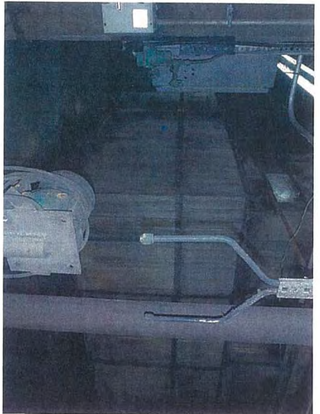
Mezzanine—B1—View of APH Duct
