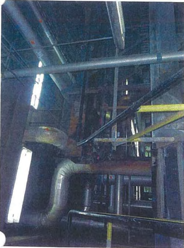
Mezzanine—E1—View of Upper Mezzanine Deck
