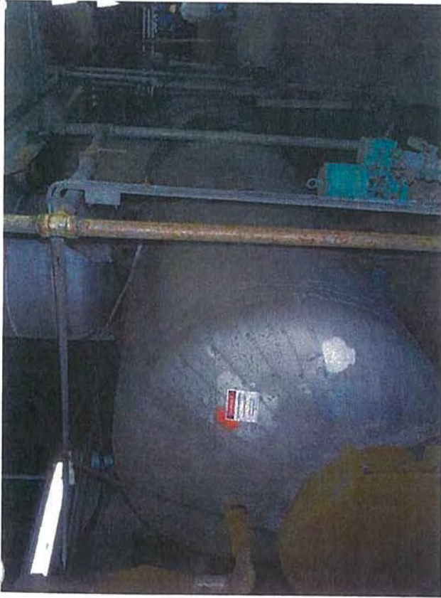
Turbine Deck—F1—View of Evaporator
