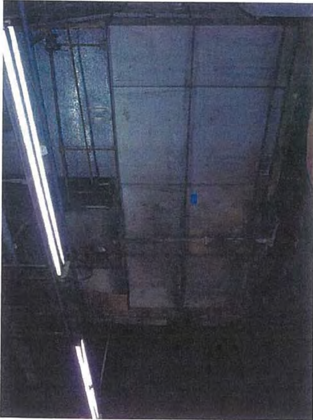
Mezzanine — E1 — View of APH Duct
