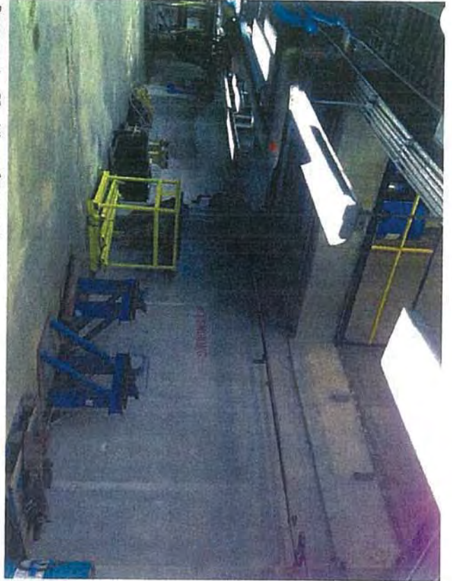
Basement—C3—View of Crane Access
