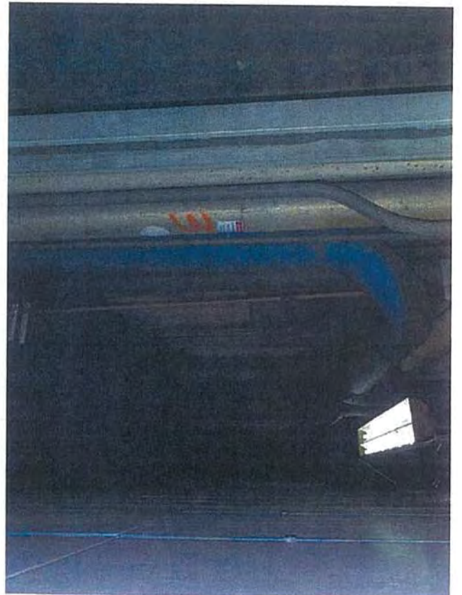
Turbine Deck—A1—View of Pipe Originating from Fuel Oil Pump (Ground Floor)
