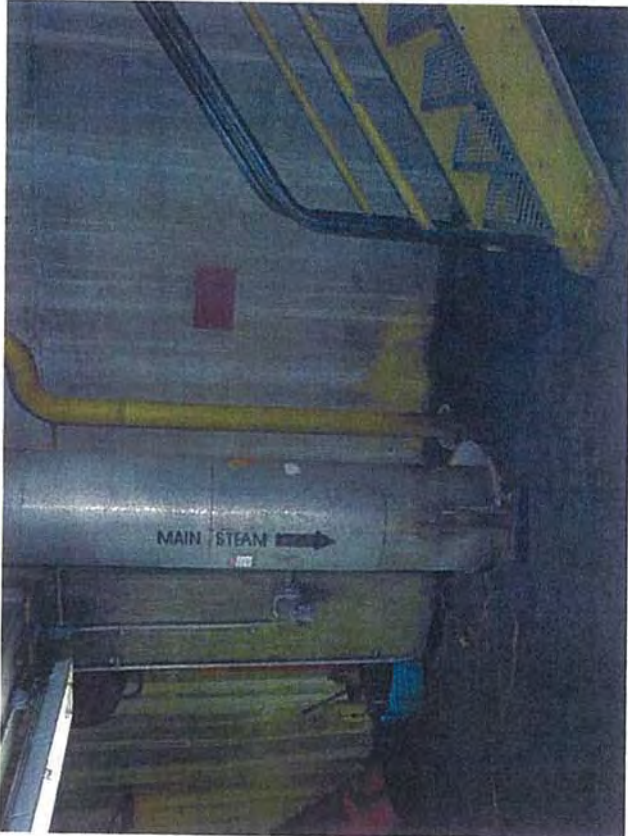
Turbine Deck—A2—View of Main Steam Line
