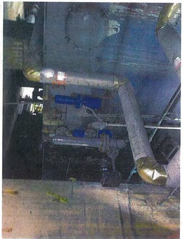
Basement—A2—View of Condenser Pipes
