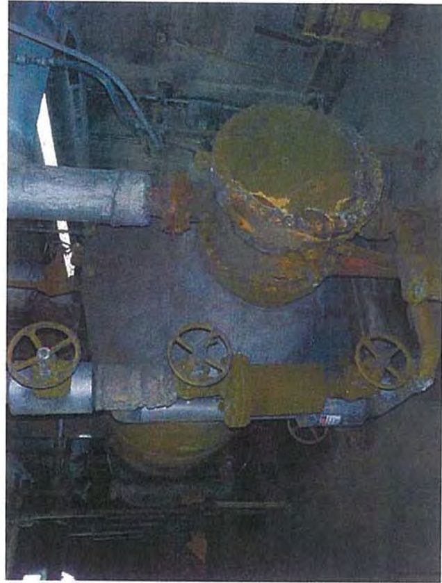
Turbine Deck—F1—View of Evaporator and Pipes
