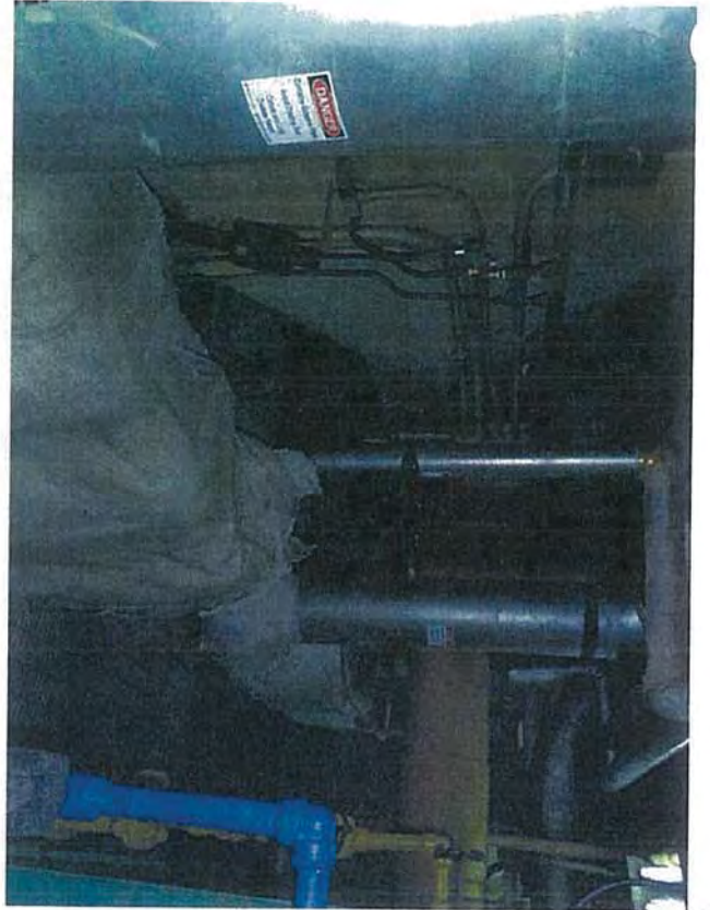
Ground Floor—E2—View of Condenser Pipes
