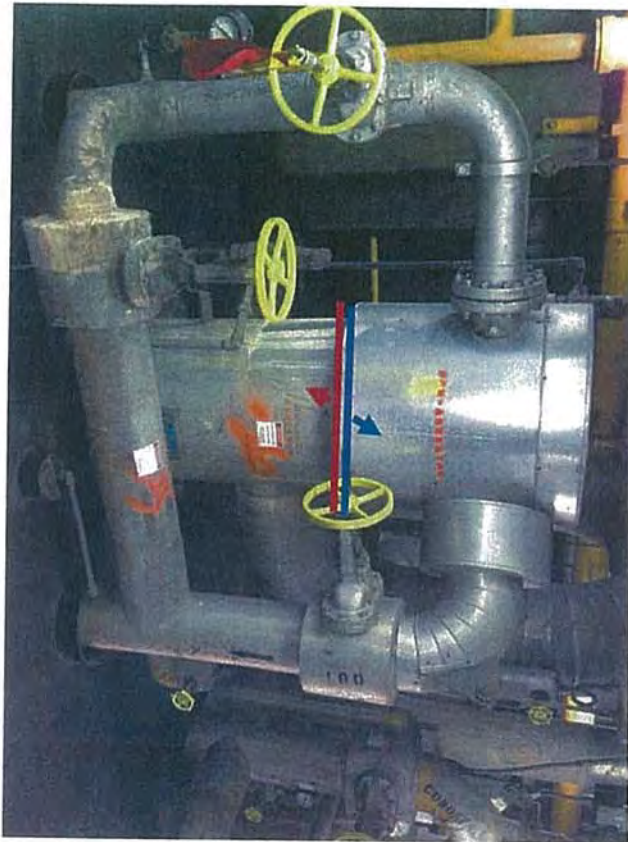
Ground Floor—B3—View of Air Eject Pipes; Asbestos (red)/Non-Asbestos (blue) Junction
