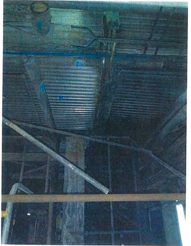
Mezzanine—B1—View of Boiler and Pipes
