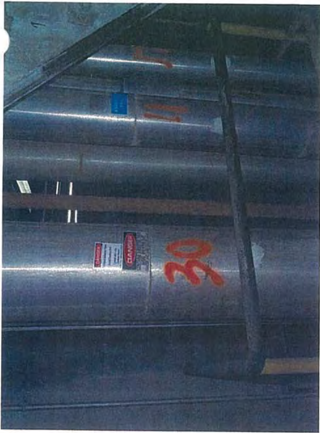
Drum Deck—C2—View of Pipes Along Staircase (Originating from Lower Levels)
