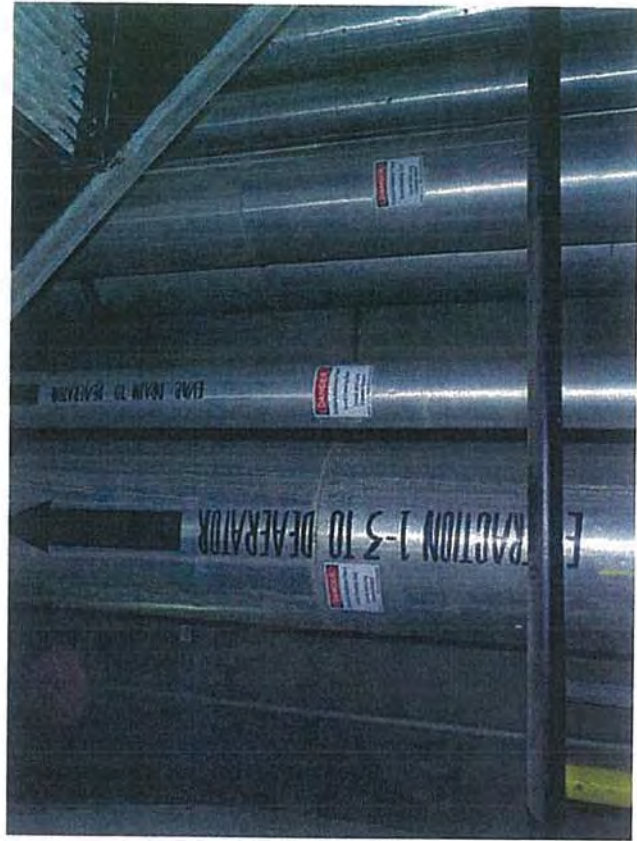
Drum Deck—F2—View of Pipes Along Staircase (Originating from Lower Levels)
