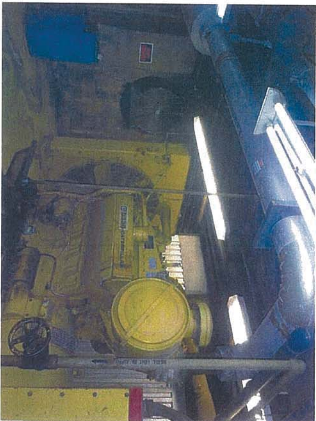
Ground Floor—D1—View of Generator and Exhaust
