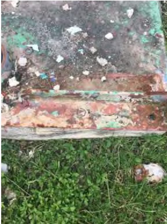
Old metal foundation
