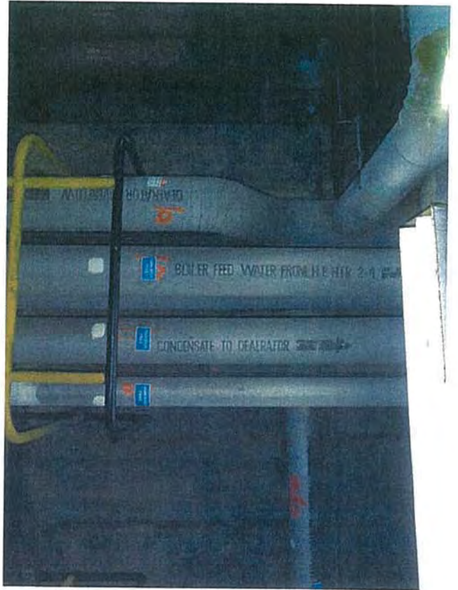
Ground Floor—C2—View of Pipes along Staircase
