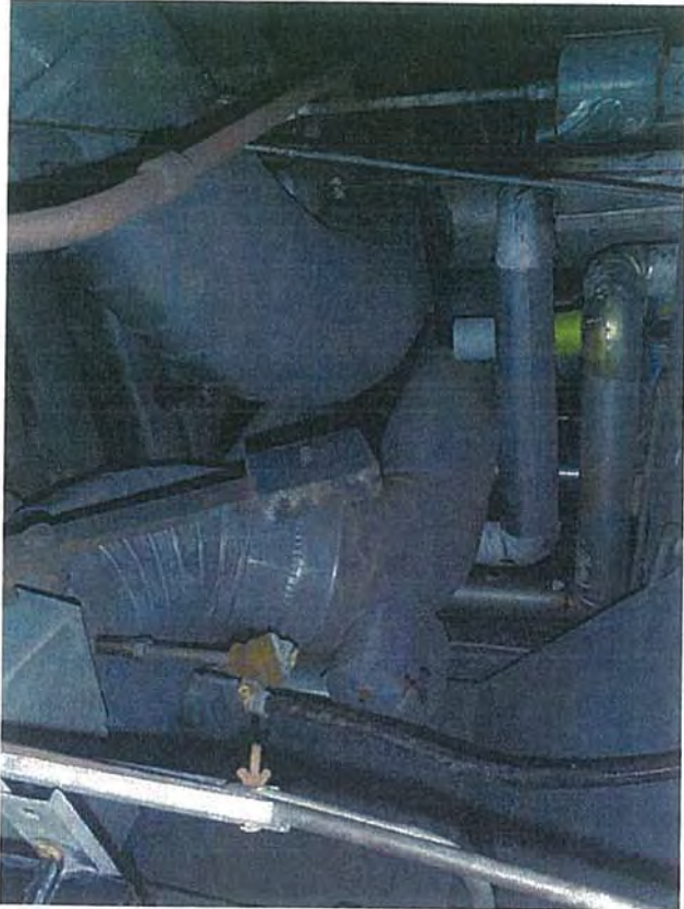
Ground Floor—E2—View of Condenser Pipes (Assumed to Contain Asbestos)
