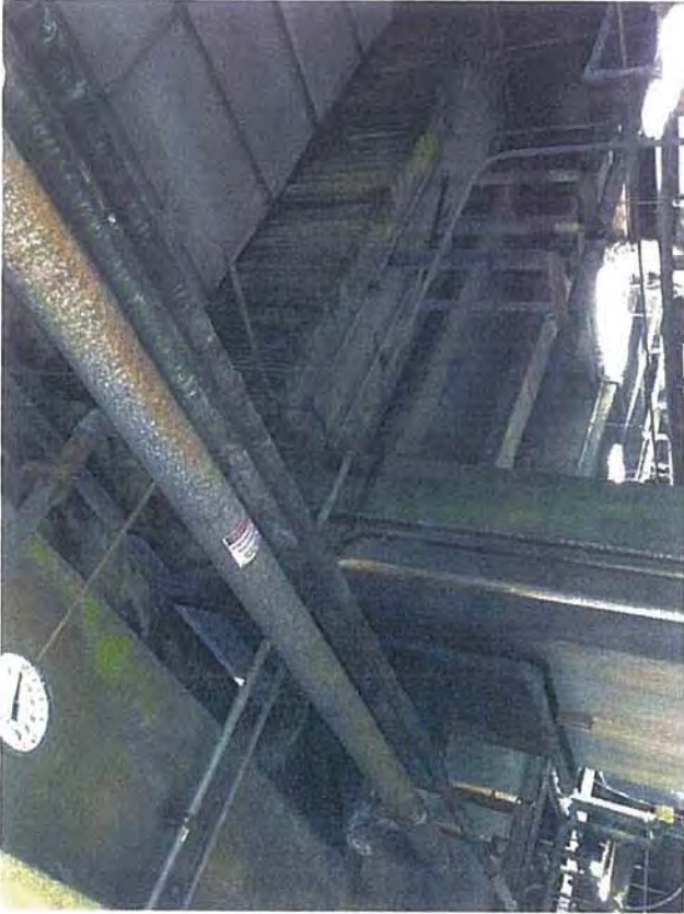
Basement—D1—View of Overhead Pipes
