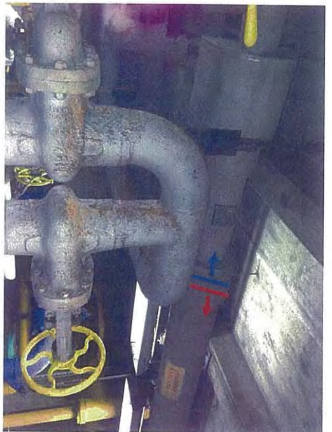
Ground Floor—A3—View of Air Eject Overhead Pipe; Asbestos (red)/Non-Asbestos (blue) Junction
