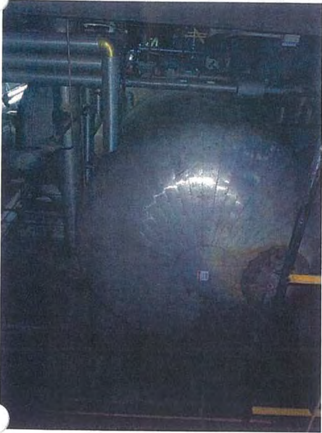
Drum Deck—F1—View of Deaerator Tank and Pipes
