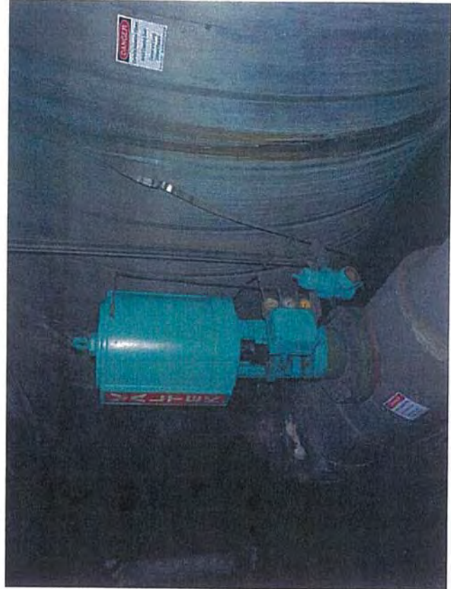
Drum Deck—C1—View of Deaerator Tank and Pipes
