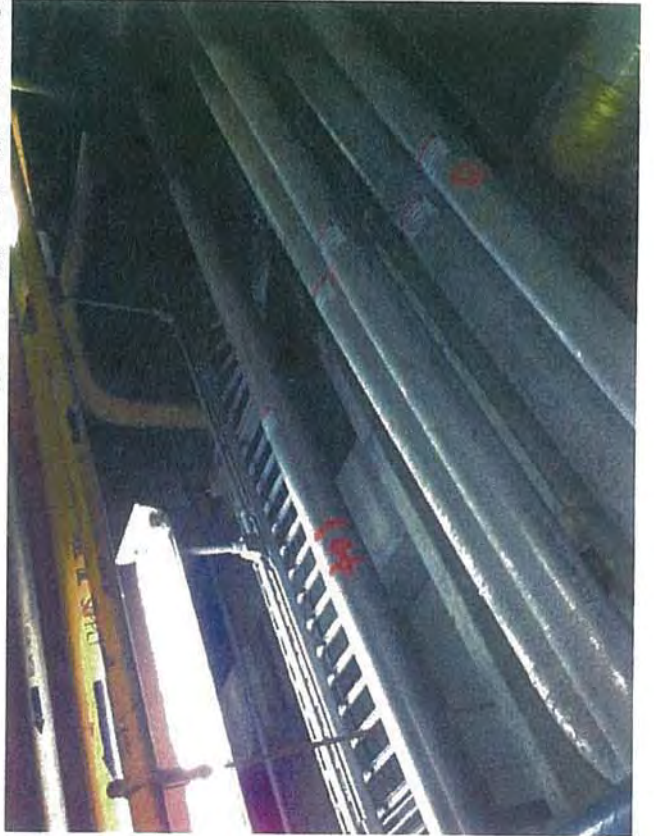
Basement—D2—View of Overhead Pipes
