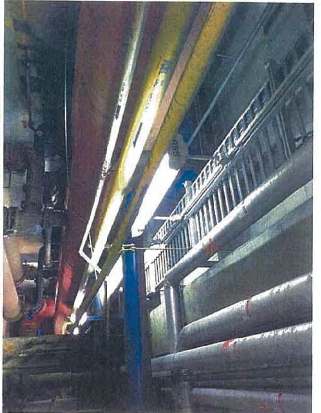
Basement—D2—View of Overhead Pipes, Heat Exchangers
