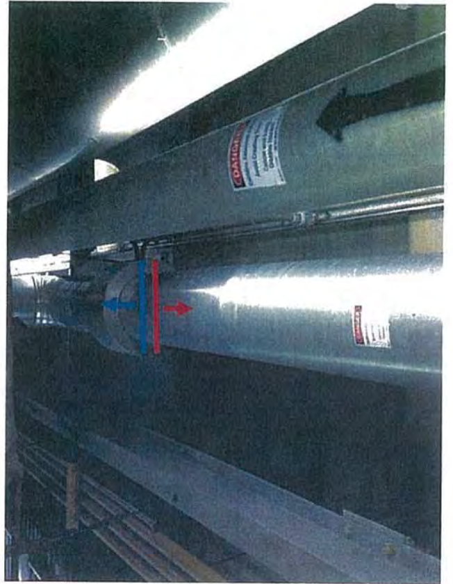
Basement—F1 — View of Overhead Pipes; Asbestos (red)/Non-Asbestos (blue) Junction
