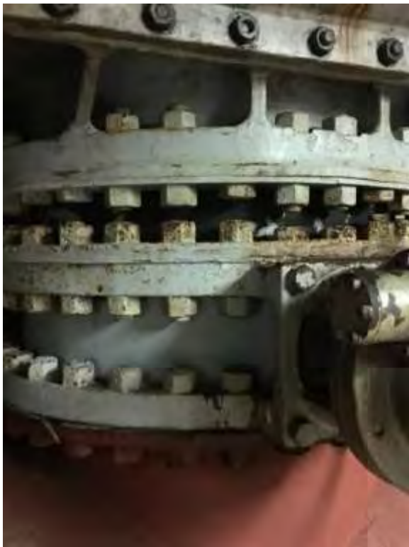
Condenser valve body
