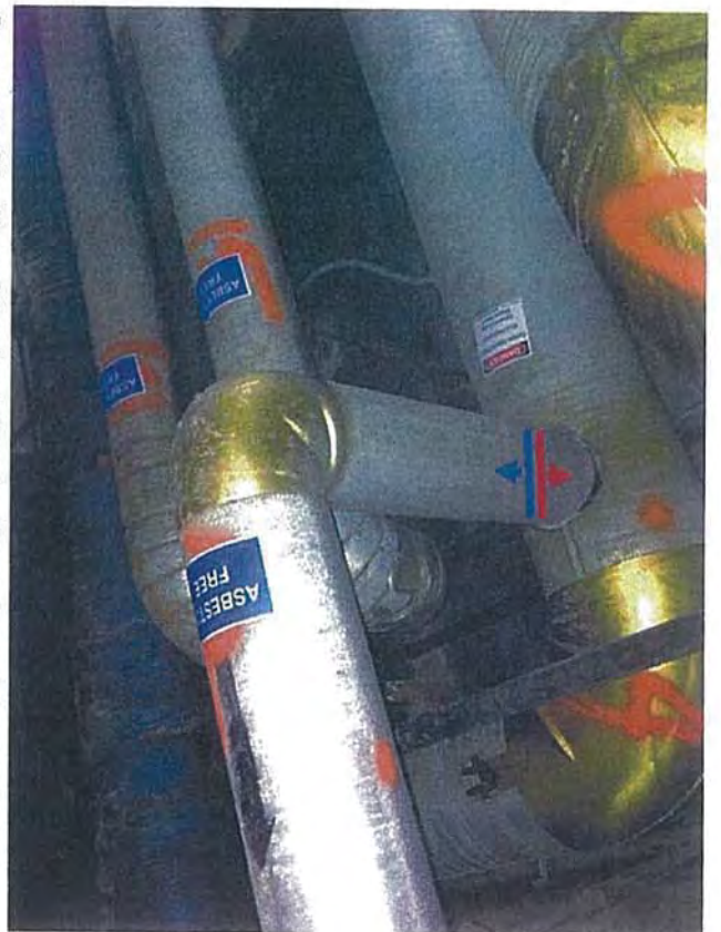
Basement—B2—View of Overhead Pipes Leading to Ground Floor; Asbestos (red)/Non-asbestos (blue) Junction
