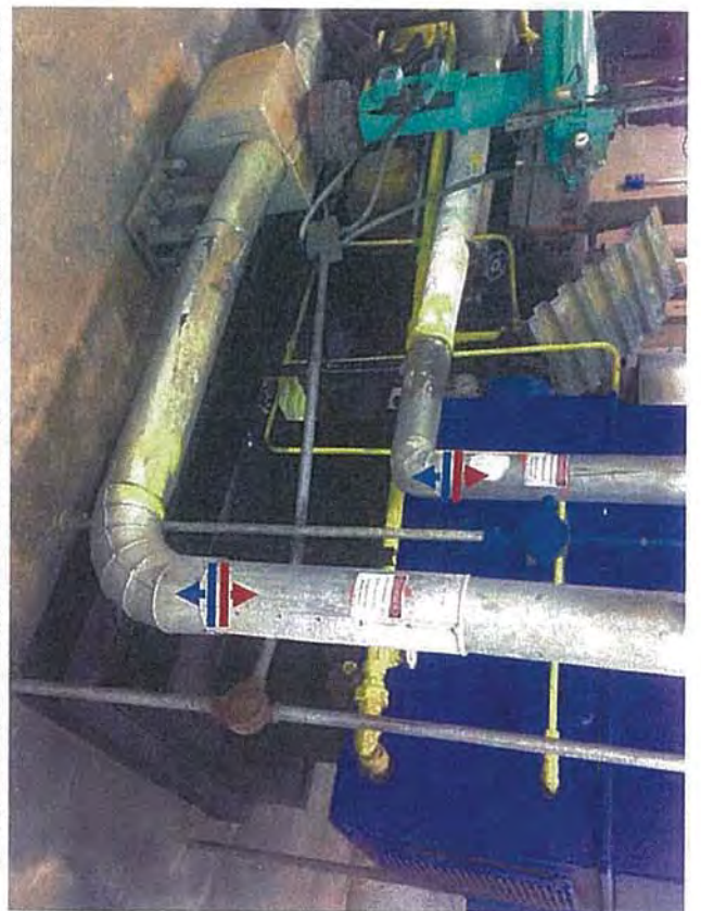
Basement—F1—View of BFWP and Pipes; Asbestos (red)/Non-Asbestos (blue) Junction
