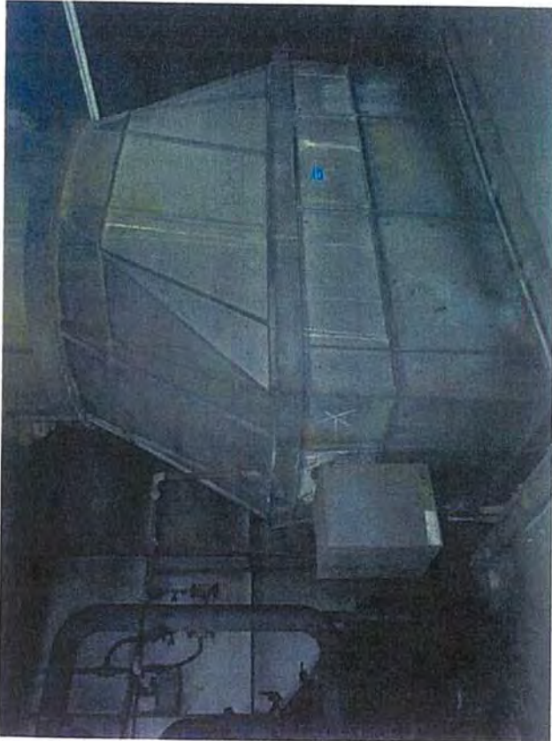
Drum Deck—E1—View of APH Duct
