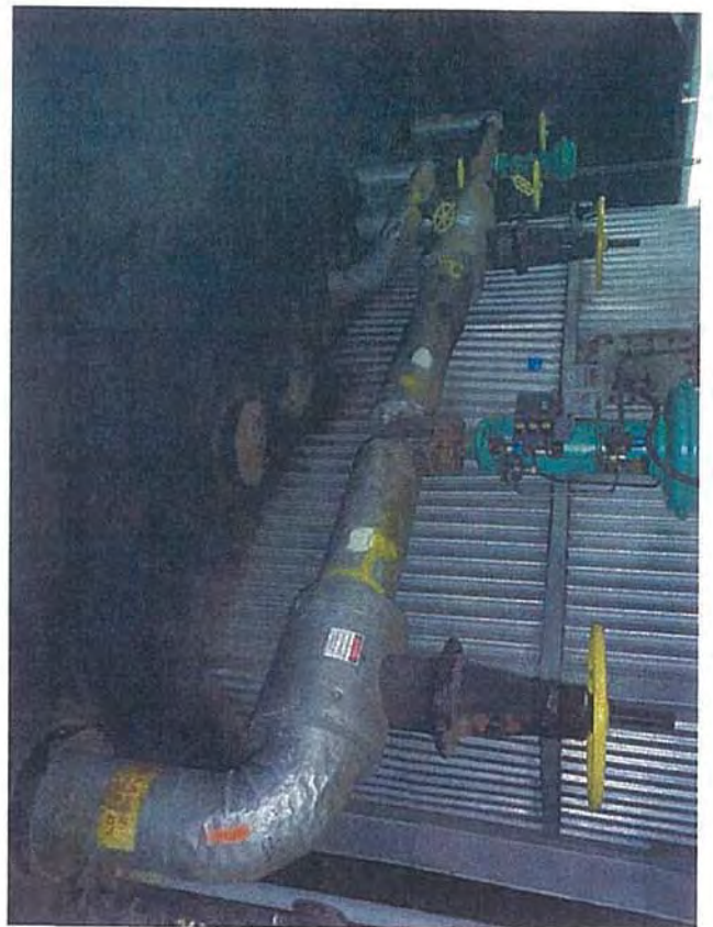
Ground Floor—E2—View of Boiler, Pipes, Valves Originating from Basement
