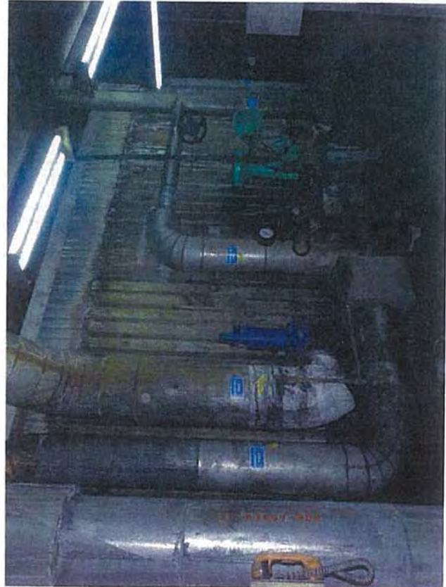
Drum Deck—B1—View of Boiler, Pipes, Tank Vent (left, Non-Asbestos only on Drum Deck)
