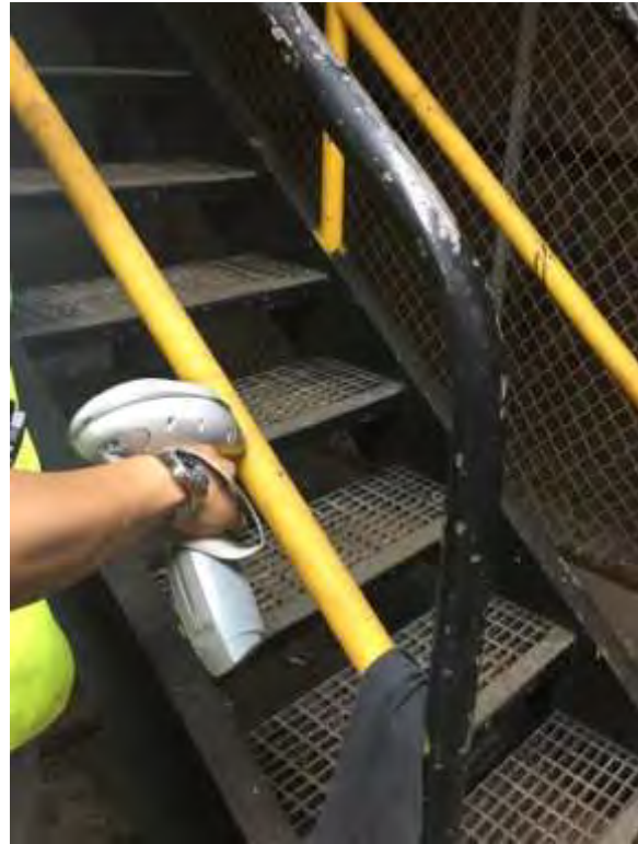
Yellow staircase railing
