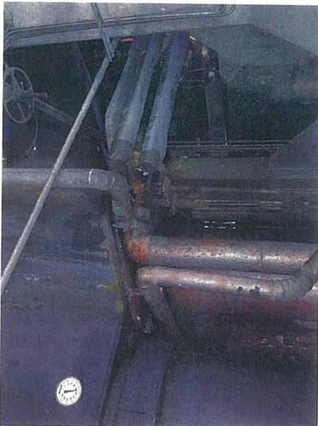
Ground Floor—A2—View of Condenser Pipes and Main Steam Line Asbestos (Red)/Non-Asbestos (Blue) Junction
