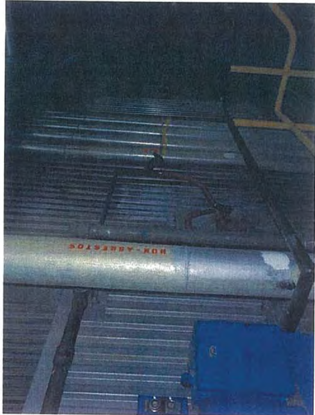
Mezzanine—B2—View of Boiler Pipes
