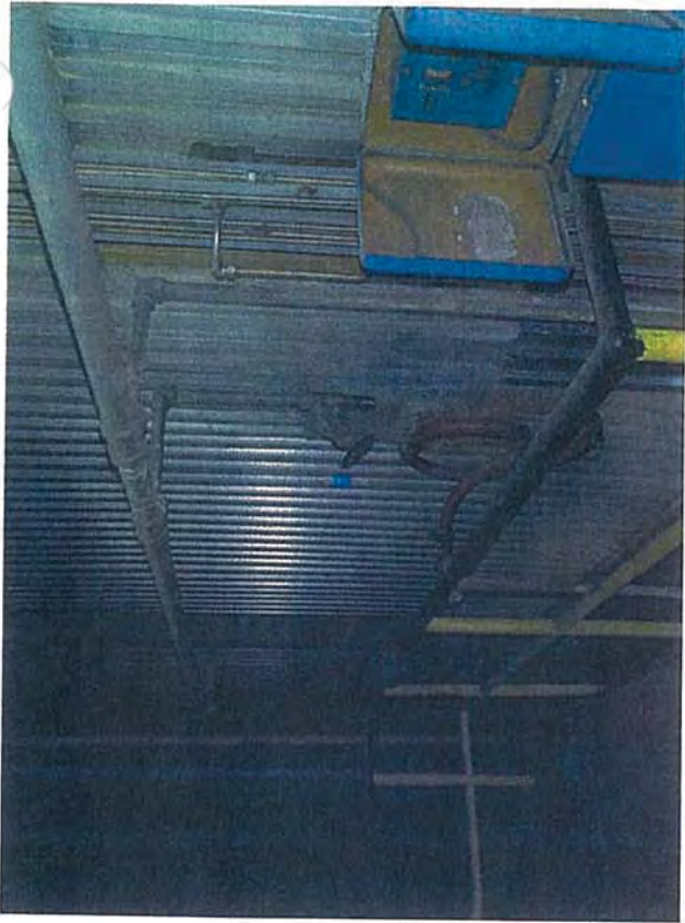
Mezzanine — B2 — View of Boiler
