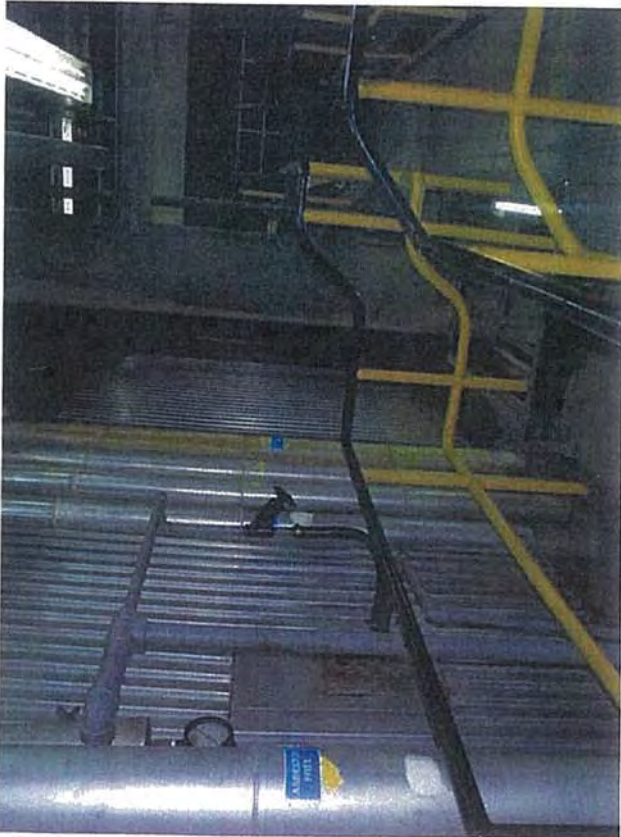
Mezzanine—E2—View of Boiler and Pipes
