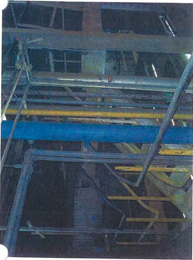
Mezzanine —D1—View of Pipe from Fuel Oil Pump (Originating from Ground Floor)
