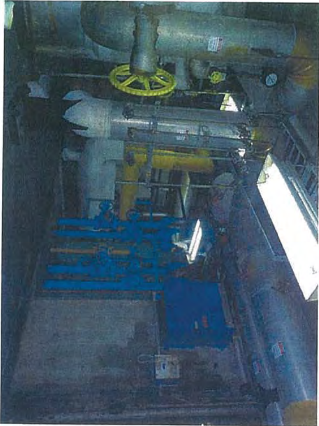
Ground Floor—B2—View of Condenser Pipes, HP Heater Pipes, and Overhead Pipes
