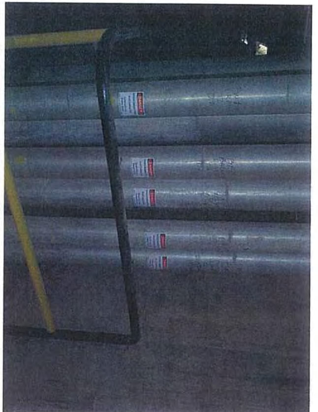
Turbine Deck—F2—View of Pipes along Staircase Originating from Lower Levels
