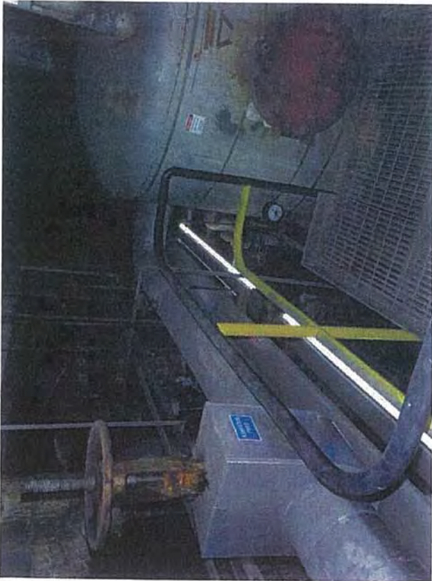
Drum Deck—F1—View of Pipes above Deaerator Tank
