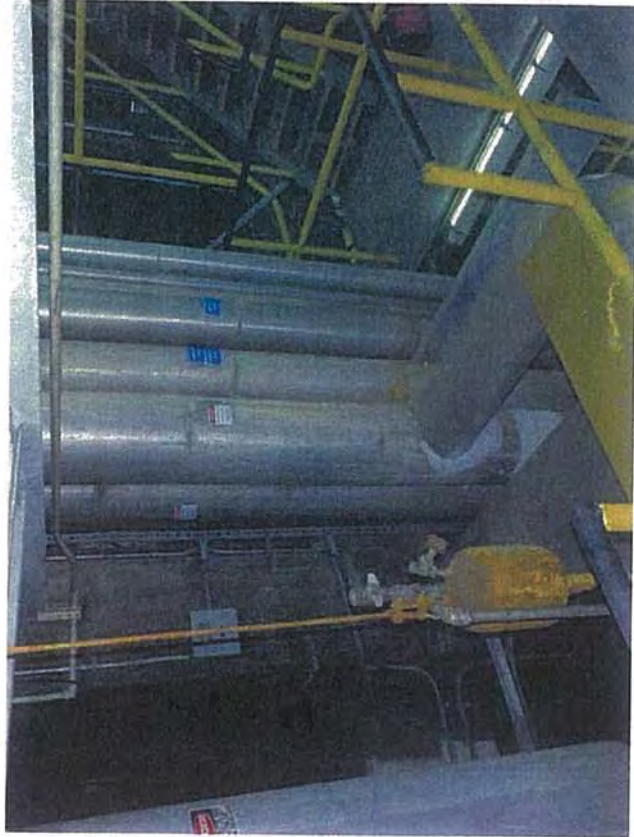
Mezzanine—C2—View of Pipes Along Staircase (Originating from Lower Levels)
