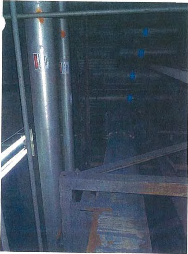
Mezzanine—E1—View of Pipes of Upper Mezzanine Deck, Boiler Pipes
