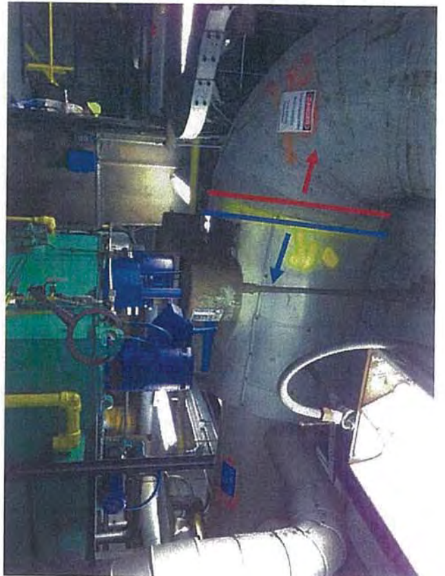
Ground Floor—A2—View of Condenser Pipes and Main Steam Line Asbestos (Red)/Non-Asbestos (Blue) Junction
