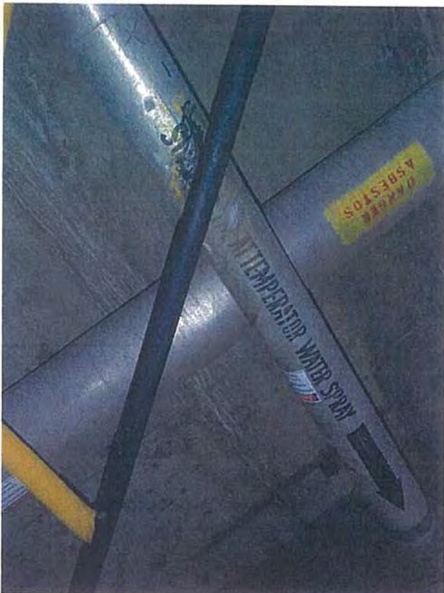
Ground Floor—F2—View of Pipes Along Staircase
