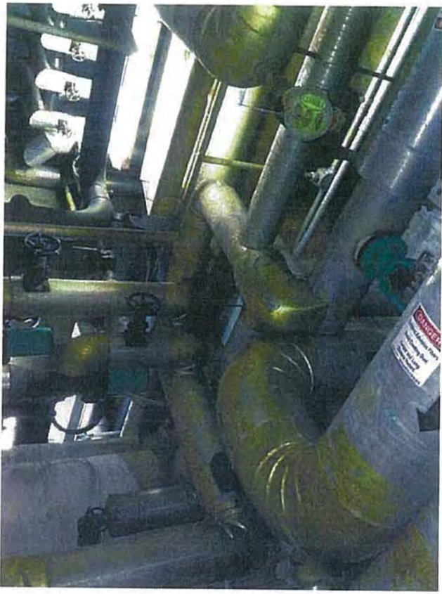
Basement—E2—View of Condenser/LP Heater Overhead Pipes
