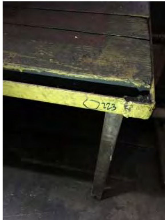
Yellow platform frame
