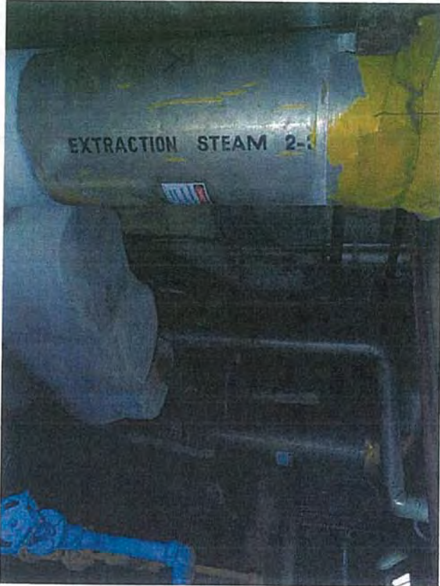
Ground Floor—B2—View of Condenser Pipes
