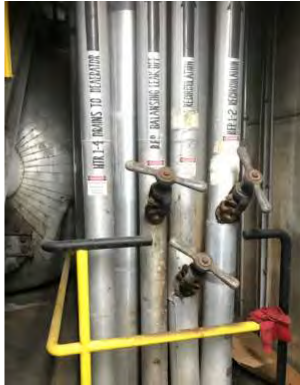
Example of a 9 inch asbestos pipe
