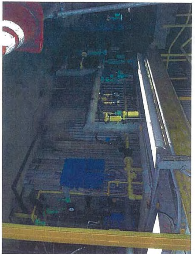
Turbine Deck—E2—View of Boiler and Pipes
