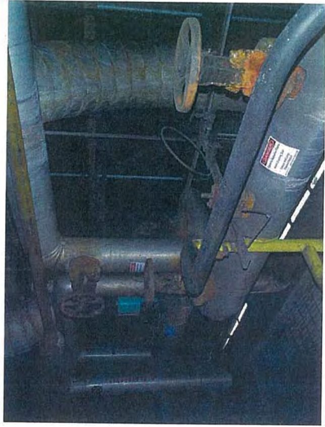
Drum Deck—C1—View of Pipes above Deaerator Tank
