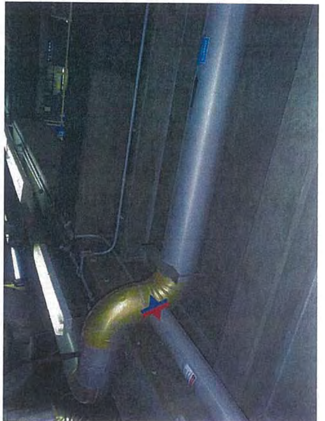
Ground Floor—B2—View of Overhead Pipes Asbestos (Red)/Non-Asbestos (Blue) Junction
