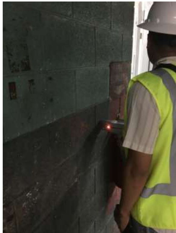
Basement green wall
