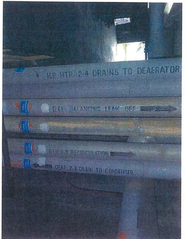
Ground Floor—C2—View of Pipes along Staircase
