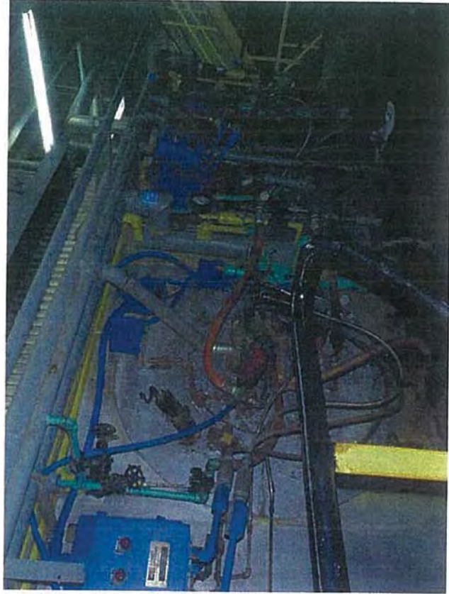
Mezzanine—E2—View of Boiler and Pipes
