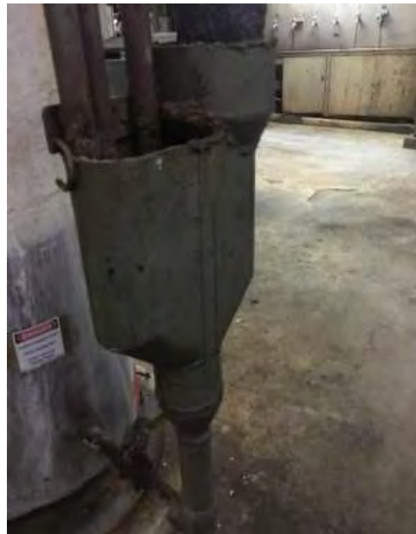
Example of a 10 foot asbestos tank
