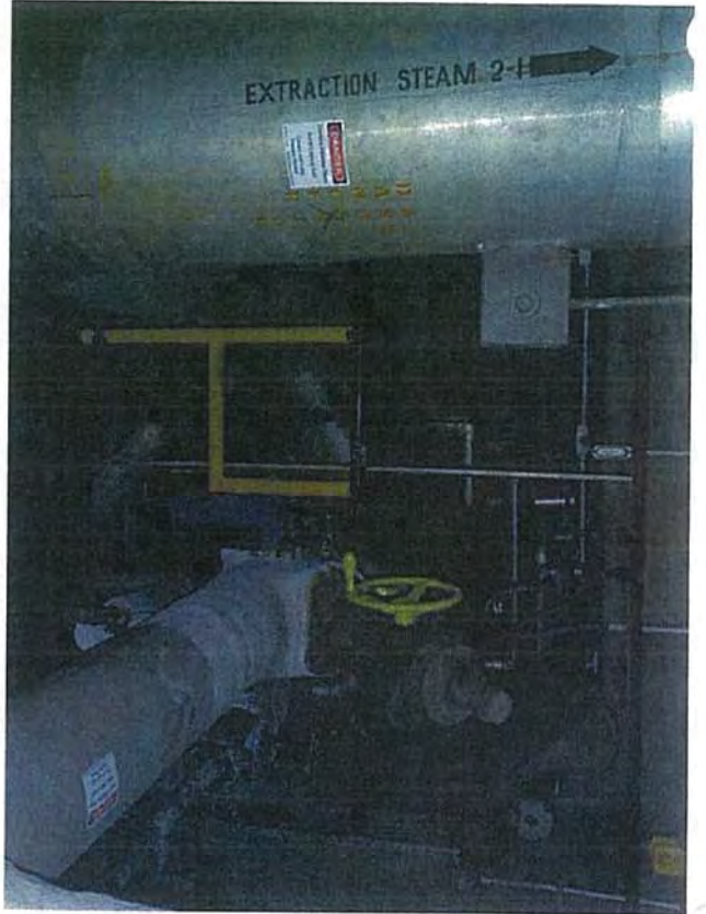
Ground Floor—B2—View of HP Heater/Condenser Pipes
