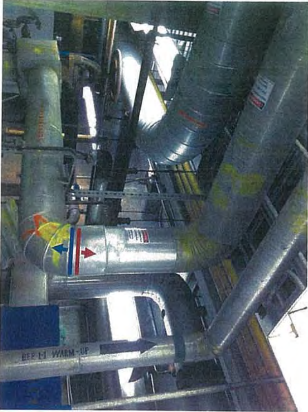
Basement—F1—View of BFWP and Overhead Pipes; Asbestos (red)/Non-Asbestos (blue) Junction
