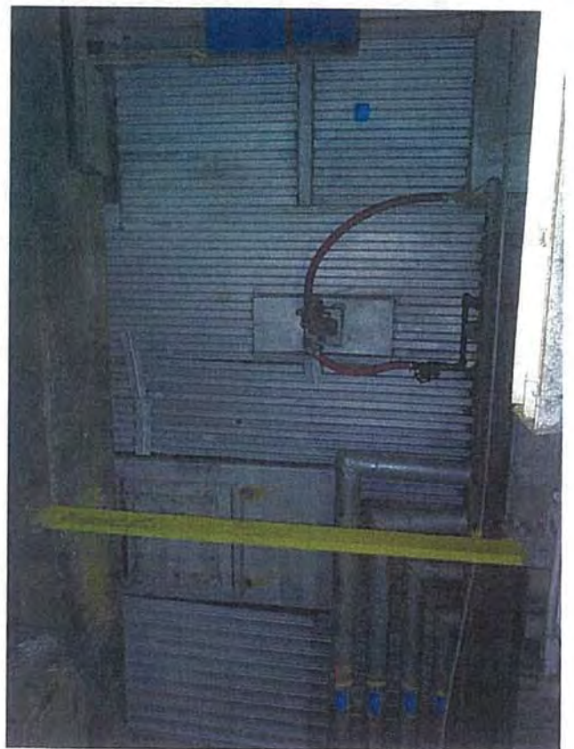
Turbine Deck—B2—View of Boiler and Pipes
