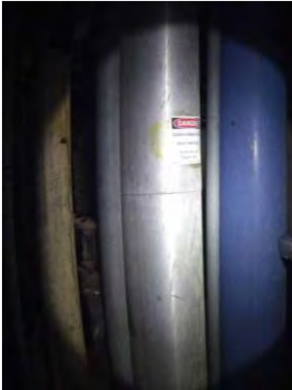
Example of a 4 foot asbestos pipe
