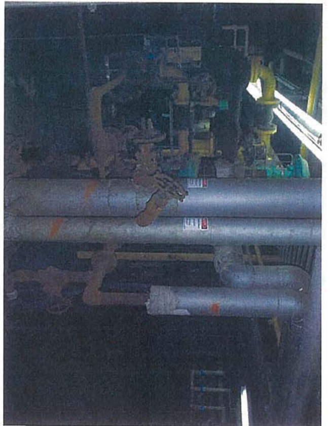
Ground Floor—D1—View of Fuel Oil Pump and Pipes
