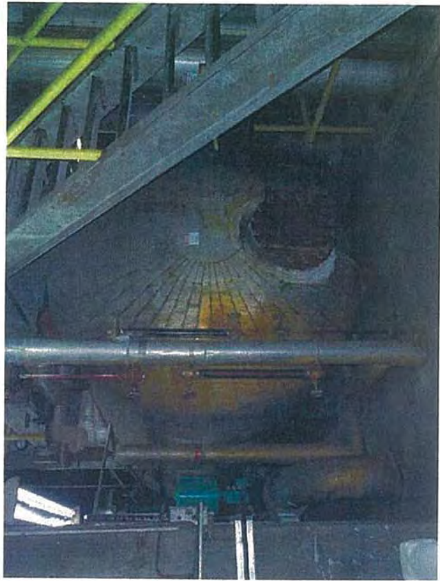
Drum Deck—C2—View of Deaerator Tank and Pipes
