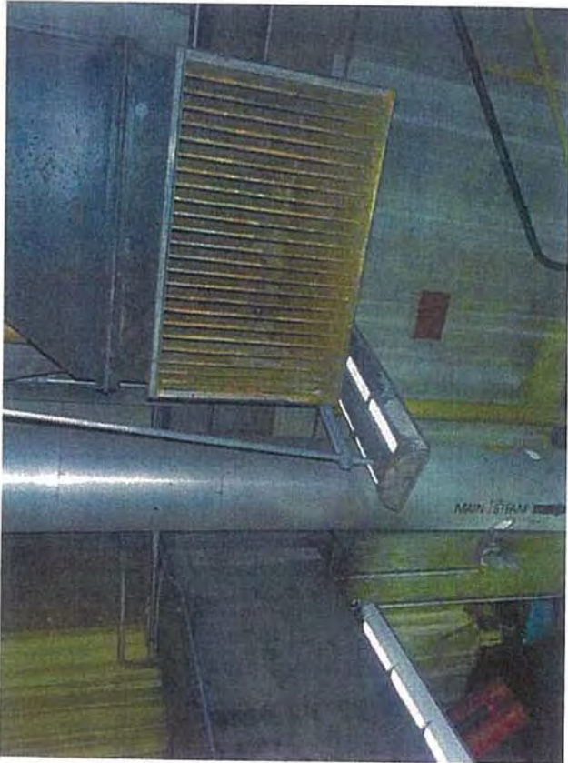
Mezzanine—A2—View of Main Steam Line
