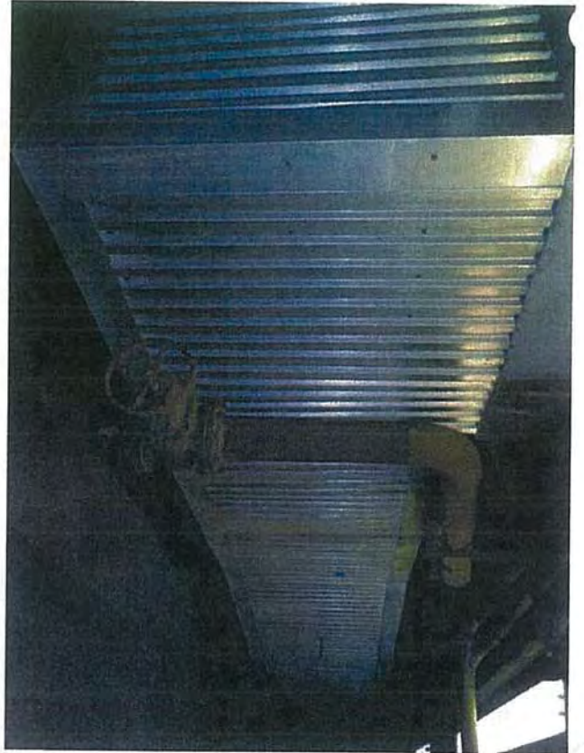
Ground Floor—E1—View of Boiler and APH Duct
