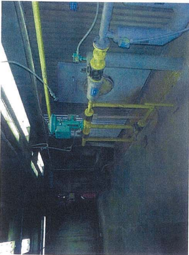
Turbine Deck—E1—View of Boiler
