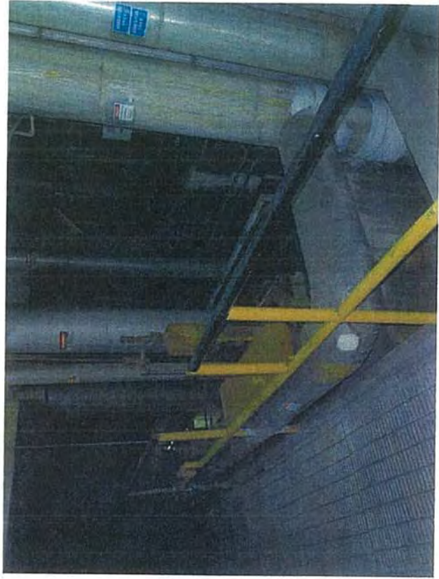
Mezzanine—C2—View of Pipes above Evaporator
