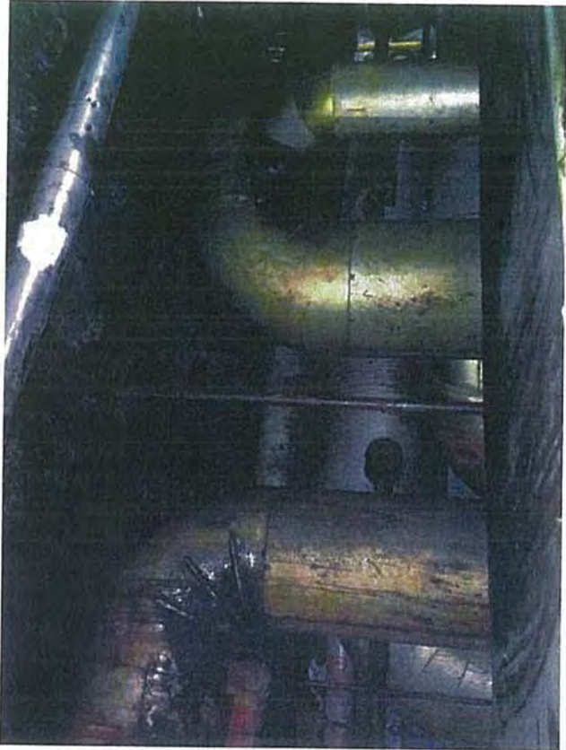
Ground Floor—A2—View of Condenser Pipes (Assumed to Contain Asbestos)
