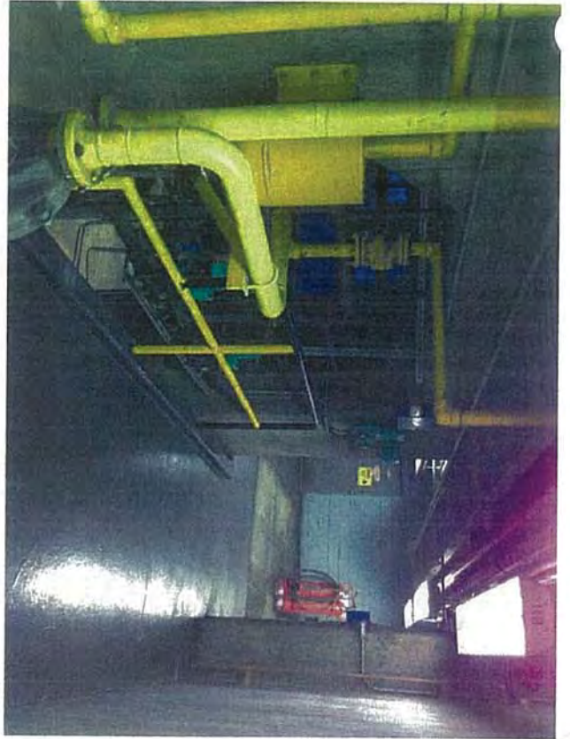
Ground Floor—A3—View of Condenser
