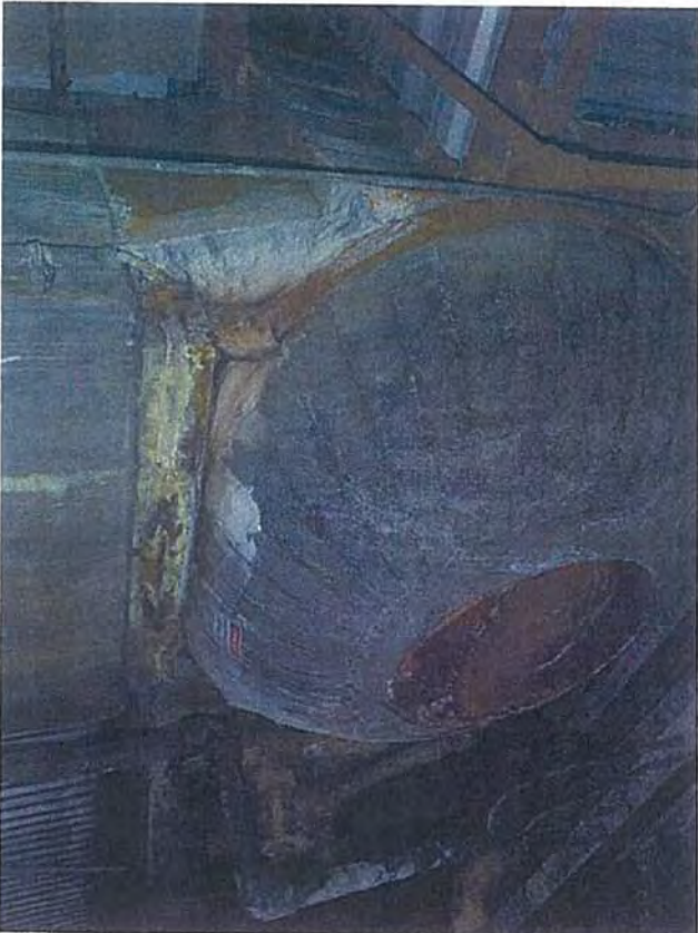
Ground Floor—B1—View of Boiler Hatch
