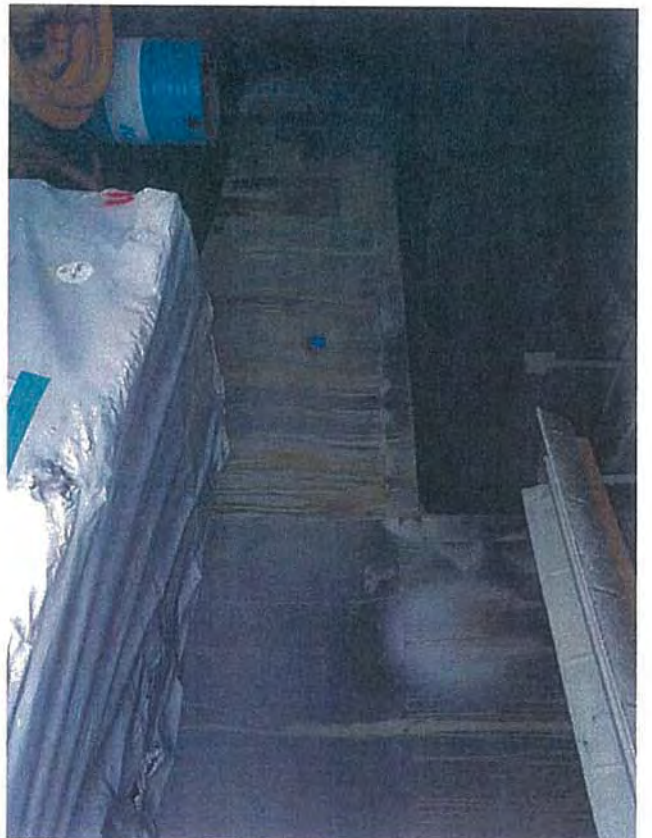
Ground Floor—B1—View of APH Duct
