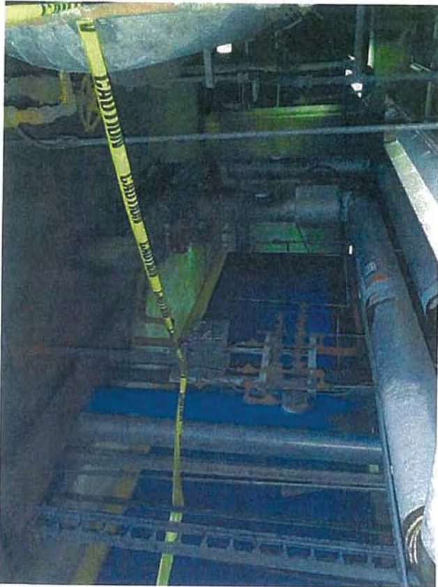
Turbine Deck—C1—View of Evaporator, Pipes, and Valves
