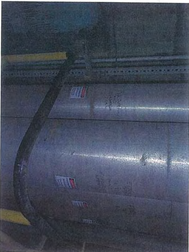
Turbine Deck—F2—View of Pipes along Staircase Originating from Lower Levels
