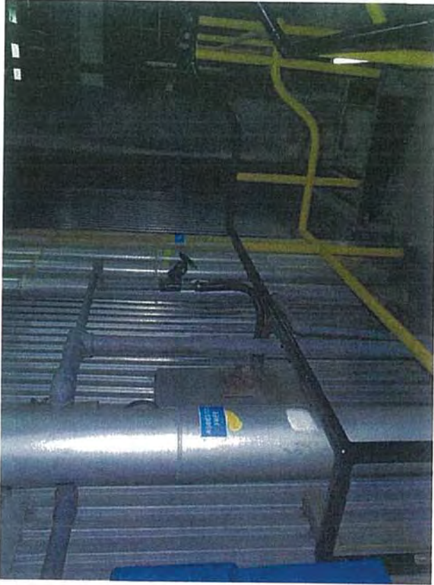
Mezzanine—E2—View of Boiler and Pipes
