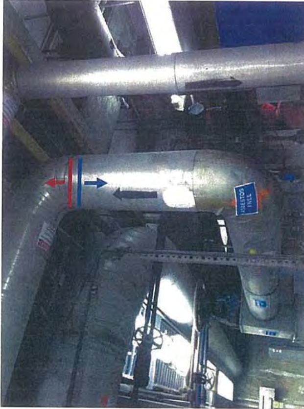
Basement—C1—View of BFWP and Pipes; Asbestos (red)/Non-Asbestos (blue) Junction
