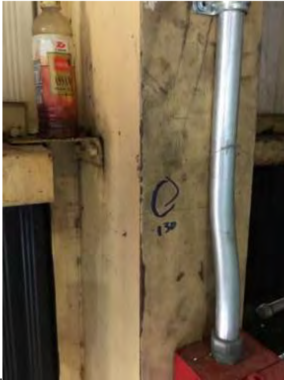
Yellow metal beam
