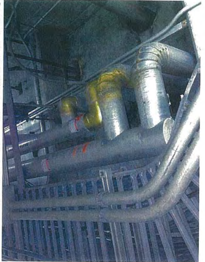
Basement—B3—View of Overhead Pipes Leading to Air Eject of Ground Floor
