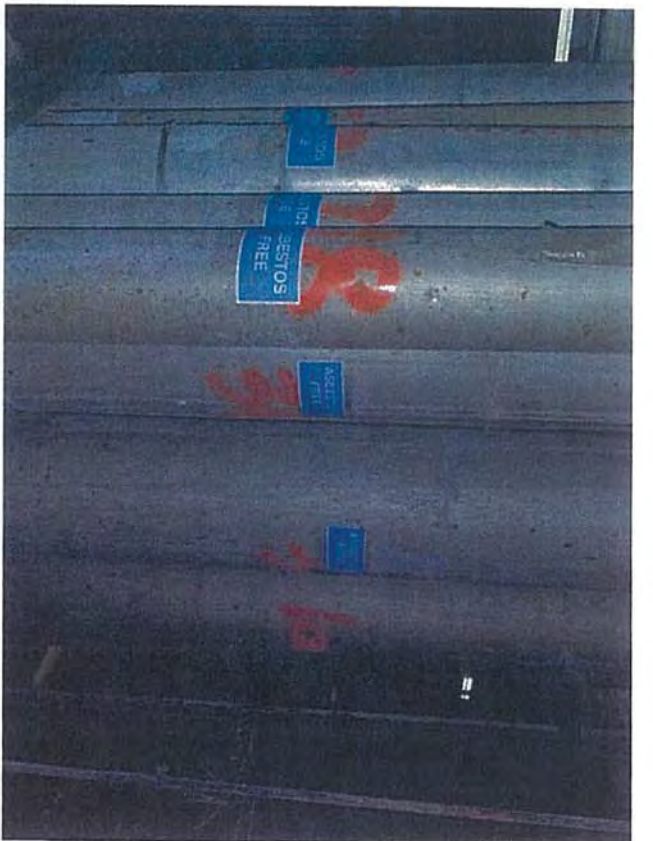
Turbine Deck—C2—View of Pipes along Staircase Originating from Lower Levels
