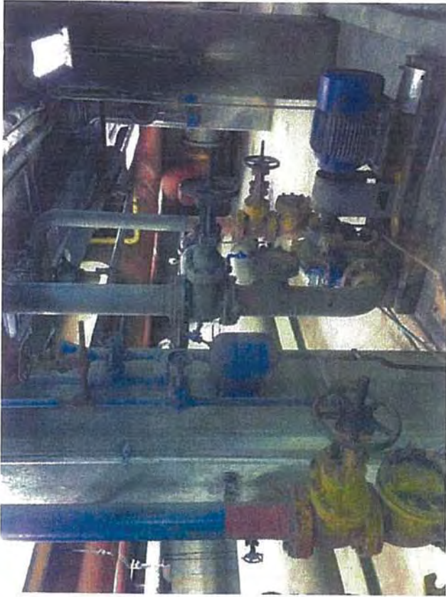
Basement—A1—View of Heat Exchangers, Pumps
