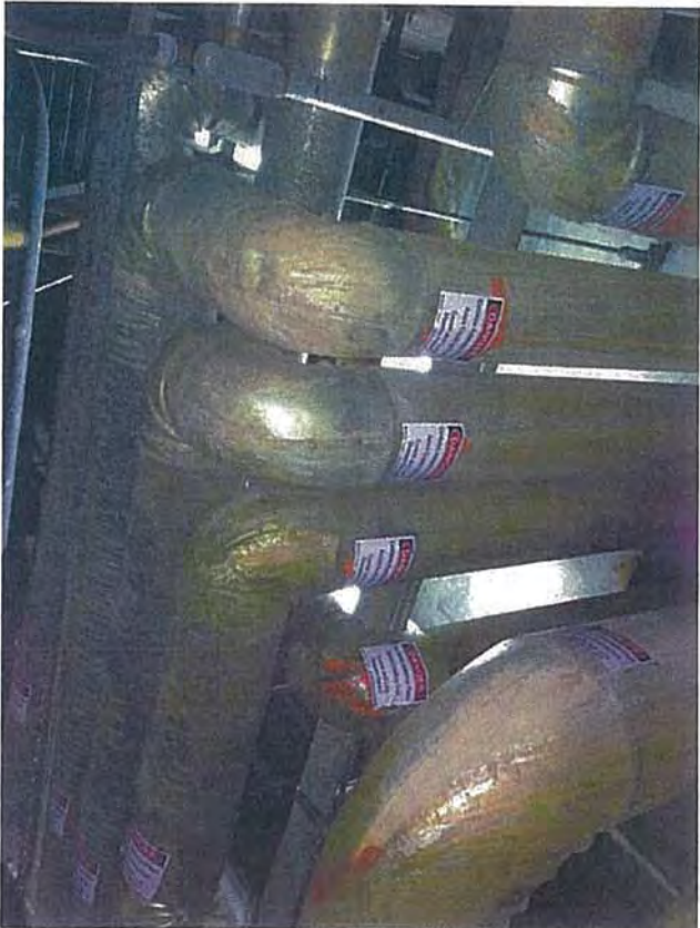
Basement—F2—View of Pipes along Staircase Leading to Upper Levels
