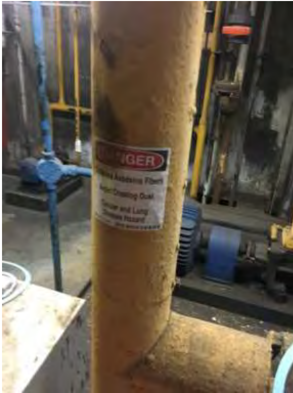
Example of a 2 foot asbestos pipe
