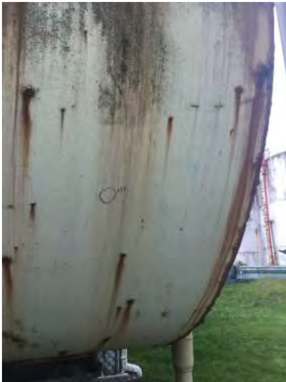
Water tank north of engine No. 4
