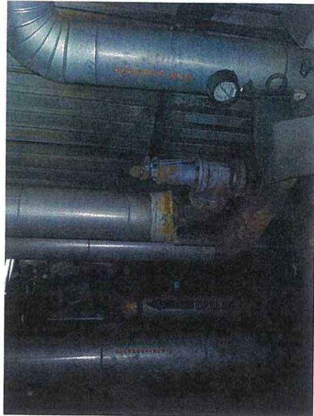
Drum Deck—E1—View of Boiler, Pipes, and Tank Vent (left, Non-Asbestos only on Drum Deck)
