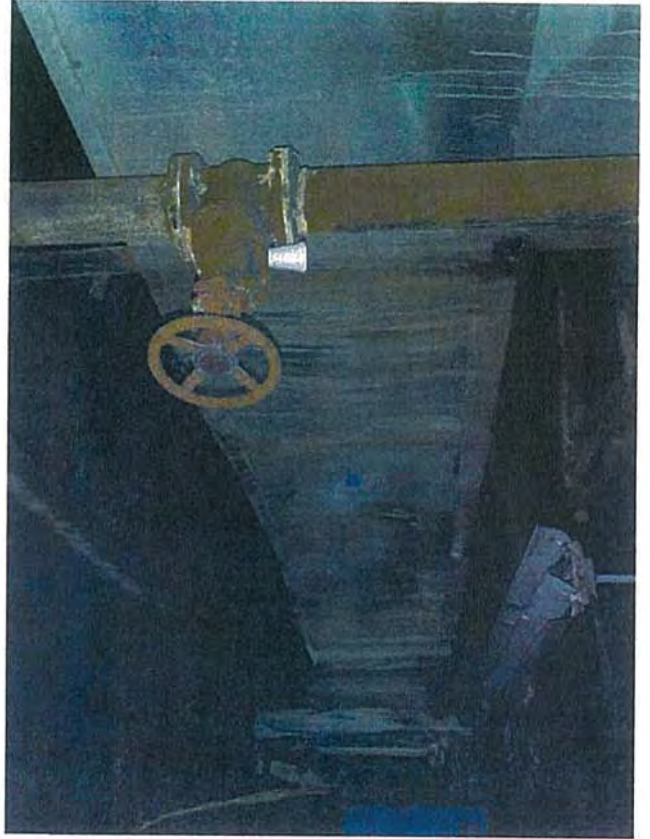
Ground Floor—B1—View of APH Duct
