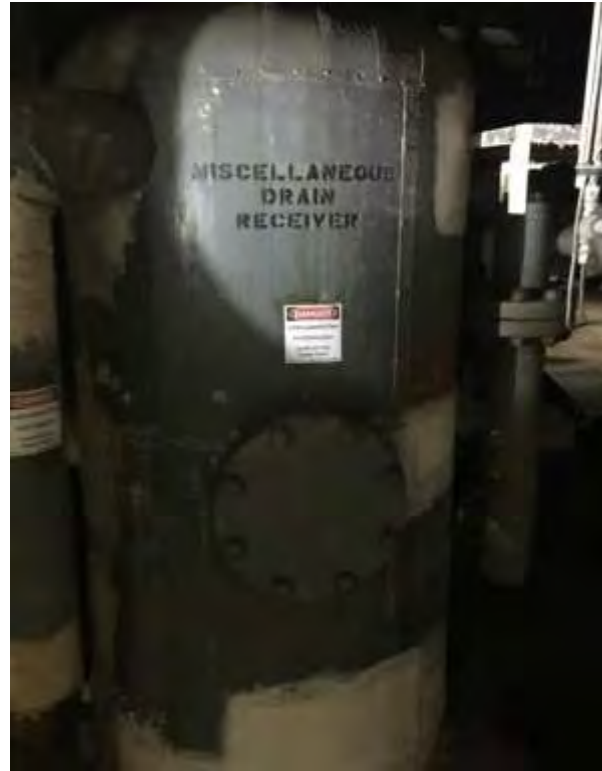
Example of a 8 foot asbestos tank
