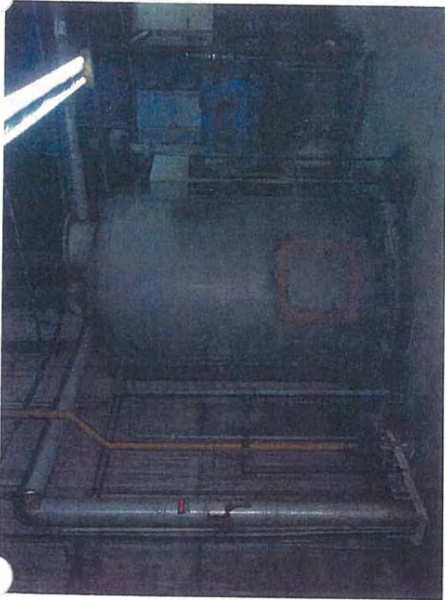
Drum Deck—A1—View of Pipe from Fuel Oil Pump from Ground Floor
