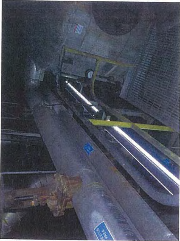
Drum Deck—C1—View of Pipes above Deaerstor Tank
