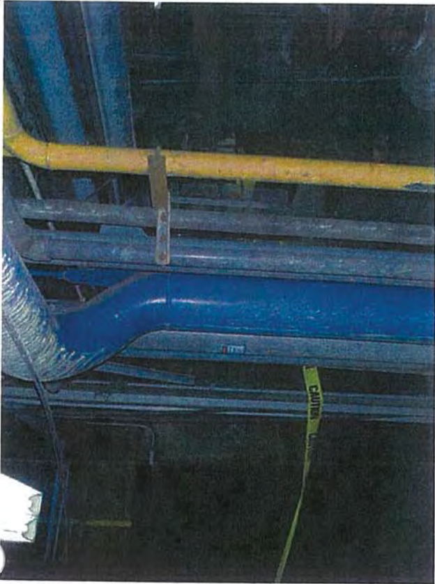
Turbine Deck—D1—View of Pipe Originating from Fuel Oil Pump
