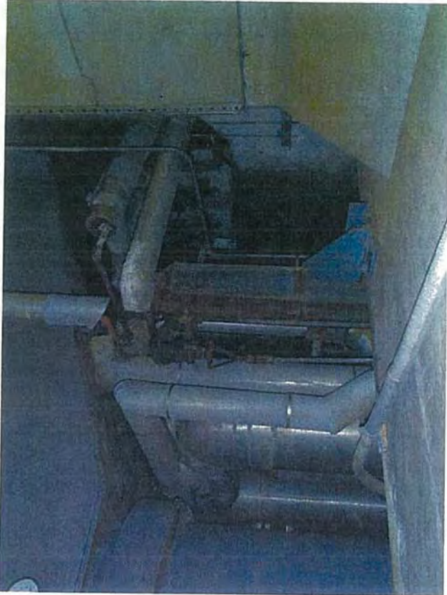
Ground Floor—D2—View of Condenser Pipes (Assumed to Contain Asbestos)
