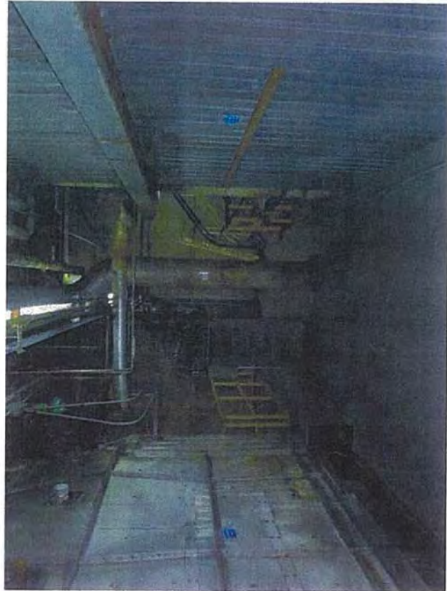
Mezzanine — E1 — View of APH Duct, Boiler, Tank Vent
