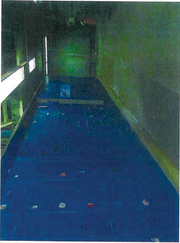
Turbine Deck—D1—View of 480V Panel, CST
