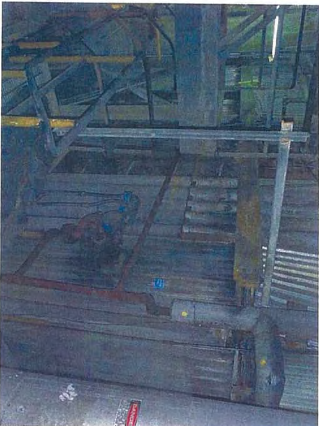
Mezzanine—B1—View of Boiler and Tank Vent (right)
