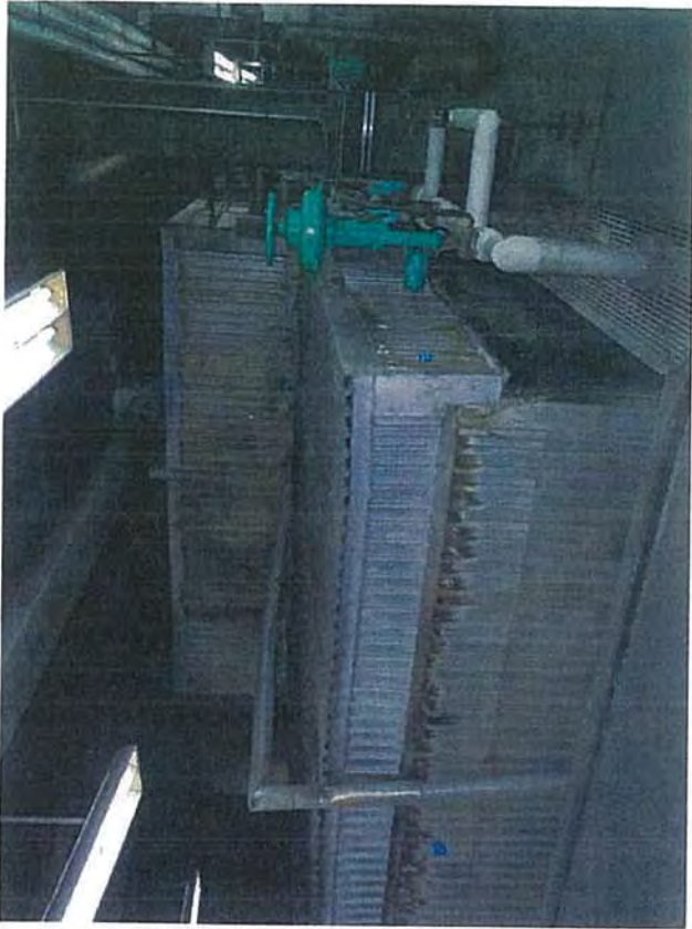
Drum Deck—B2—View of Boiler
