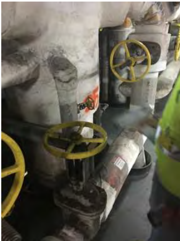
Example of a 3 foot asbestos pipe
