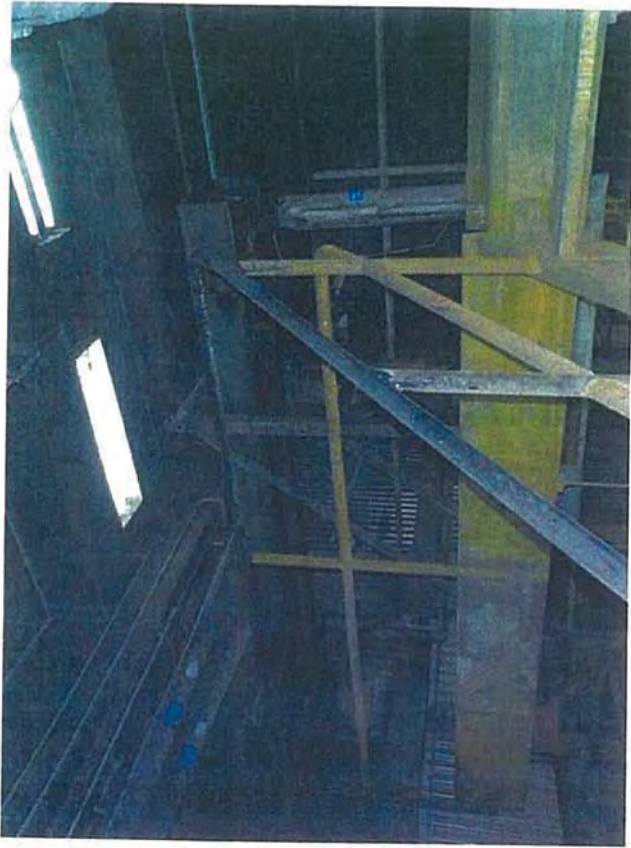
Mezzanine —D1—View of Upper Mezzanine Pipes
