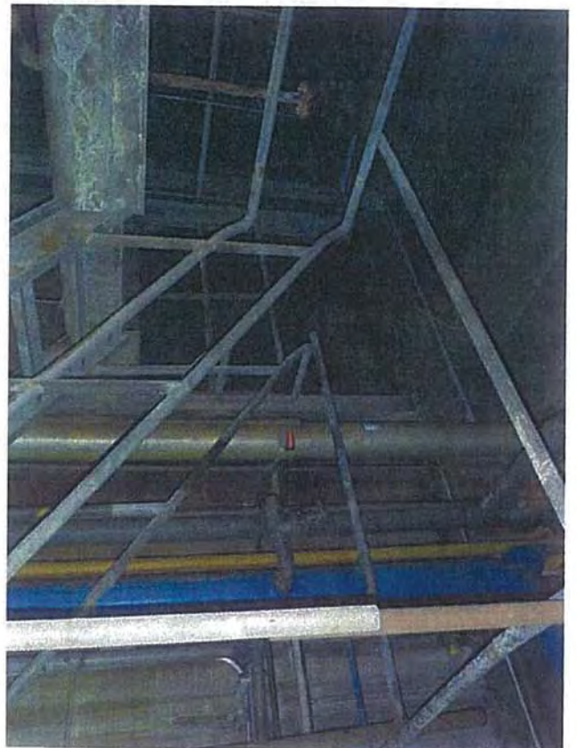
Mezzanine Deck—A1—View of Pipe from Fuel Oil Pump (Originating from Ground Floor)
