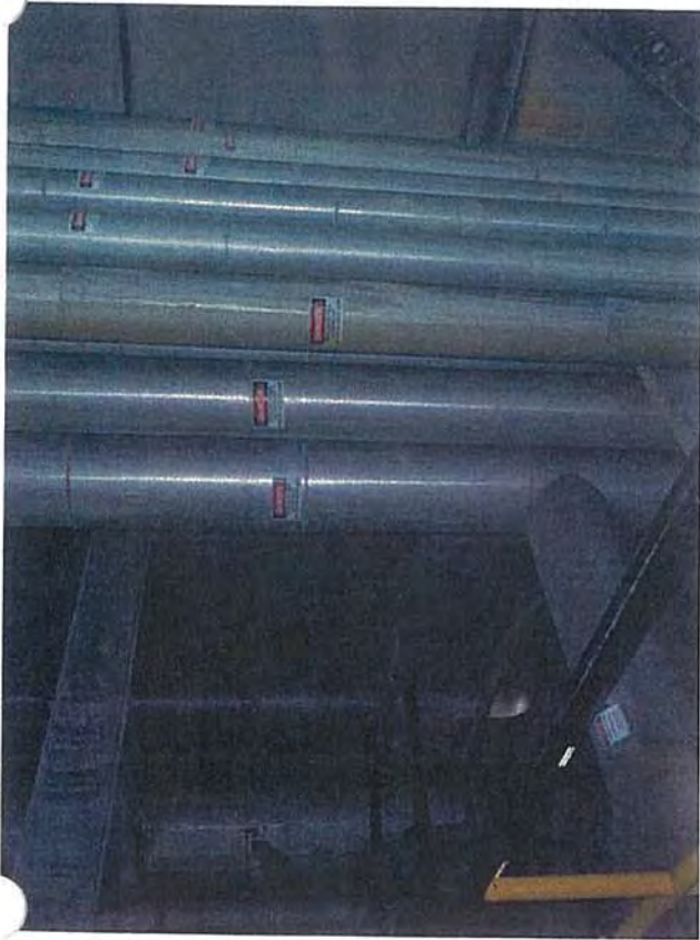
Mezzanine—F2—View of Pipes Along Staircase (Originating from Lower Levels)
