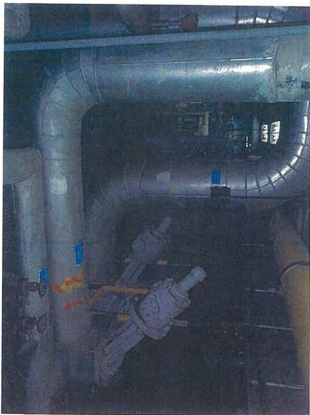
Ground Floor—E2—View of HP Heater/Condenser Pipes
