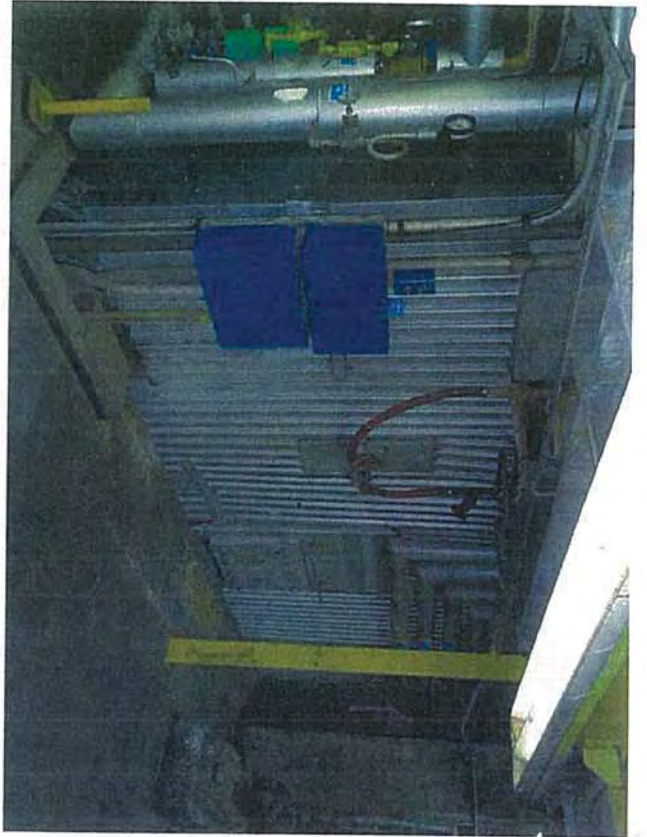
Turbine Deck—B2—View of Boiler and Pipes
