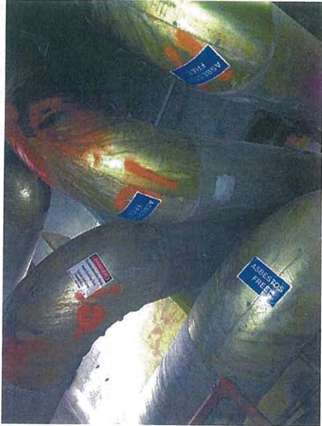
Basement—C2—View of Pipes along Staircase Leading to Upper Levels
