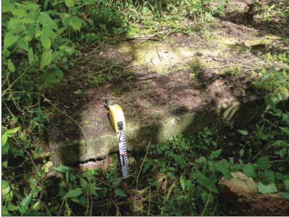
Figure 24. TS-1 Feature 2 concrete foundation (facing northwest).
