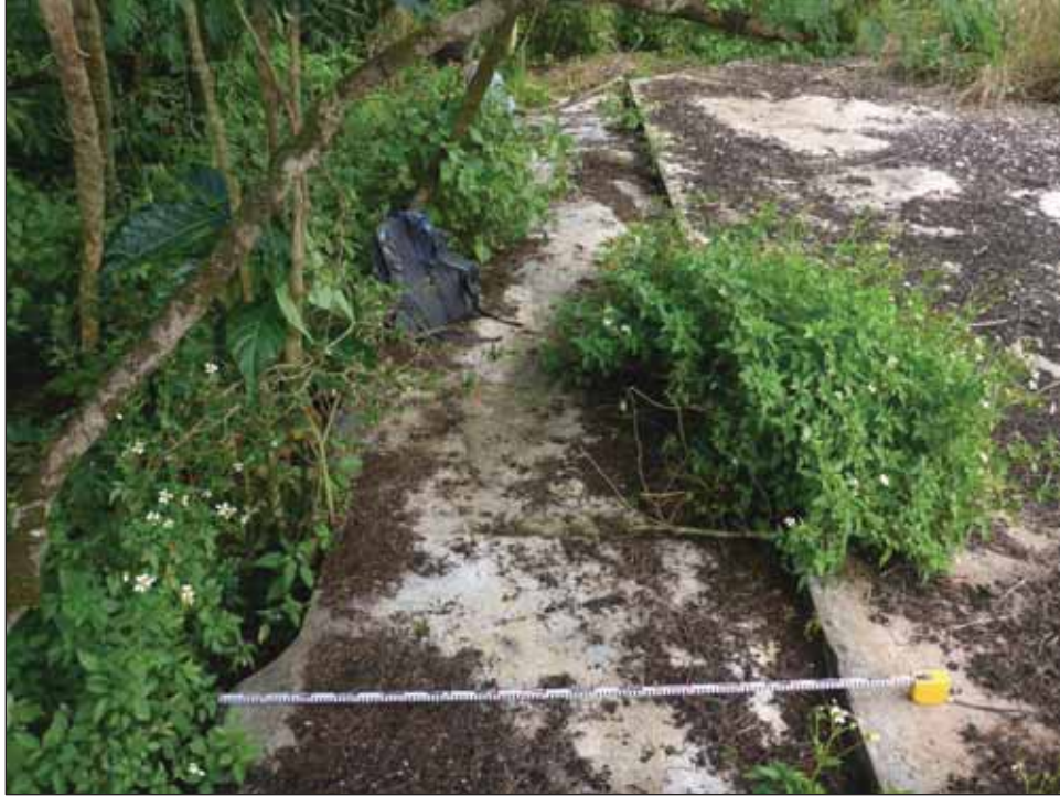
Figure 30. TS-1 Feature 4 lower step along slab's north-facing axis (facing east).
