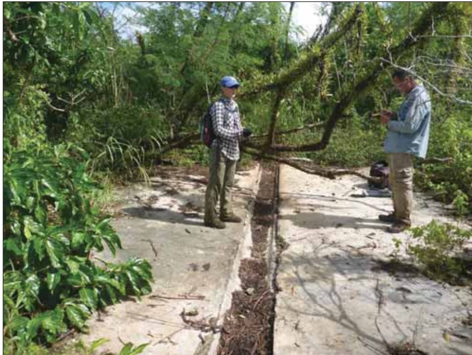
Figure 26. TS-1 Feature 3 overview (facing northeast).
