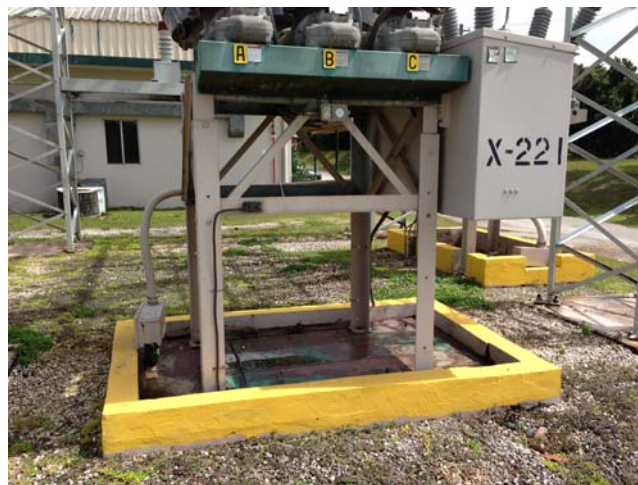
Photo 1 – Berm Floor of X-221 – Concrete – Green, Brown
