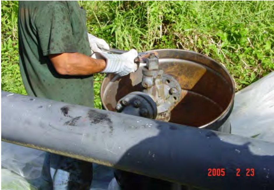
Low Point Drain Valve to be opened to relieve pressure at Spill Point.
