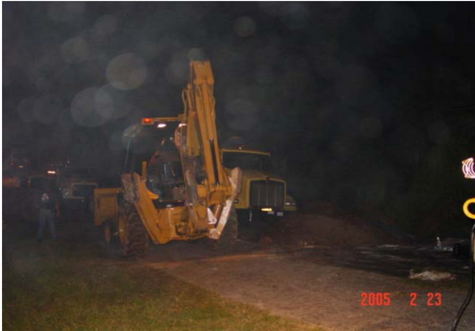
Back hoe utilized in digging and transferring soil to stockpile area on right side.
