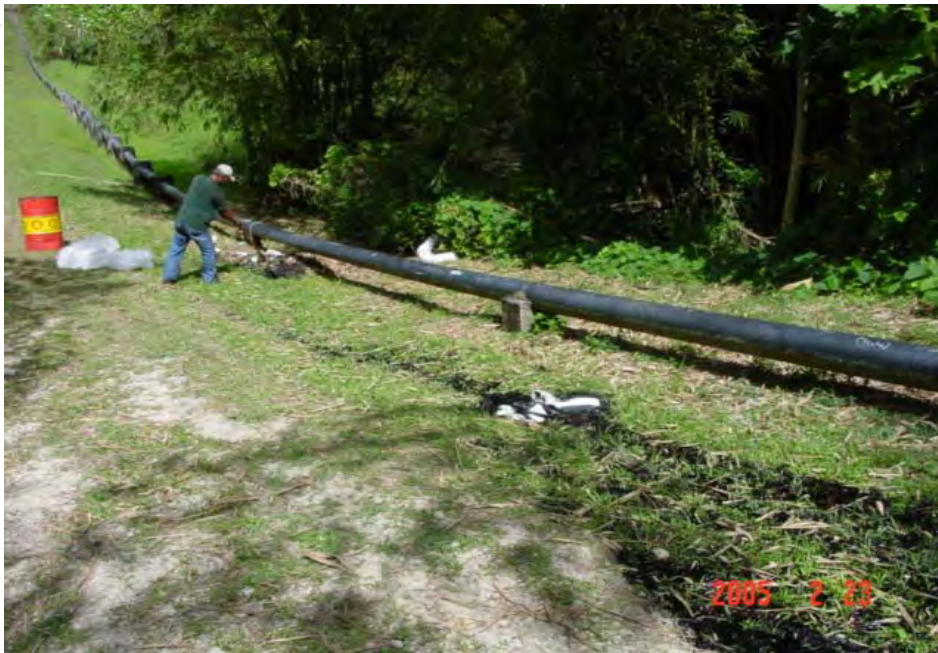
Oil flowing downhill. Greg Quitana on the scene. Booms were placed at the end of the flow about 80 ft downhill from the Spill Point.
