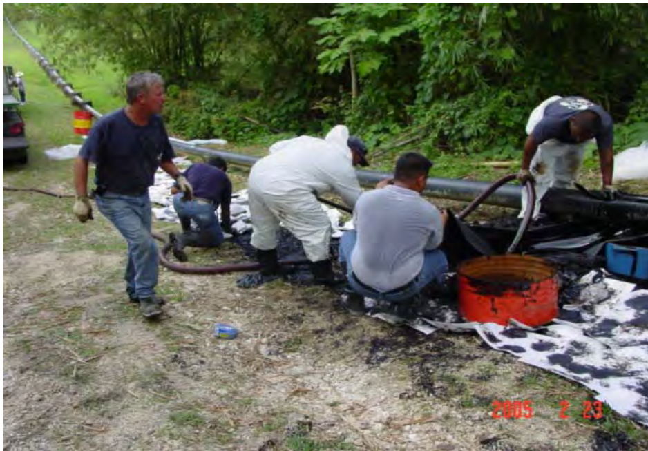
Personnel removing contaminated pads and soil.
