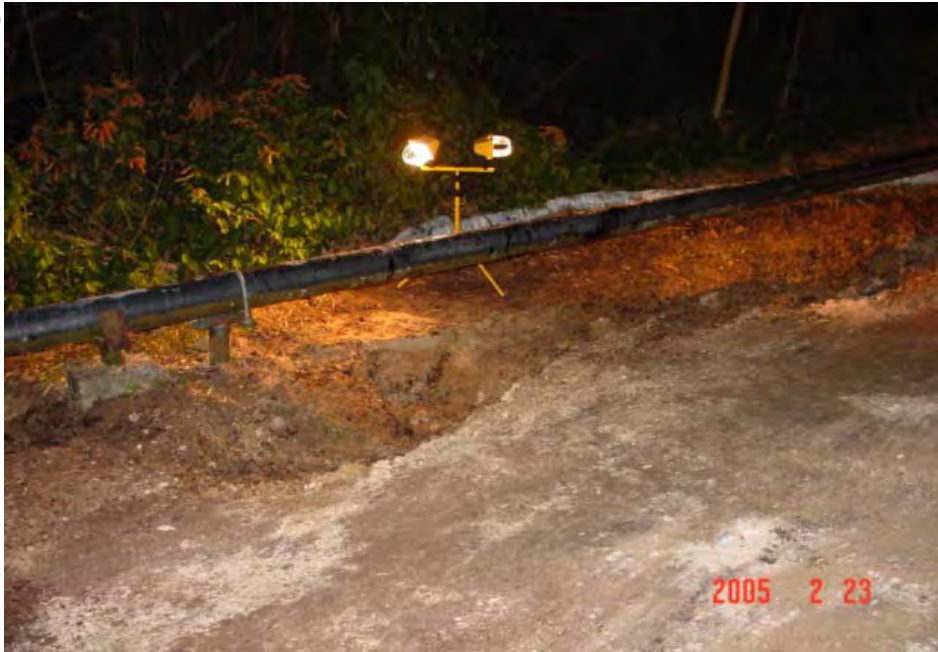
Contaminated soil has been removed.
