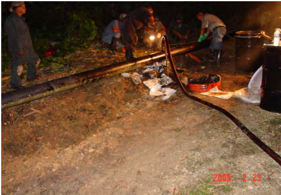
Central Maintenance crews preparing to weld a metal plate around the leak. Contaminated soil has been removed.
