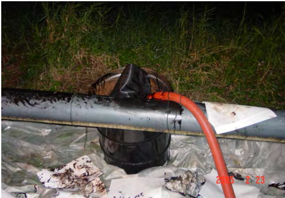
Low Point Drain Valve opened oil being pumped out into Tanker Truck.
