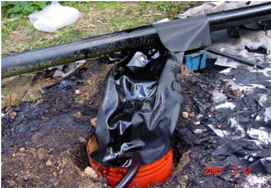
Rubber mat used to direct flow inside a waiting drum. Vacuum truck pumped out oil collected in drum.
