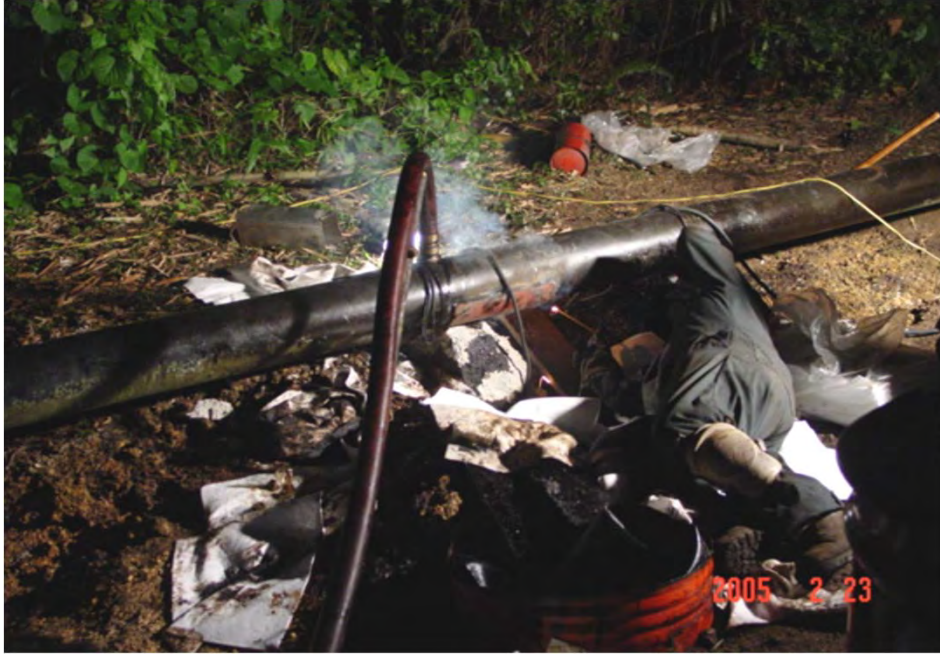
Central Maintenance Crew welding plate over the leak.
