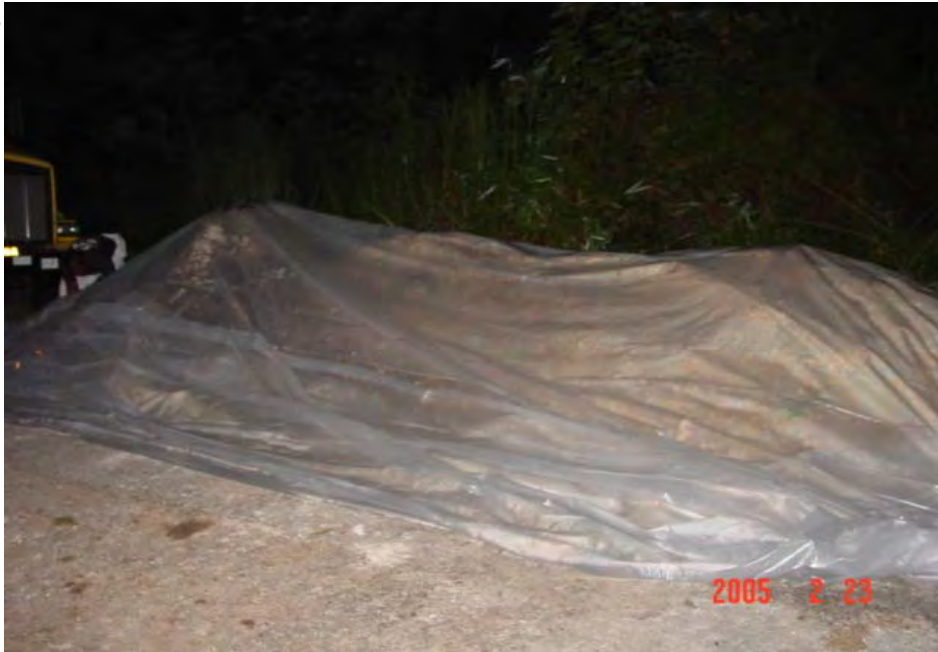
Stockpiled soil covered with plastic sheeting. An estimated 1.5 - 2 dump truck loads of soil was removed.
