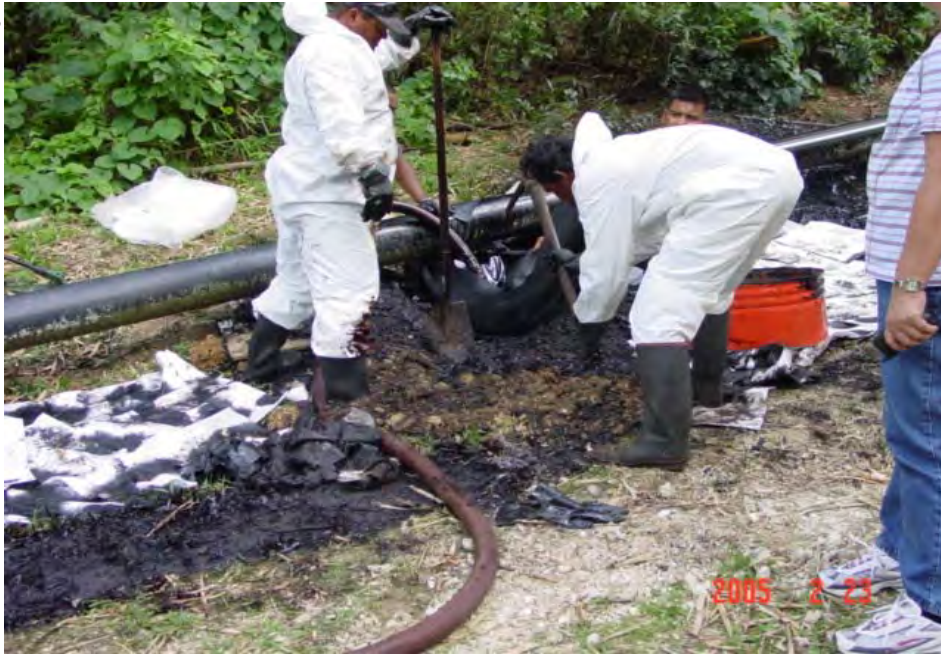
Personnel removing contaminated pads and soil.
