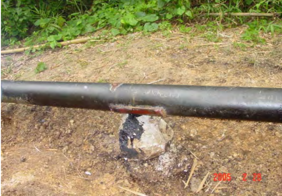
Leak has been repaired
