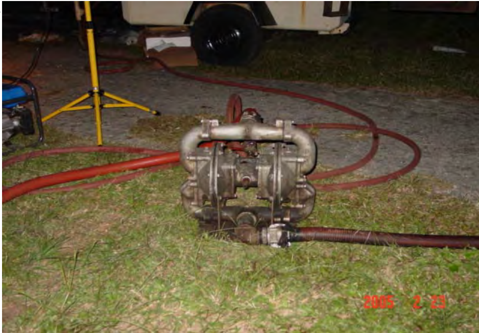
Diaphragm pump transferring oil from Low Point Drain Valve to Tanker Truck.
