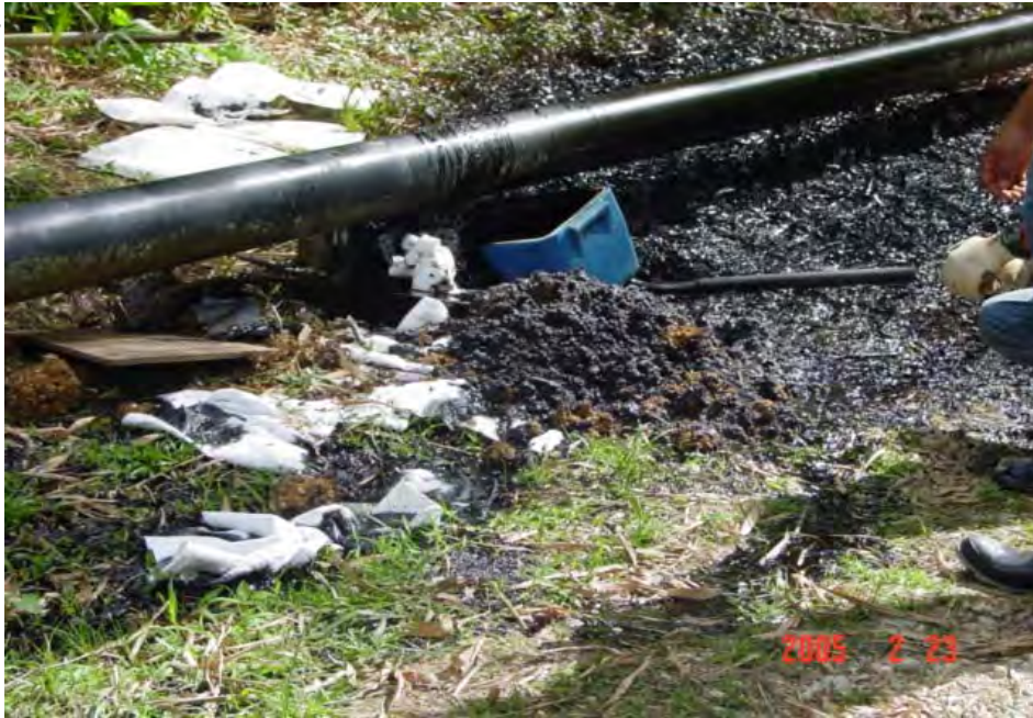
Spill Point. Defect located at the saddle area.
