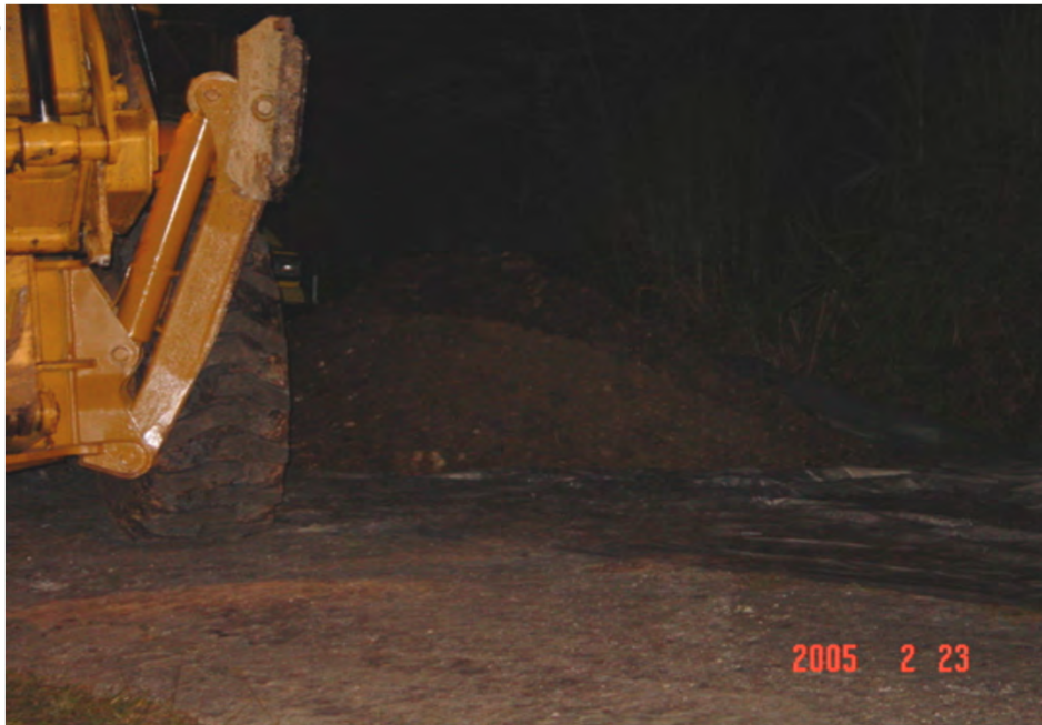
Close-up of stockpiled soil. Plastic sheeting was laid on the ground prior to soil transfers.
