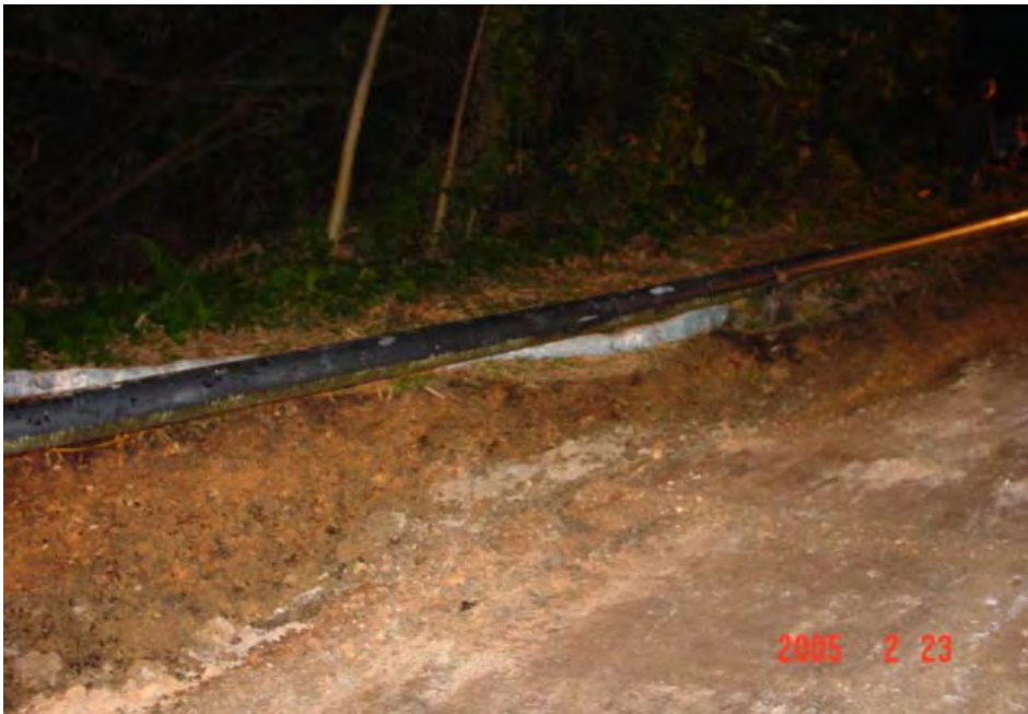
Contaminated soil has been removed.
