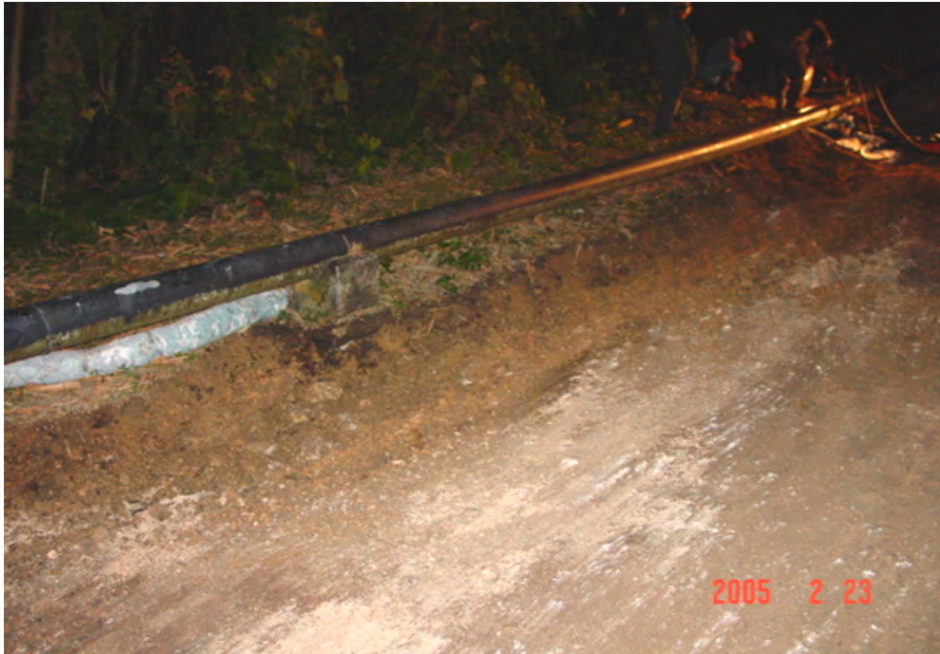
Contaminated soil has been removed.
