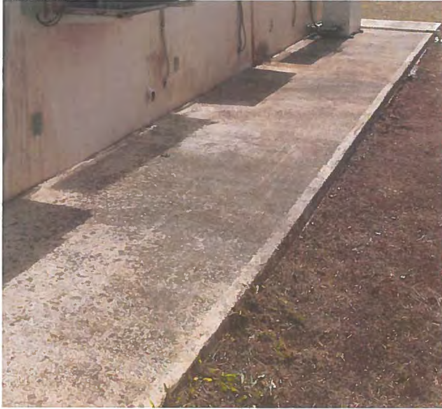
Photo 5 of 8 February 24 2015 Photo taken at the northern concrete sidewalk after the cleanup
