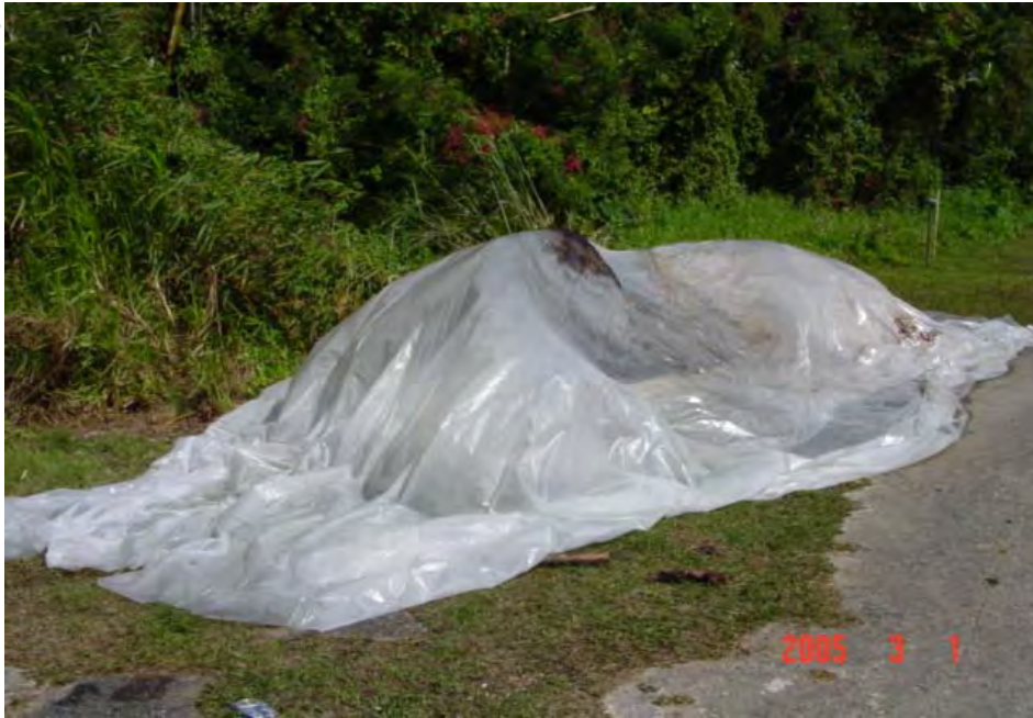
Stockpiled contaminated soil.
