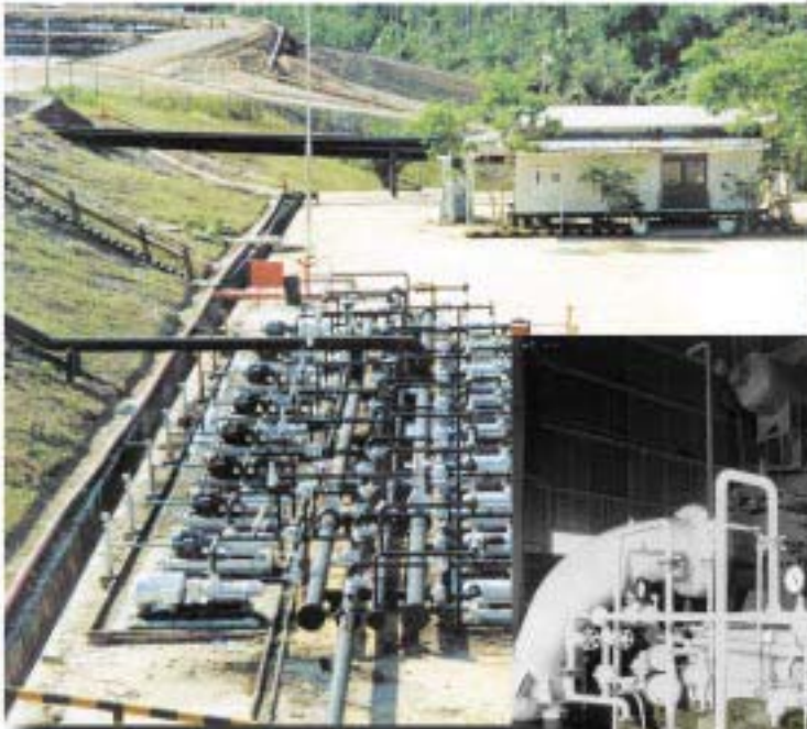
(16) 6D-312 pumps on crude oil pipeline service in the Pacific Rim area
