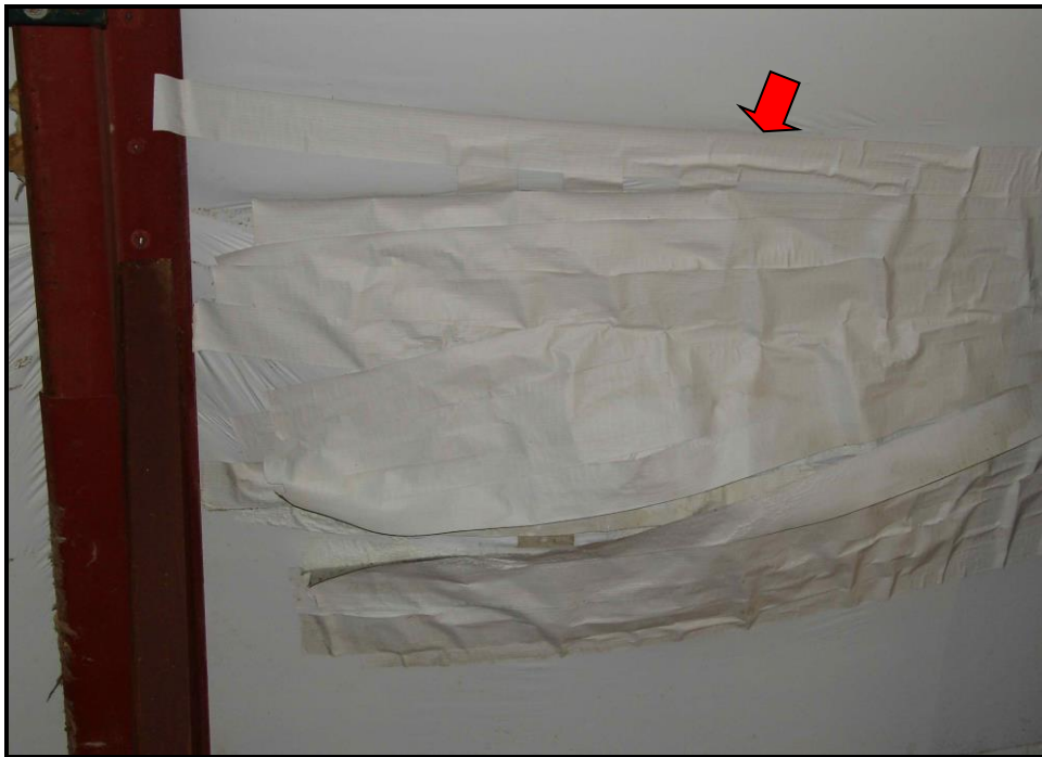
Roof leakage resulting to damage of roof insulation
