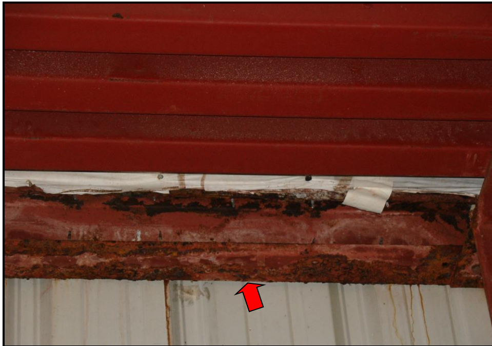
Evidence of corrosion on sidewall girts supporting the wall cladding and roof due to water intrusion
