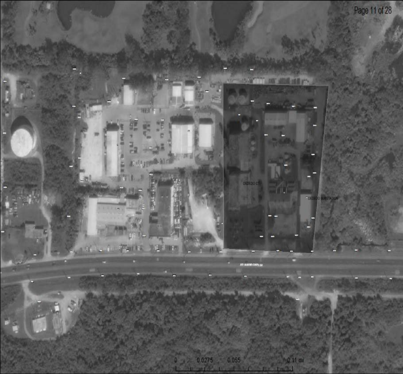
Attachment C Combustion Turbine Compound Dededo
