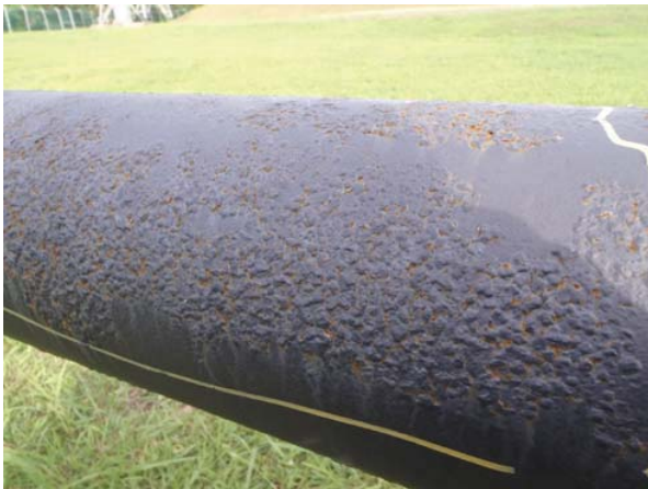
Closed view of corrosion
