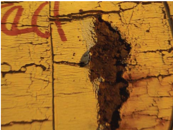
Closed view of corrosion
