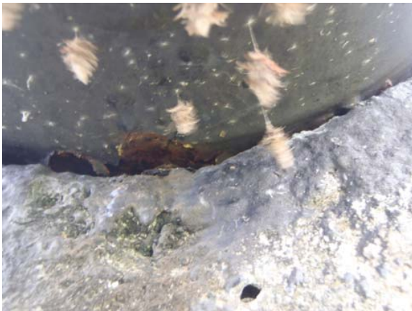
Closed view of corrosion
