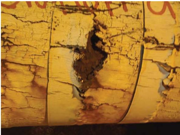
Closed view of corrosion
