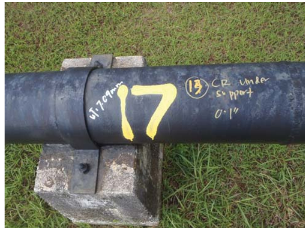
Corrosion under pipe support
