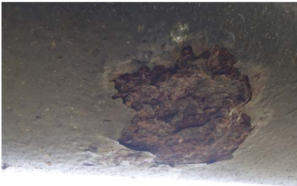
Closed view of corrosion
