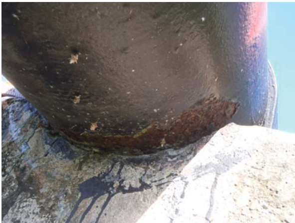
Closed view of corrosion
