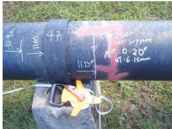
Corrosion under pipe support
