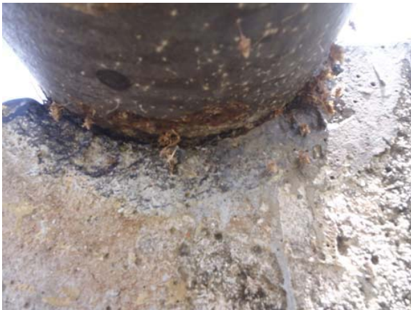
Close view of corrosion
