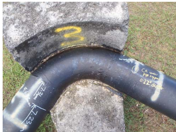
Corrosion under pipe support
