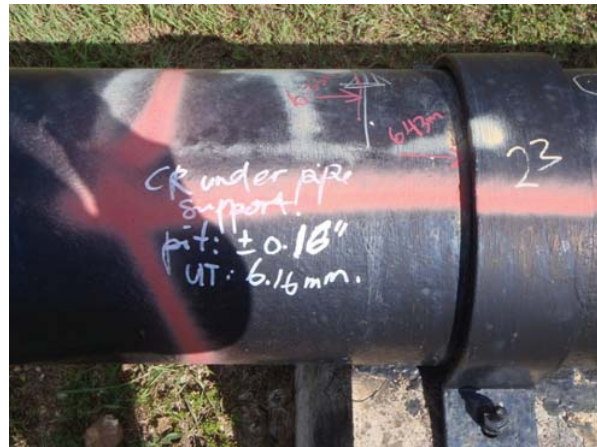
Corrosion on pipe support
