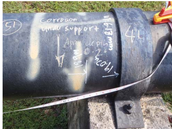
Corrosion under pipe support
