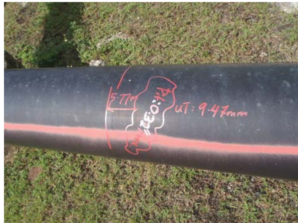
Severe corrosion localized at 6H00
