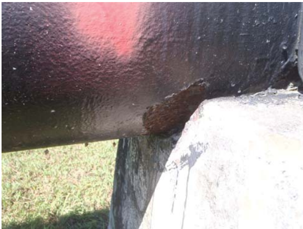
Closed view of corrosion
