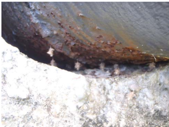
Closed view of corrosion
