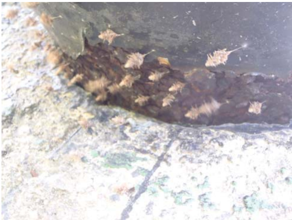
Closed view of corrosion
