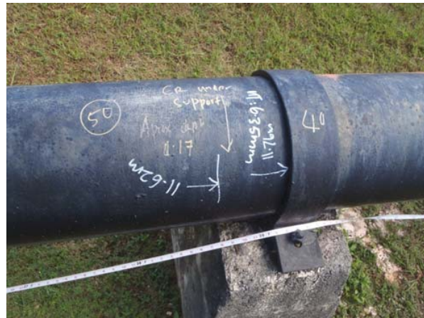
Corrosion under pipe support
