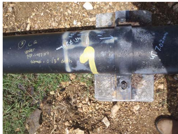
Corrosion under pipe support
