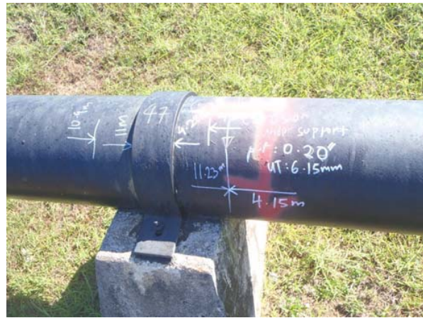
Corrosion under pipe support
