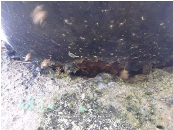
Closed view of corrosion
