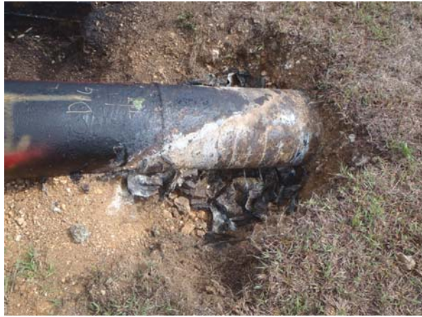
View of soil to air interface
