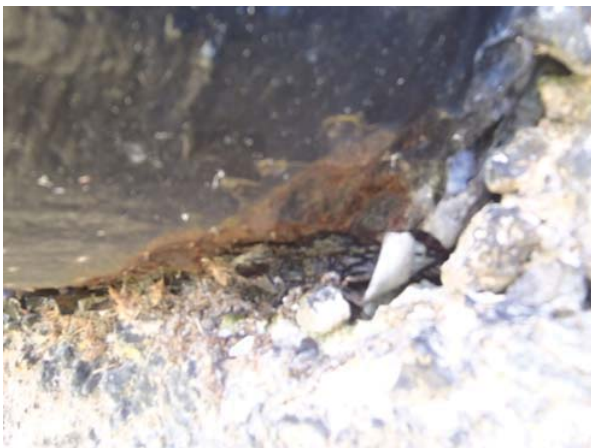
Closed view of corrosion
