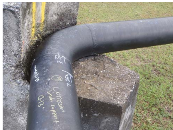
Corrosion under pipe support
