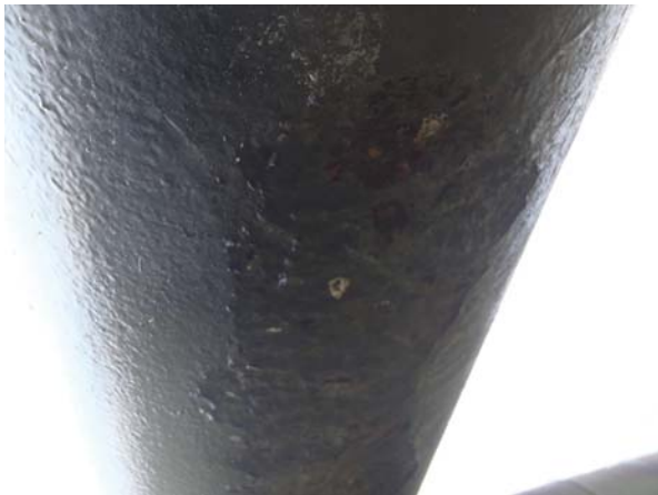
Closed view of corrosion
