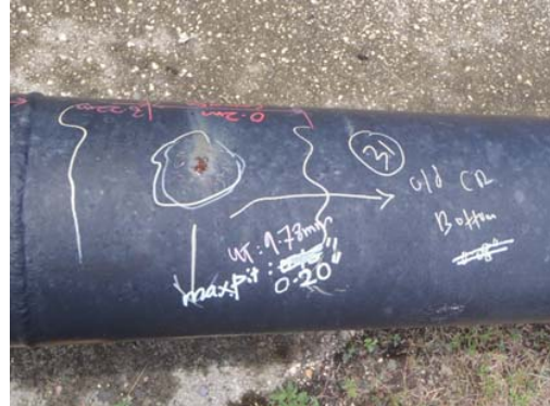
Localize corrosion at 6H00
