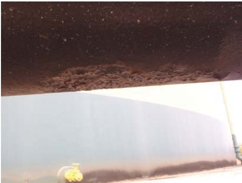
Closed view of corrosion
