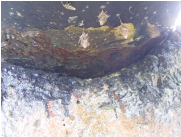
Closed view of corrosion under pipe support
