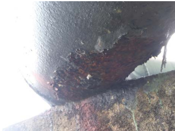
Closed view of corrosion
