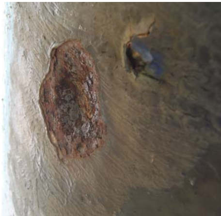
Closed view of corrosion
