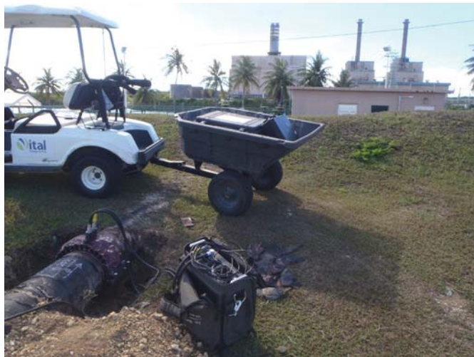
Positive direction towards pump area
