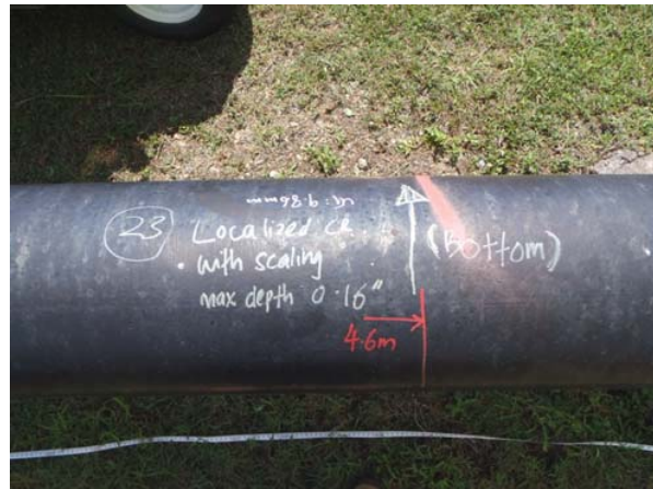
Localized corrosion at 6H00
