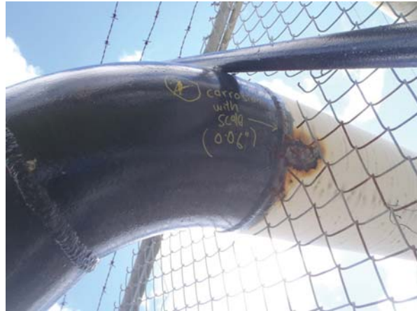
External corrosion at 6 o'clock
