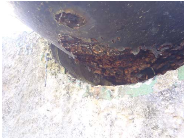
Closed view corrosion under pipe support
