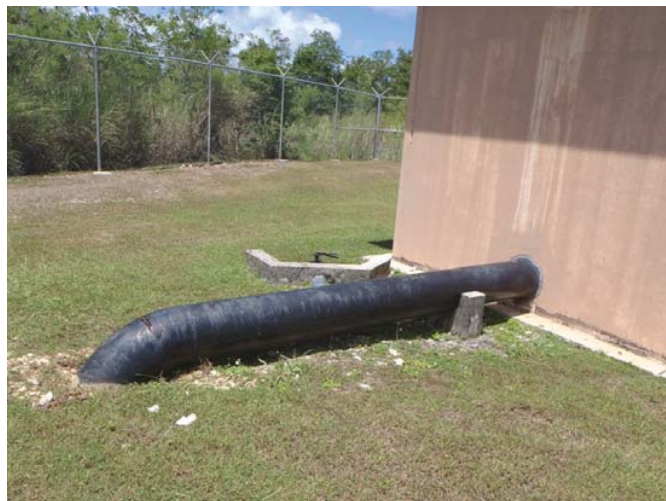
General view of pipeline
