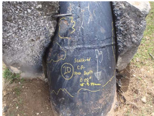
Scattered corrosion with maximum pit depth is 0.08" @ 2.0 mm
