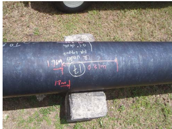
Corrosion under pipe support
