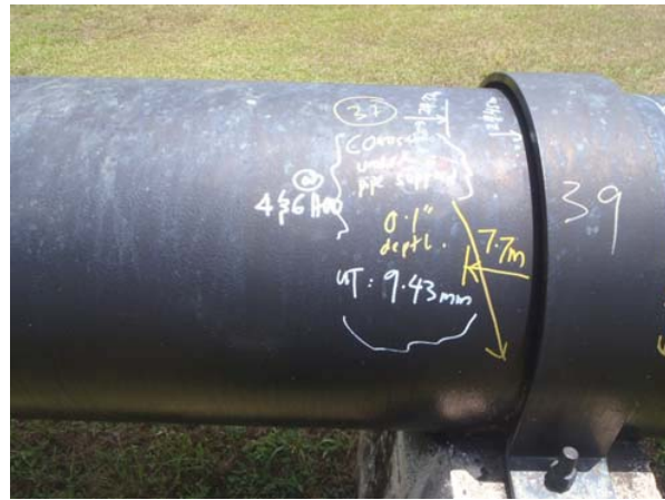
Corrosion closed to the pipe support
