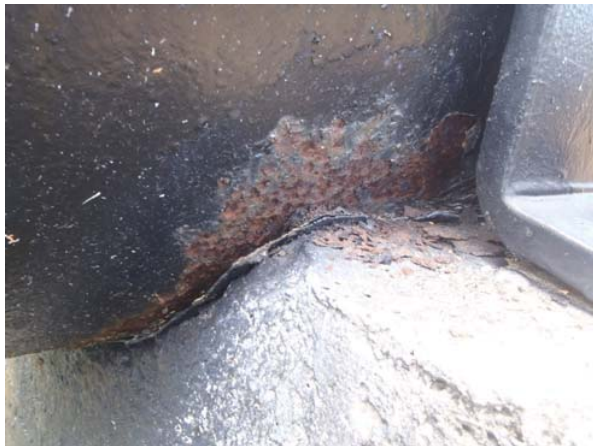
closed view of the corrosion
