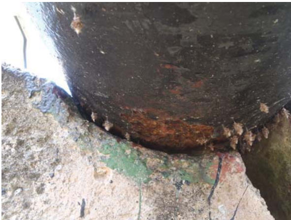
Closed view of corrosion
