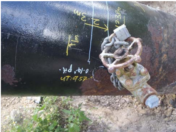
External corrosion with max. pitting is 0.14" @ 3.5 mm
