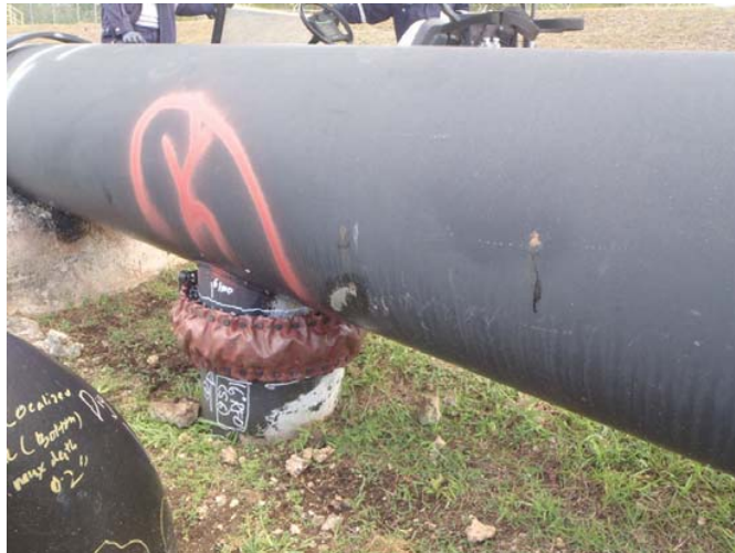
General view of pipeline
