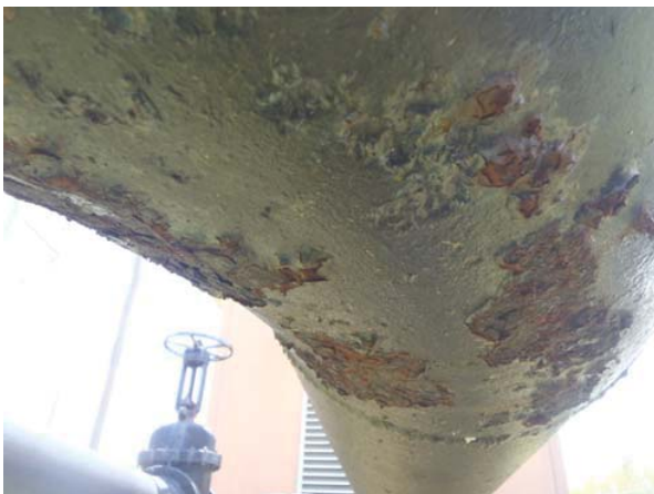
View of external corrosion with max. depth is 0.27" @ 6.8 mm
