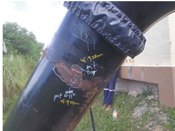
External corrosion with max. pitting is 0.11" @ 2.8 mm
