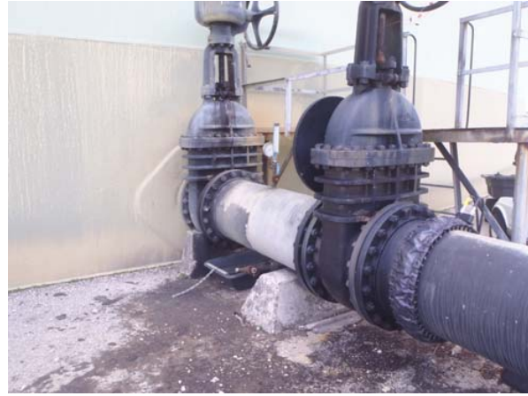
General view of external corrosion
