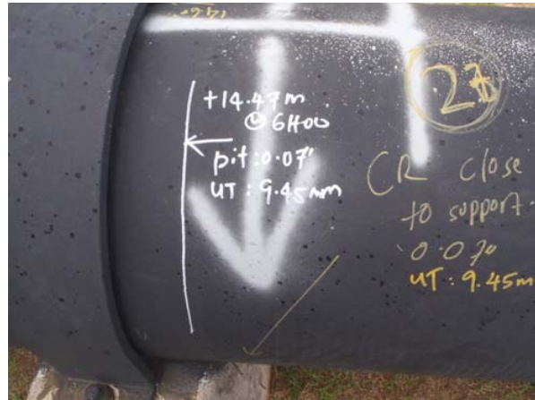
External corrosion near to pipe support
