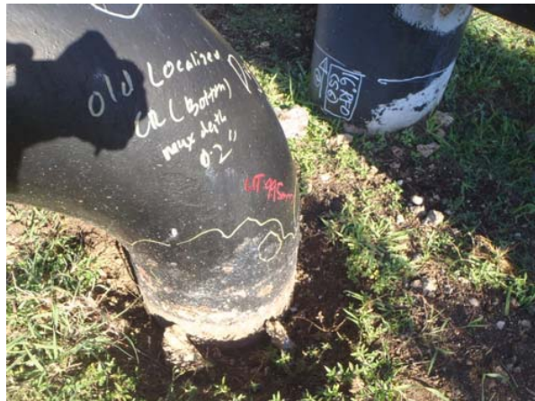
Corrosion at soil to air interface
