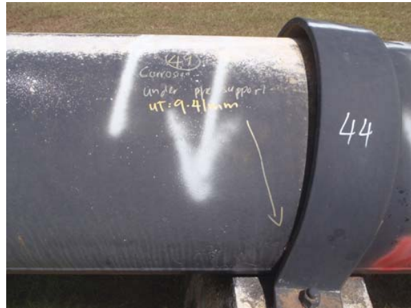
Corrosion under pipe support
