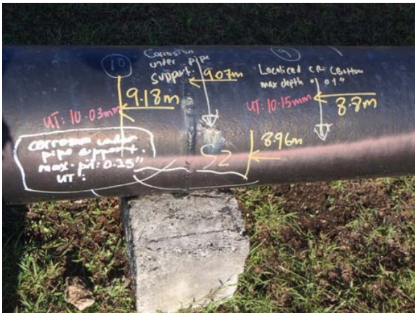
Corrosion under pipe support
