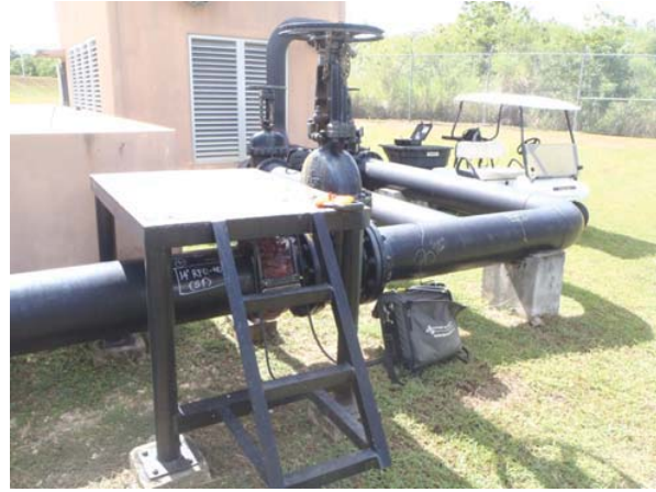
General view of pipeline
