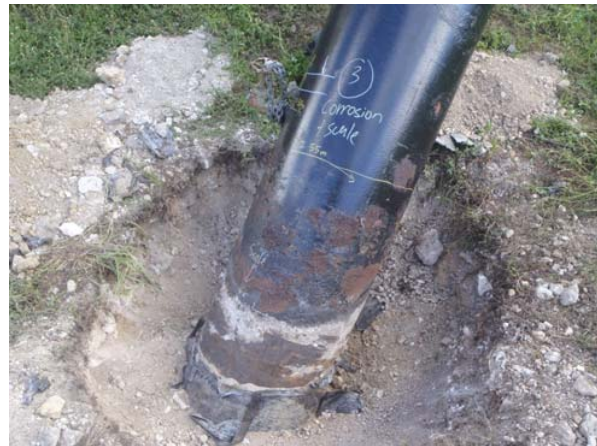
General view of external corrosion at soil to air interface
