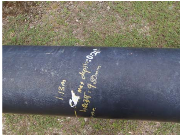
External corrosion at 6H00 with max. pit depth is 0.21" @ 5.3 mm.
