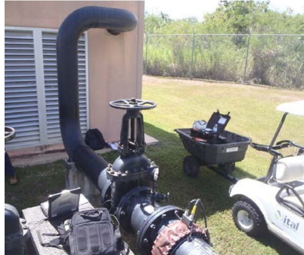
General view of pipeline
