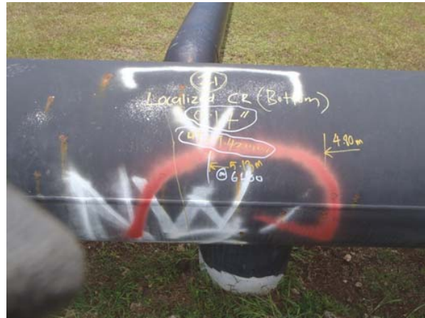
Localized external corrosion at 6H00. Max. pit depth: 0.17" @ 4.3 mm
