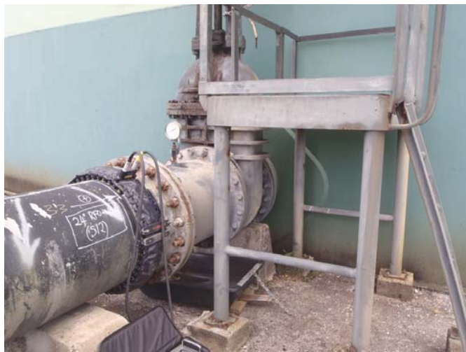
General view of positive direction - to tank 1934
