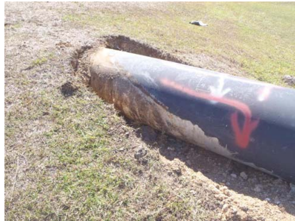
Corrosion at soil to air interface on wrapping section
