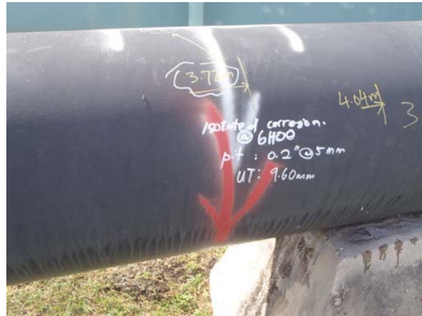
Isolated external corrosion at 6H00 near the pipe support
