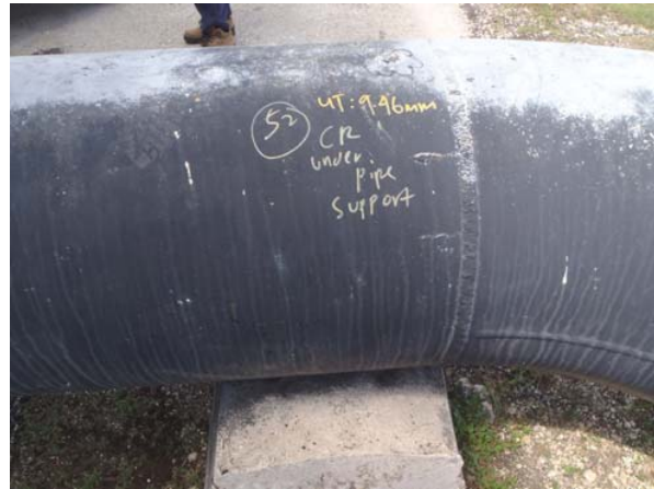
corrosion under pipe support
