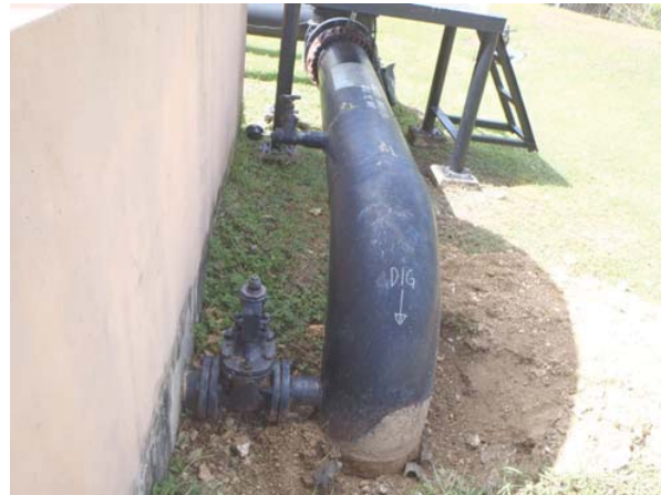
General view of pipeline
