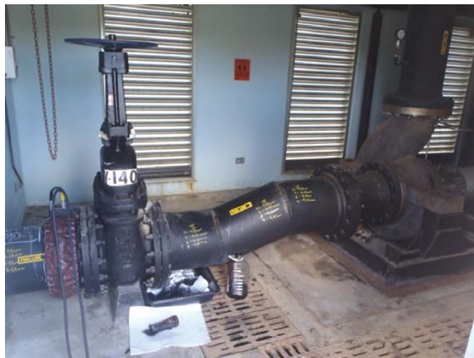
General view of pipeline
