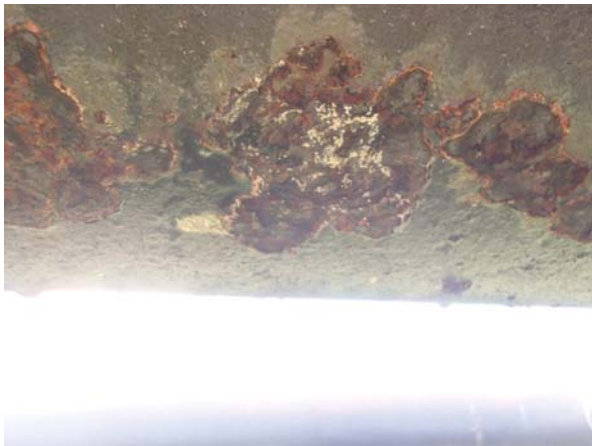
Closed view of corrosion
